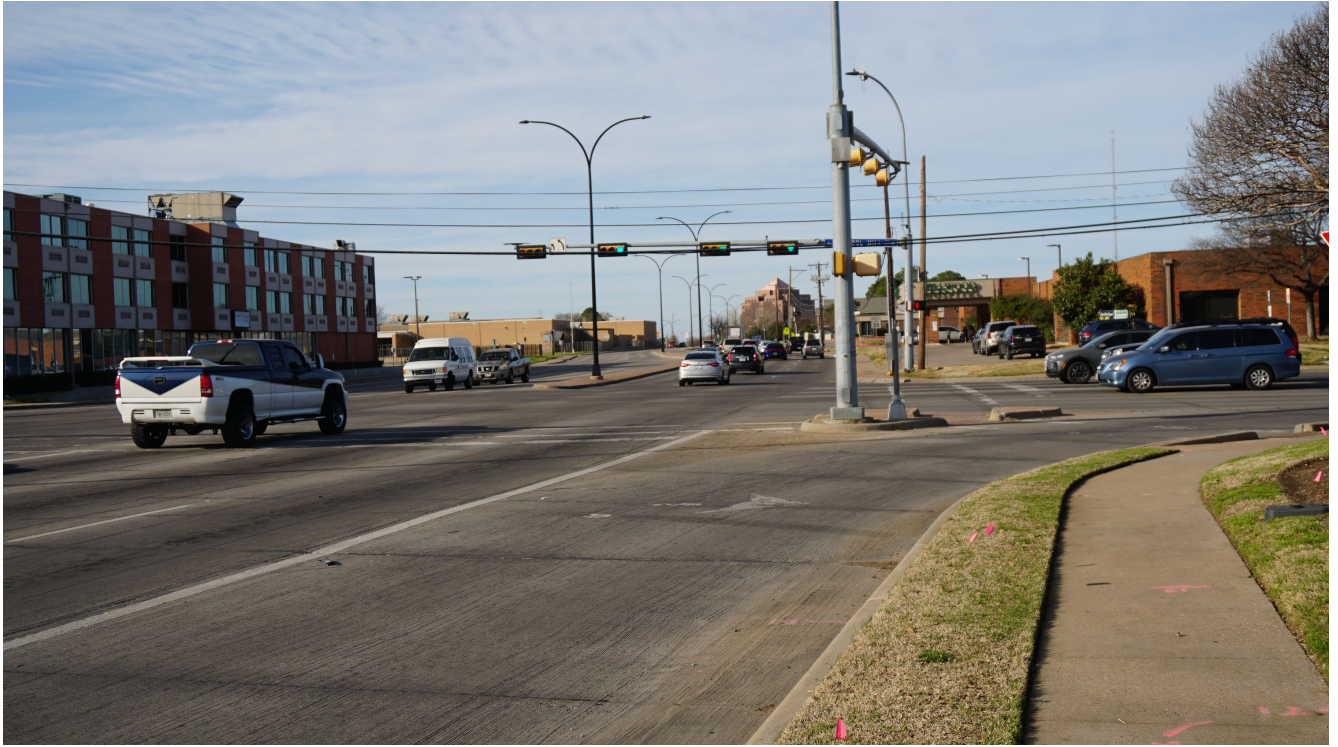
Figure 6: Design of right-turn islands like this one (southeast corner of Center Street and Randol Mill Road) allow for high-speed turns with reduced yielding to pedestrians
