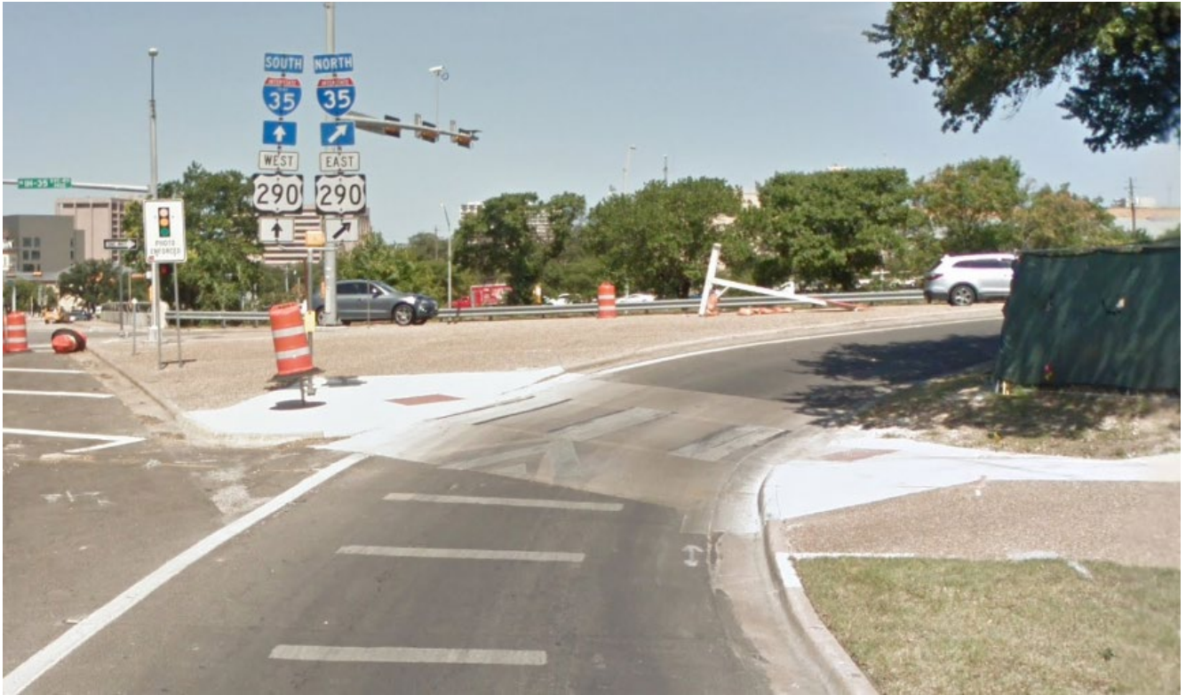
Figure 8: Example of a raised crosswalk on a turn lane joining an Interstate frontage road in Austin, TX (Source: Google Street View )
