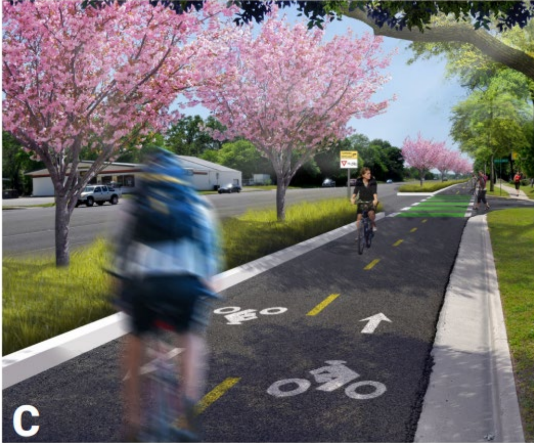
Figure 14: Example of separated bike lane option recommended with 5-6 lane roadway section (Source: Active Tyler: Active transportation Plan for the Tyler, TX Area MPO)
