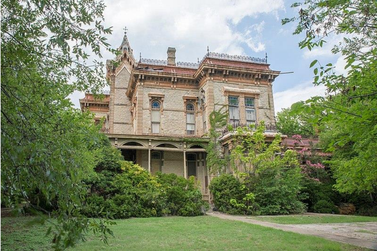
Figure 53: Waggoner Mansion (added 1974 - - #74002098): 1003 E. Main, Decatur. Picture by Renelibrary, CC BY-SA 4.0 , via Wikimedia Commons
