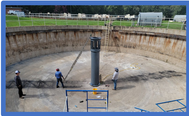
City of Huntsville August 2024 Clarifier Rehabilitation
