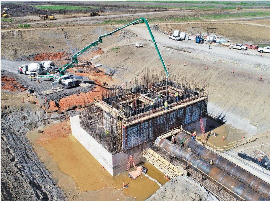
Pouring walls for the Intake Structure
