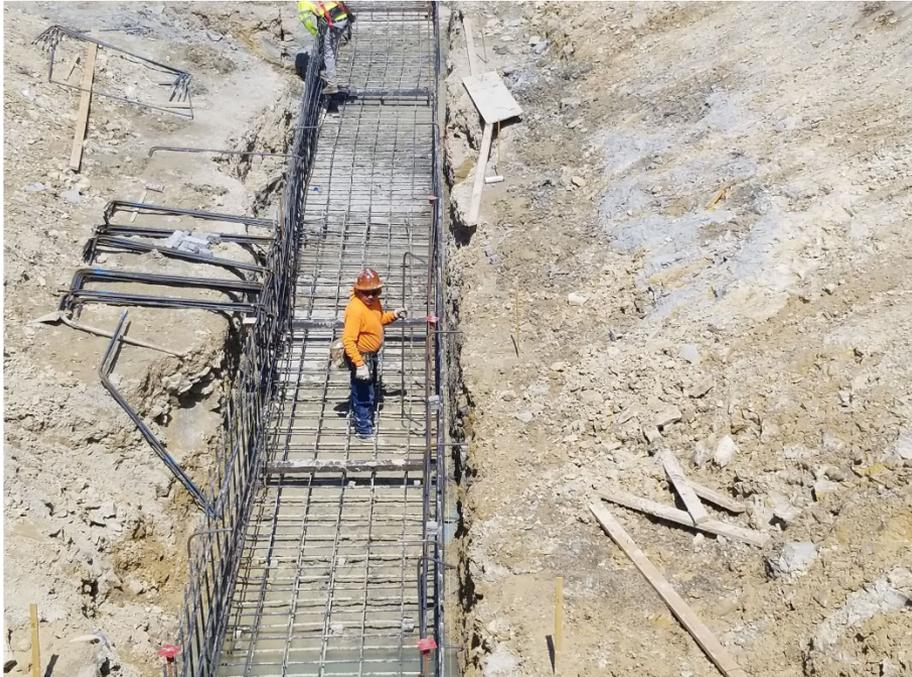
Working on reinforcing steel for pipe encasement for Chlorine Contact Basin
