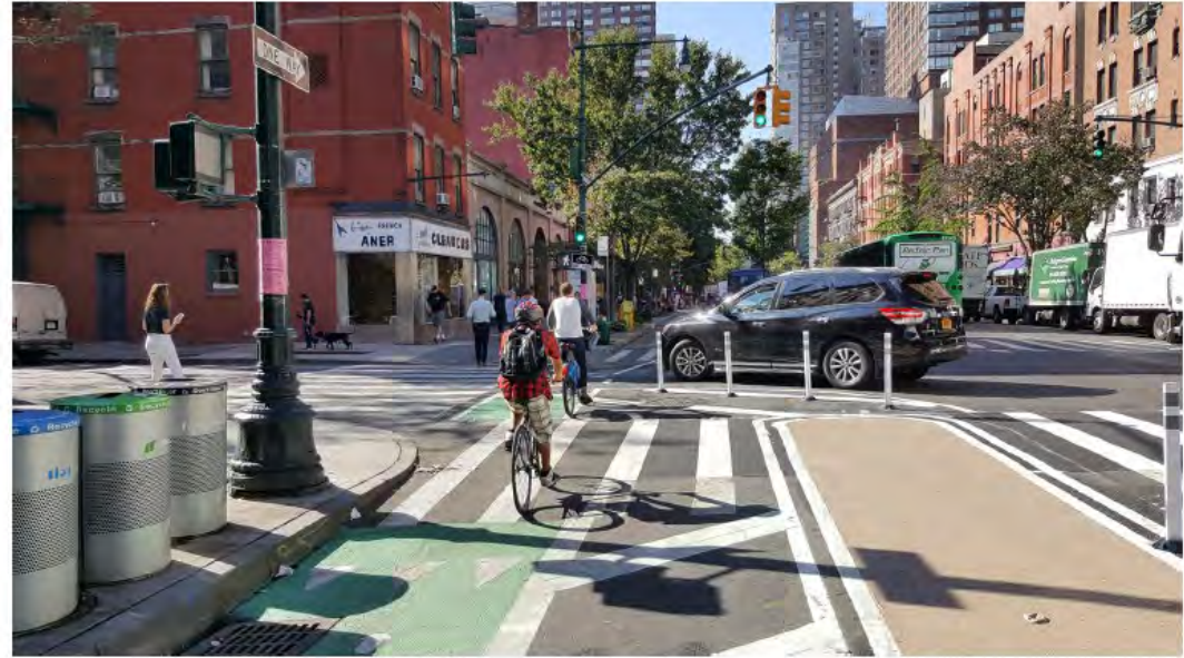
Figure 7-15: Corner Island with Flexible Delineator Posts (Source: Carl Sundstrom, PE, Office of Bicycle and Pedestrian Programs, New York City Department of Transportation)
