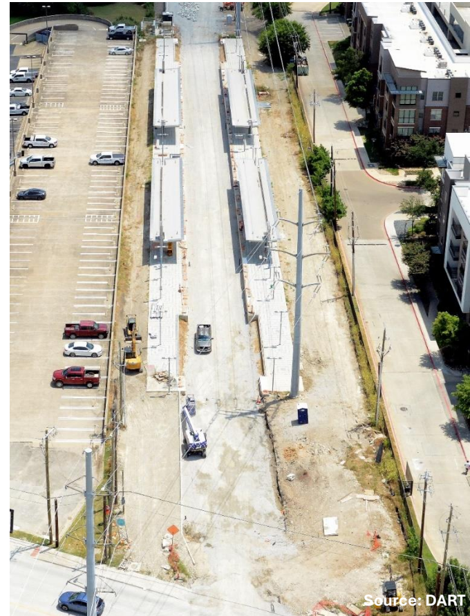
Silver Line Rail at Knoll Trail Station under construction
