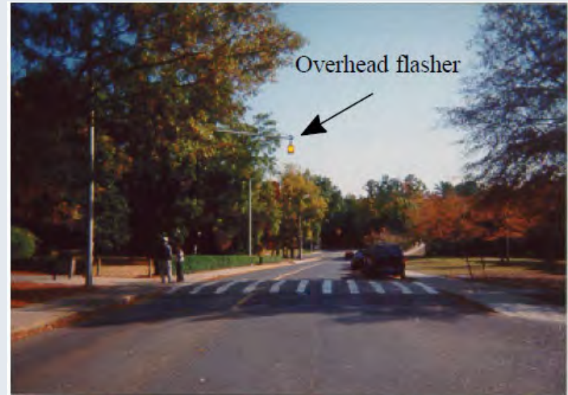
Figure 6. Raised crosswalk and overhead flasher, Towerview Drive, Durham, North Carolina.
