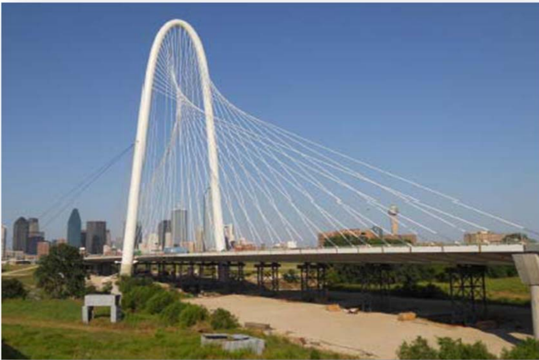
Margaret Hunt Hill Bridge in Dallas Source: NCTCOG photo archives
