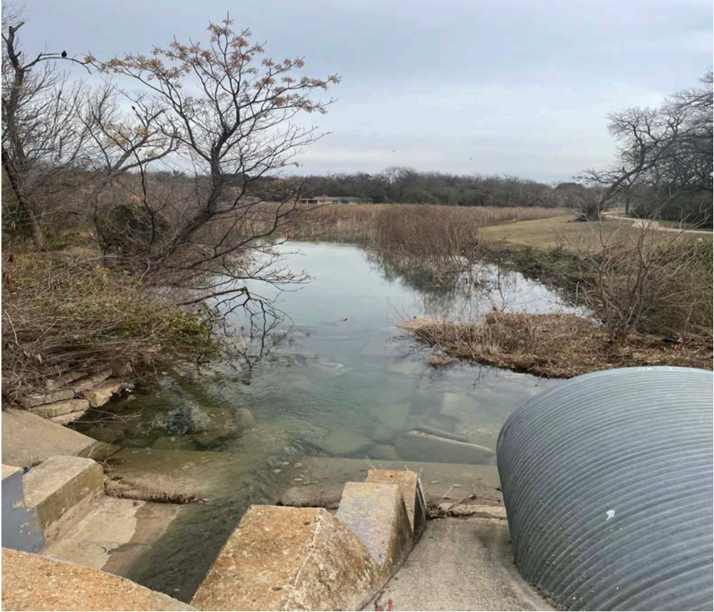
Site 4, Primary Outfall to Lake Como, Northwest Side
