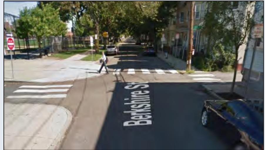
Curb Extension at Berkshire St & York St
