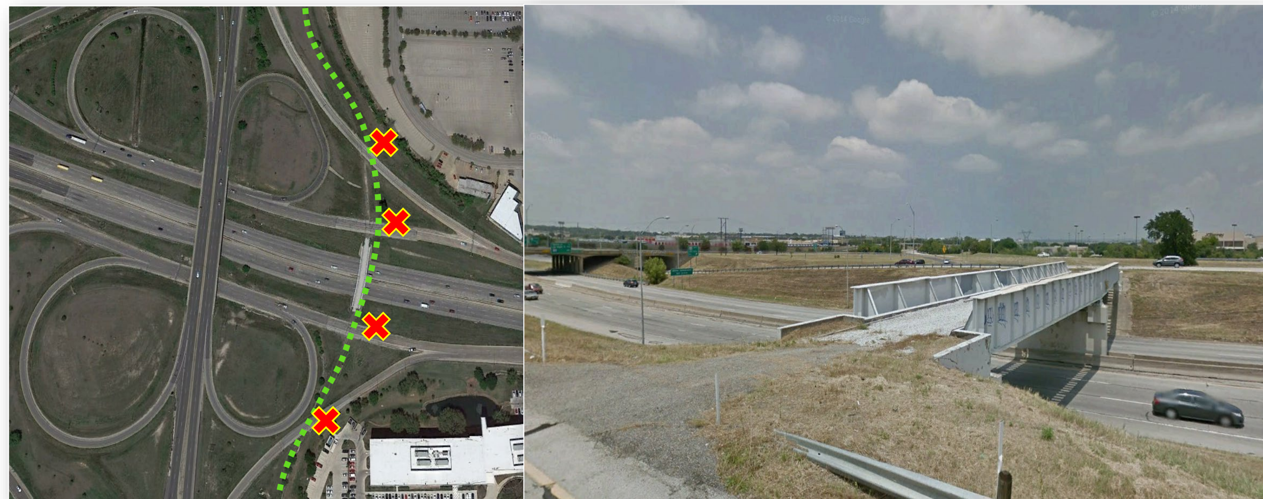
Existing Rail Bridge view north at Interstate 30
