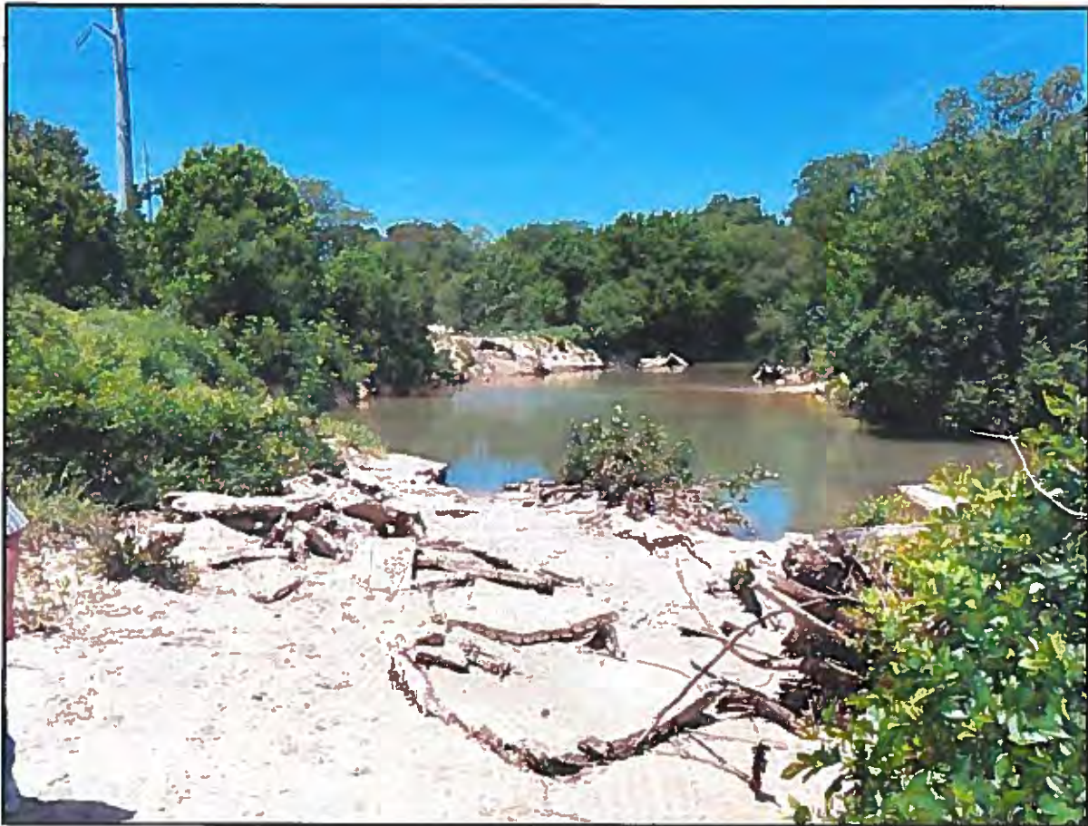
Figure 3-2: Rowlett Creek Downstream of the Atchison Topeka and Santa Fe Railroad Bridge on May 10, 2018.
