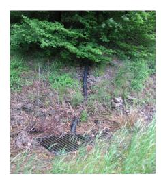
A surface hose discharging into a storm drain inlet. This may be an illicit connection. (photo courtesy WSDOT)
