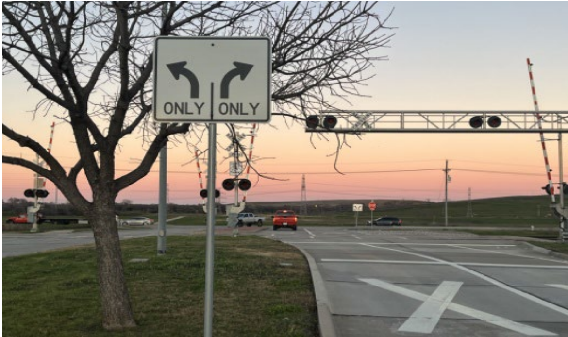
Corporate Drive ends at a 3-way stop at Railroad Street in Lewisville. Two construction projects are underway to extend the road to Old Denton Road. (Cody Thorn/Community Impact)
