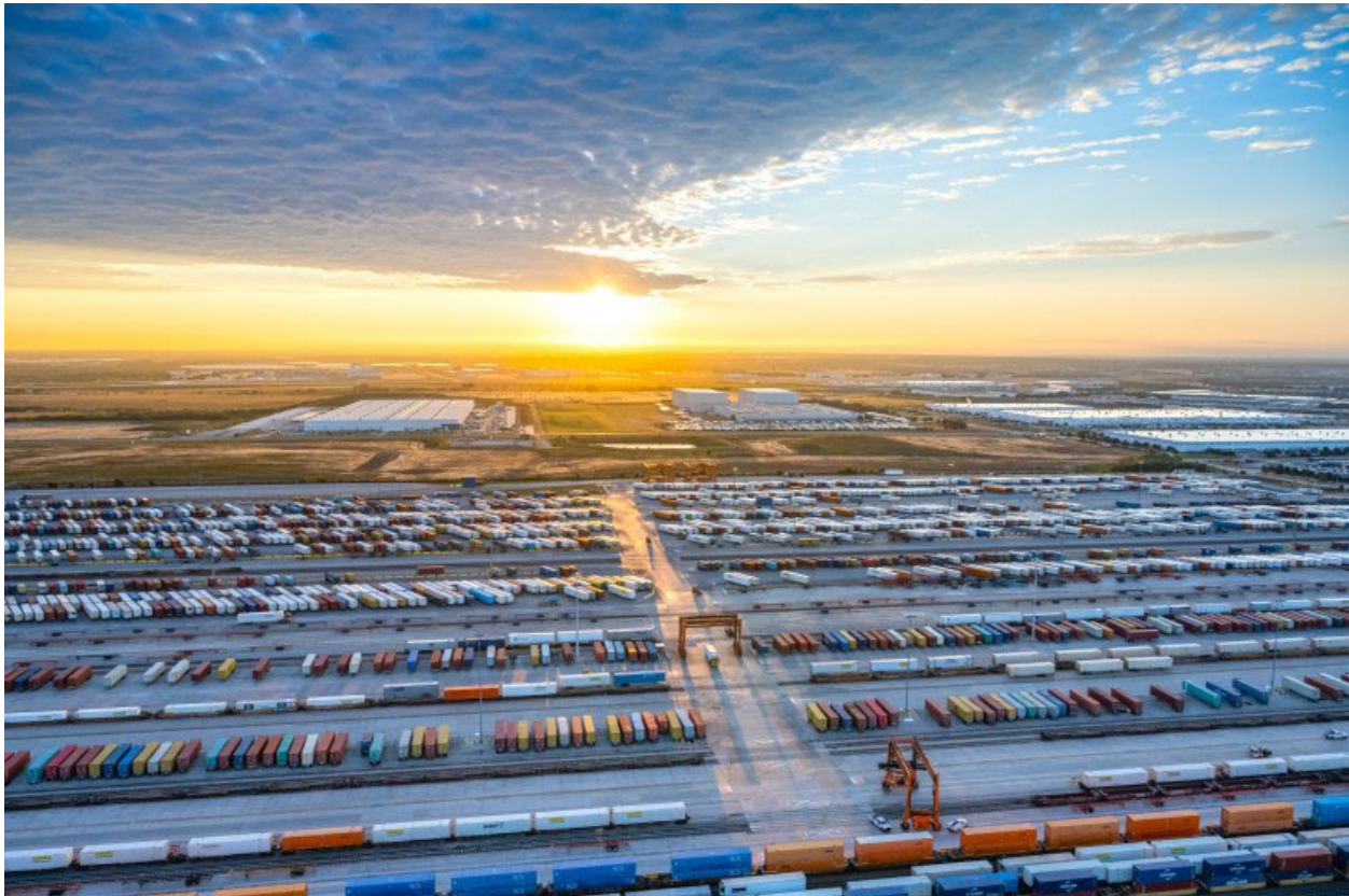
The BNSF Intermodal facility at Alliance Texas. (Courtesy photo | Hillwood) Credit: Debra Hale
