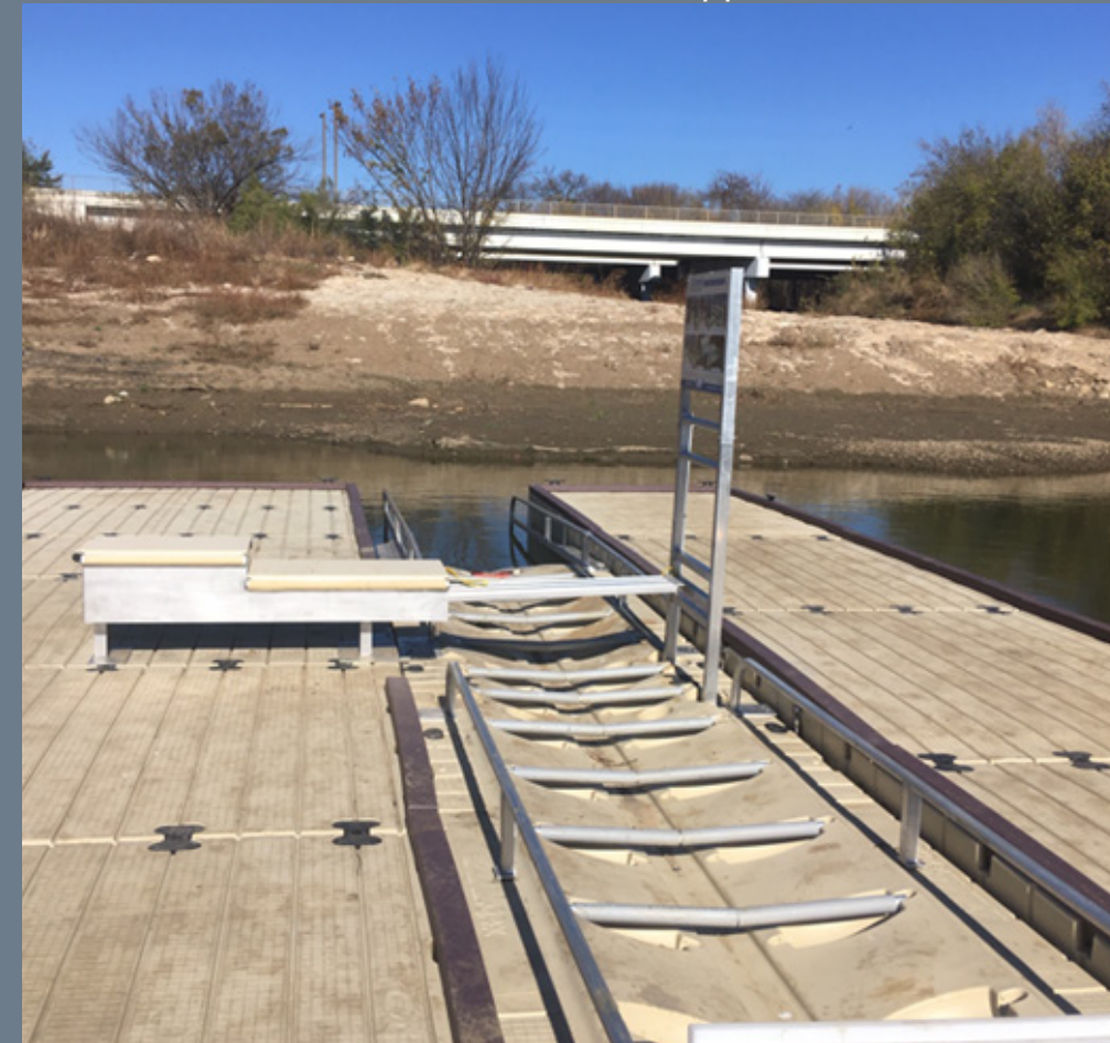
Figure 3.1: “Roll-on/roll-off” floating dock with ADA seat and slide seat support.
