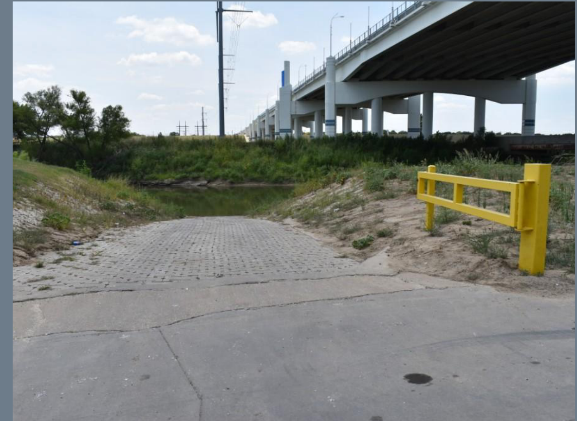
Figure 4.9: The launch site at Trammel Crow Park.
