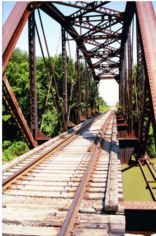
MP 741.1 - Trinity River Bridge
