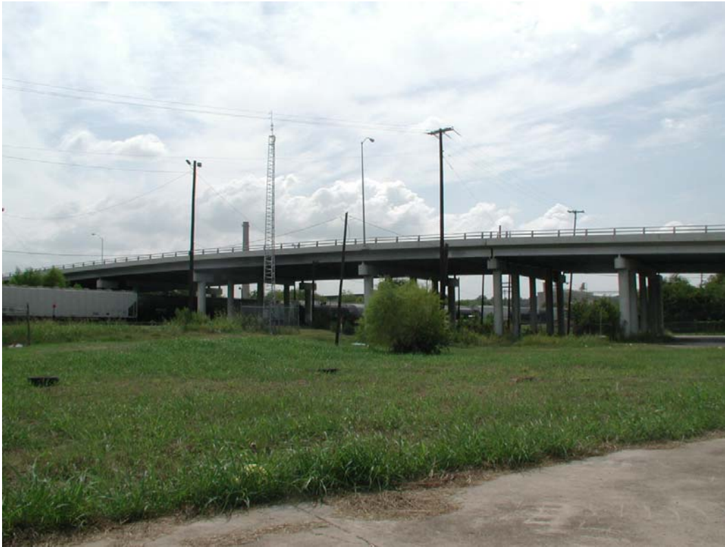
Looking South at Hampton Rd. Overpass
