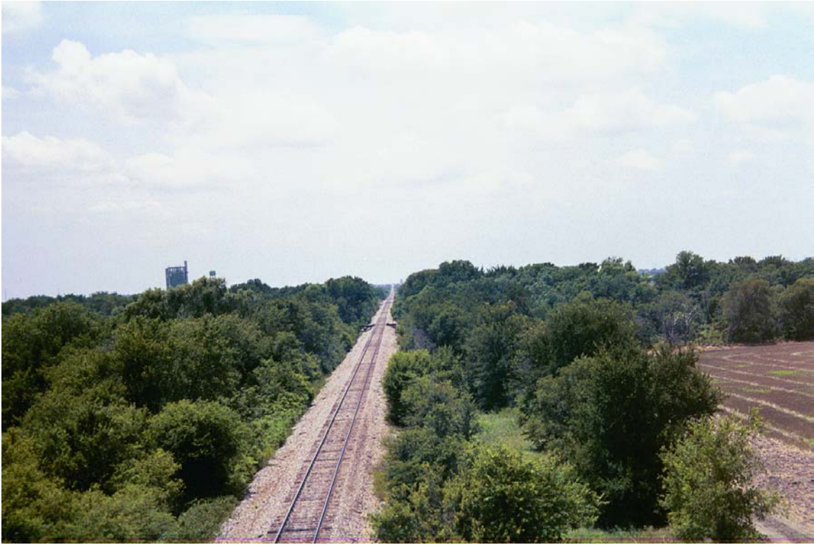
BNSF Frisco Line Looking South US 380 overpass
