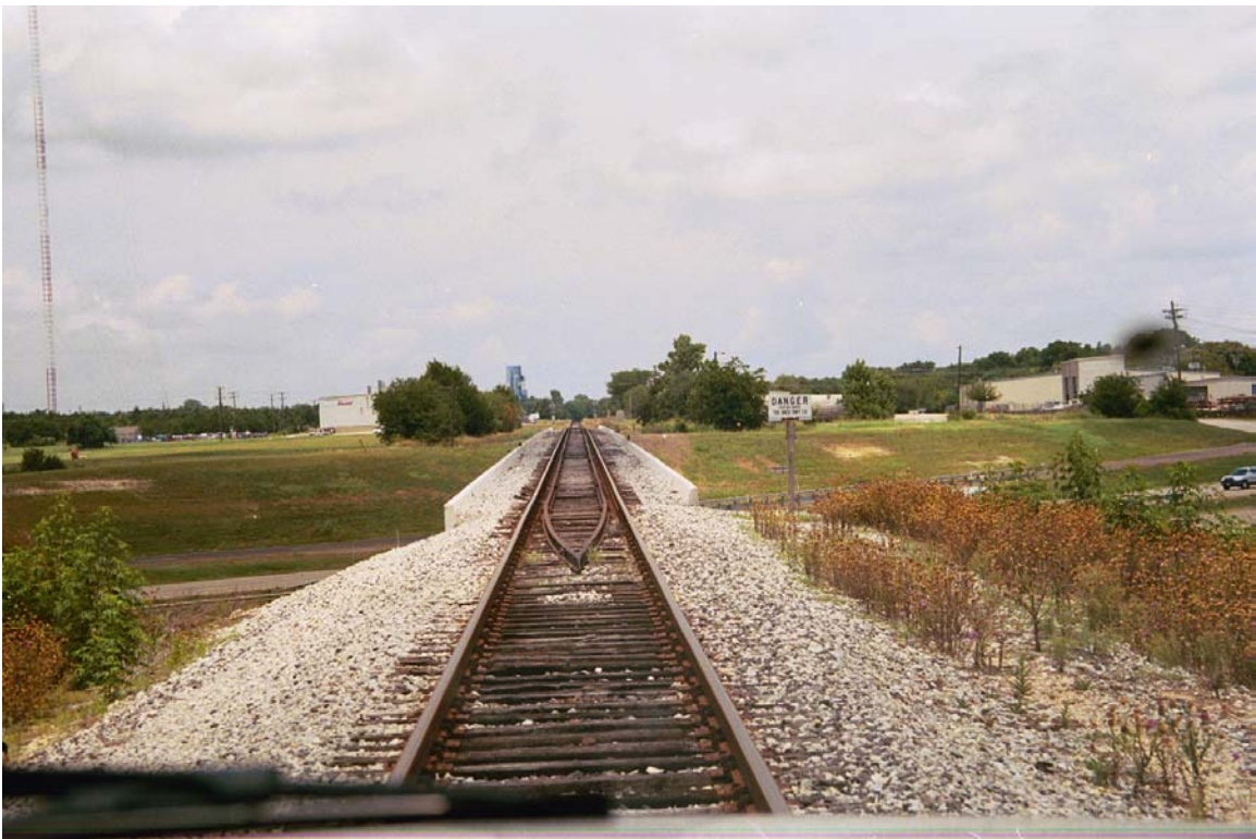
MP 33.7 Bridge over US HWY 67
