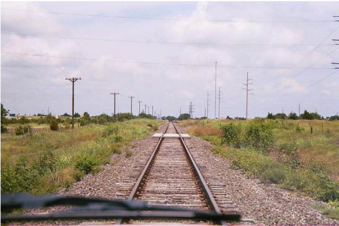
MP 28.6 Private crossing not complete
