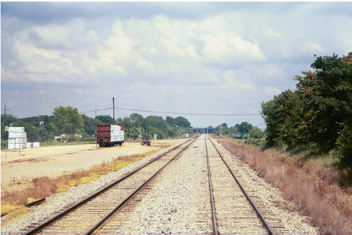
MP 621.7 Hurst Siding and Norwood Dr crossing Looking East
