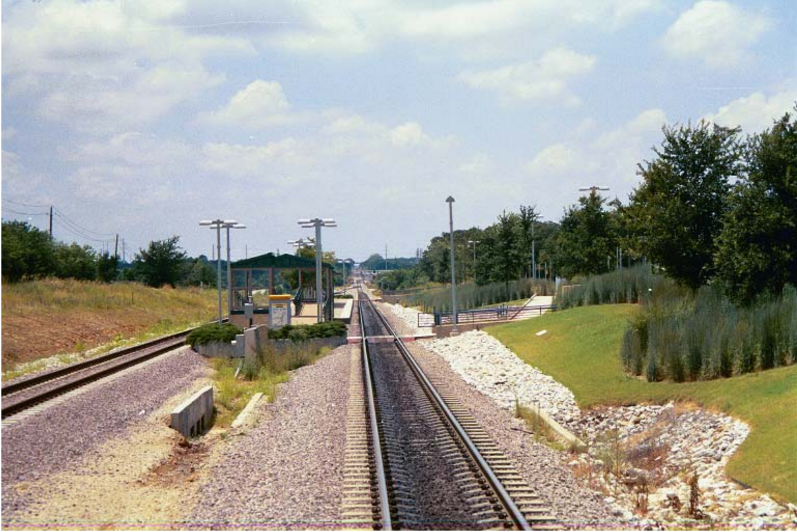
MP 631.4 West Irving Station
