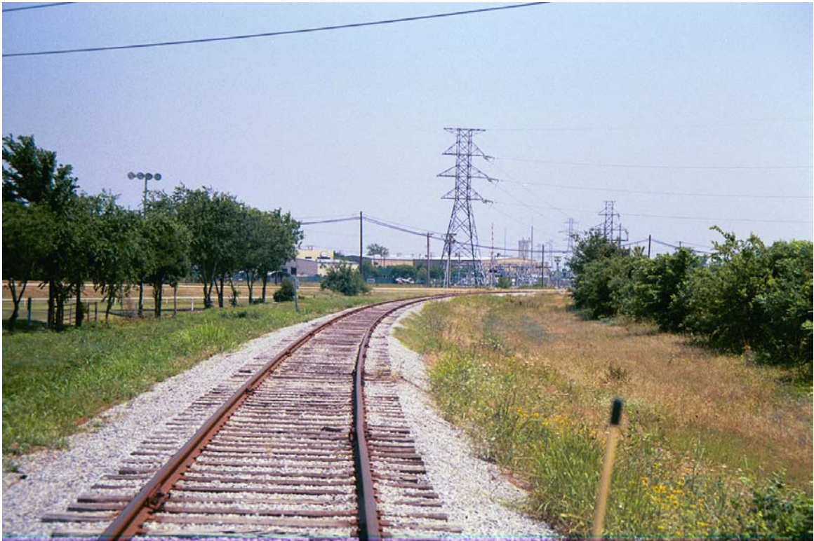
MP 735.0 – Approaching Mill Street
