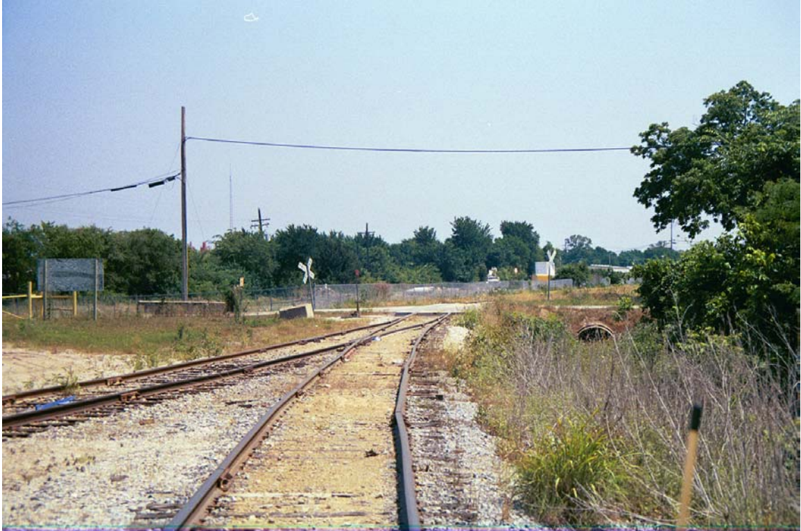
MP 736.5 – South end of ISG siding with College Street in distance. Note kink in rail at right
