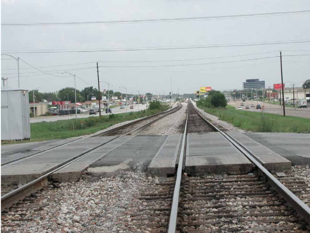
Looking East at 23 rd St.
