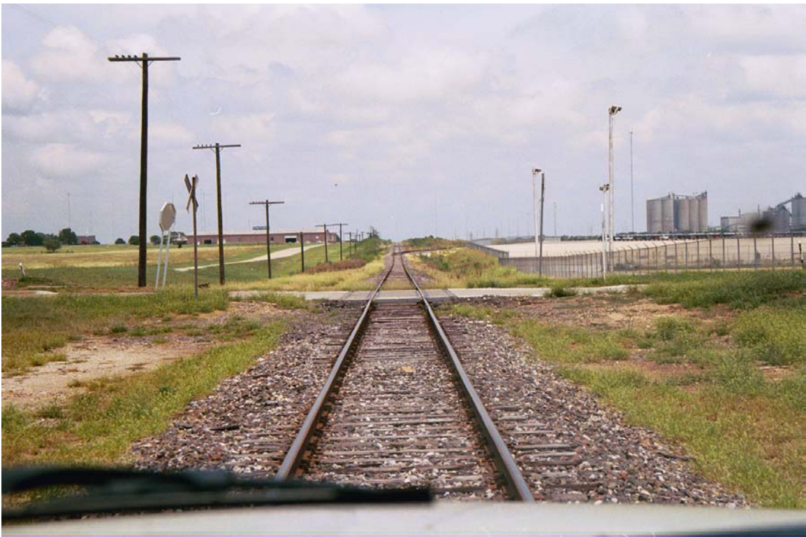
MP 27.5 Private crossing auto facility at right
