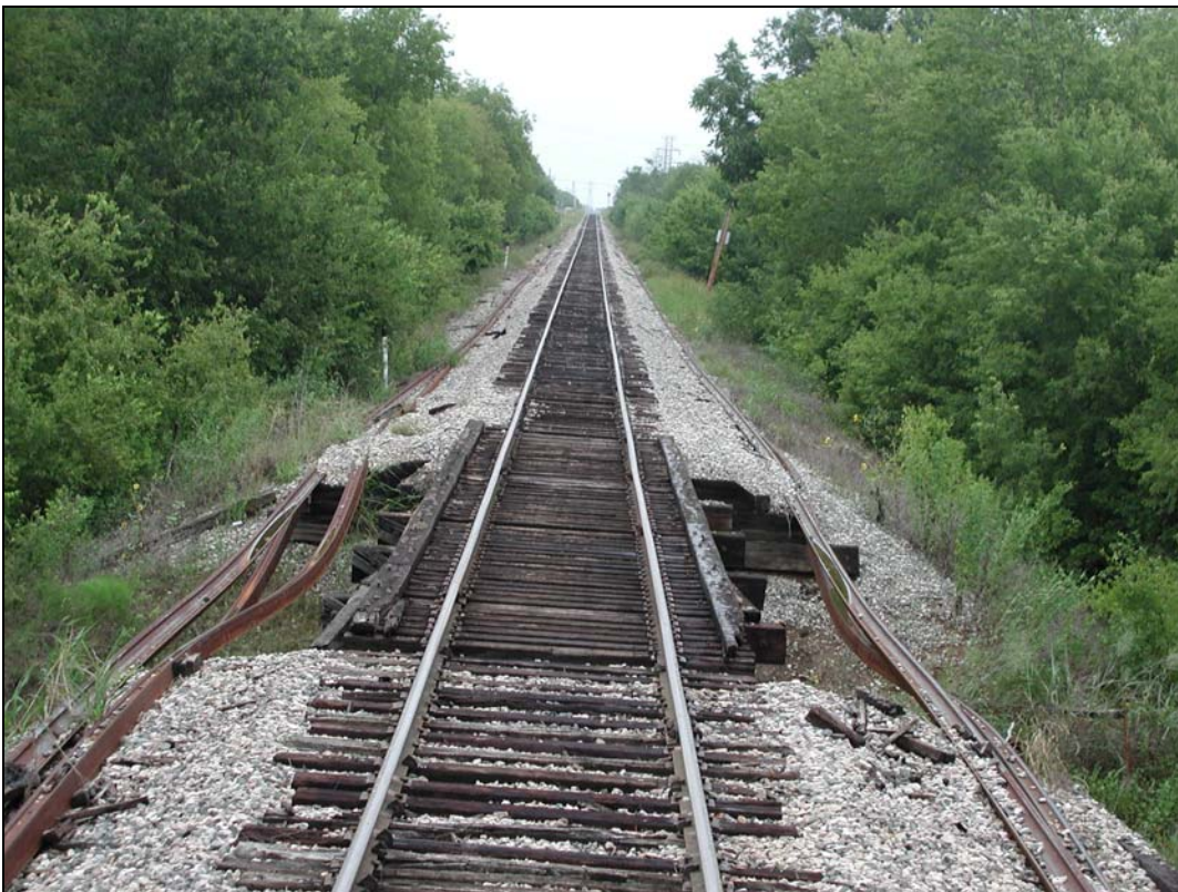
Looking east at Little Fossil Creek Bridge (East Track Crossing)
