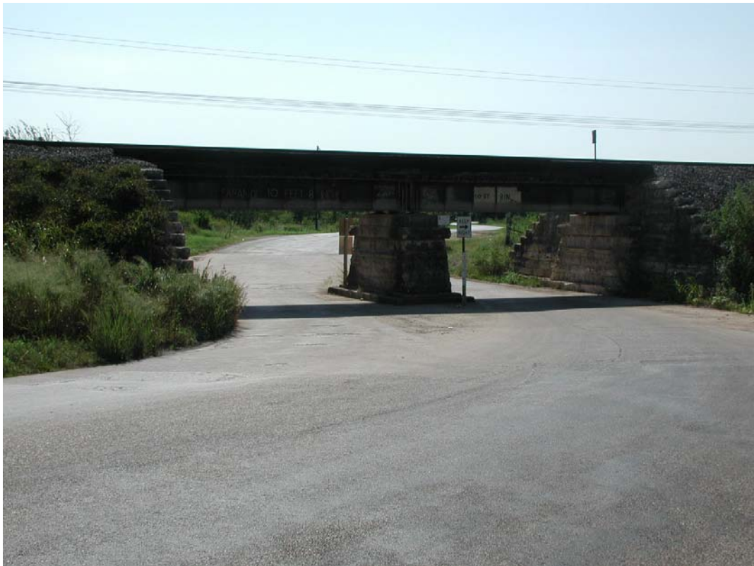
Looking East at bridge at MP 330.0
