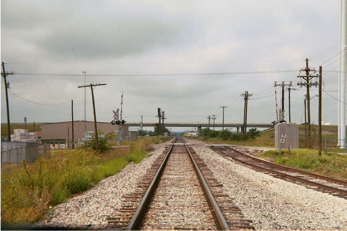
MP 794.7 Solon crossing with HWY 287 overpass in distance
