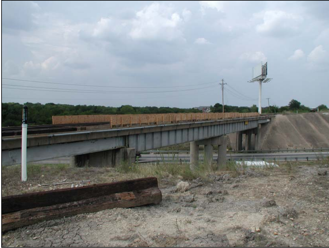
Looking south at Loop 820 (Railroad Overpass)
