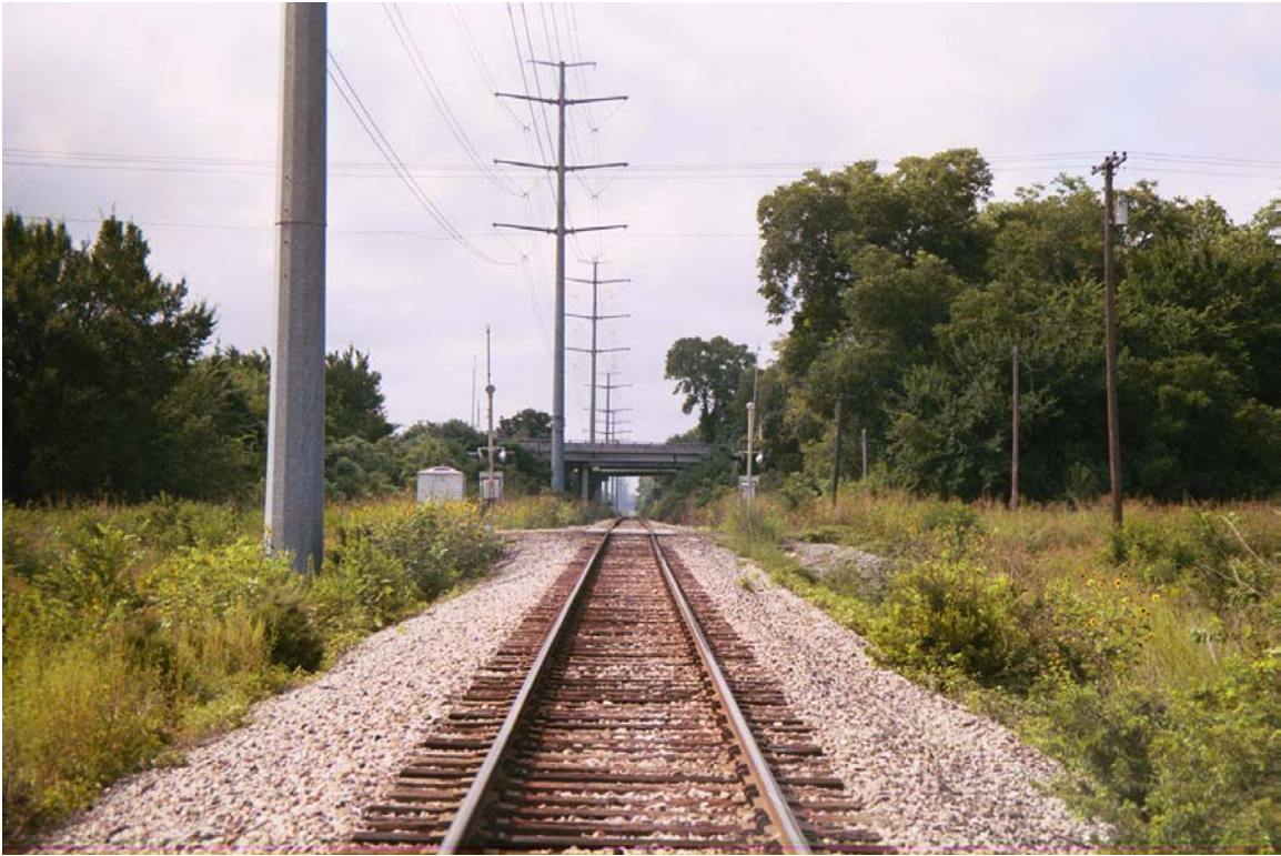
MP 773.7 Ledbetter Dr and HWY 12 Loop overpass
