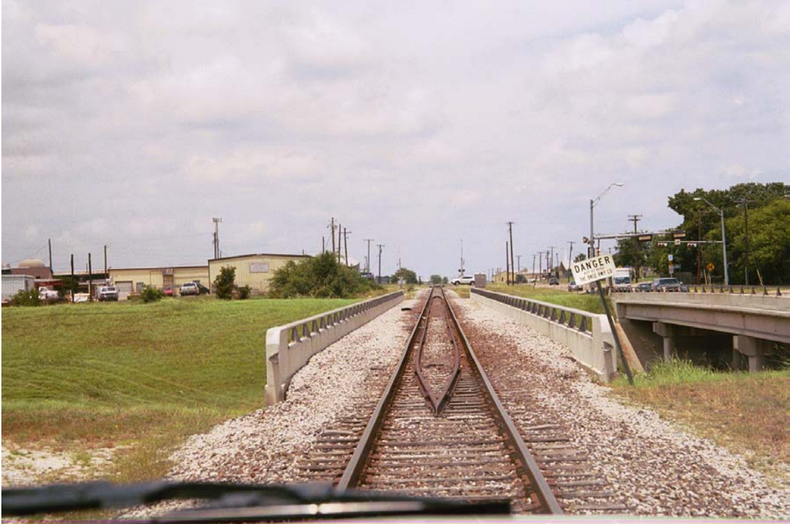
MP 40.7 Bridge over I-20 with Red Bird Rd in distance
