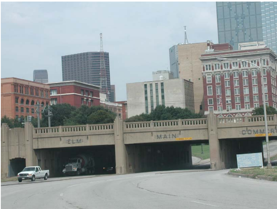
Looking East at west railroad bridge elevation over Elm, Main & Commerce
