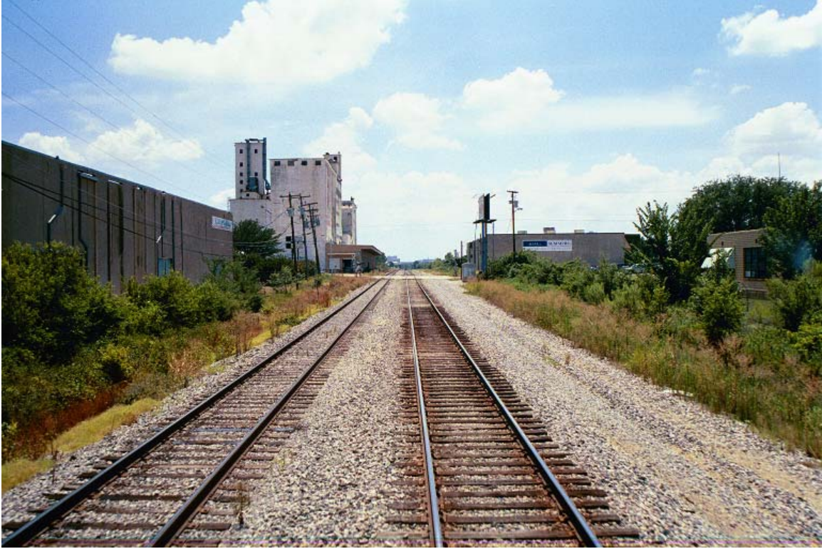
MP 614.2 Sylvania siding and Beach St crossing
