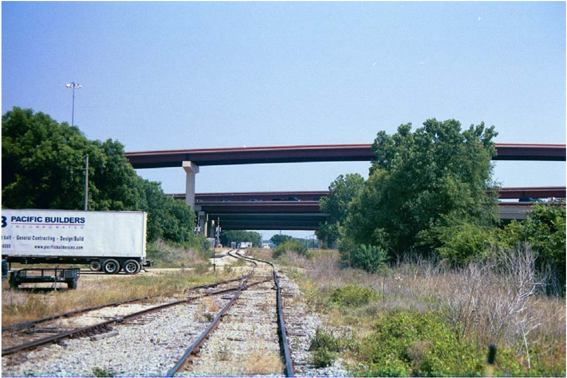
MP 742.3 - South end of siding and private road at Vanguard industry. SH-190 overpass.
