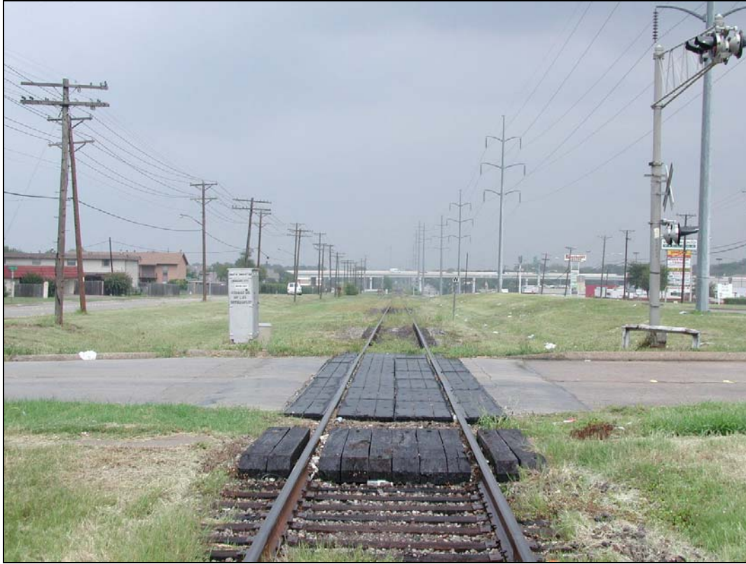
Looking North at Gorman
