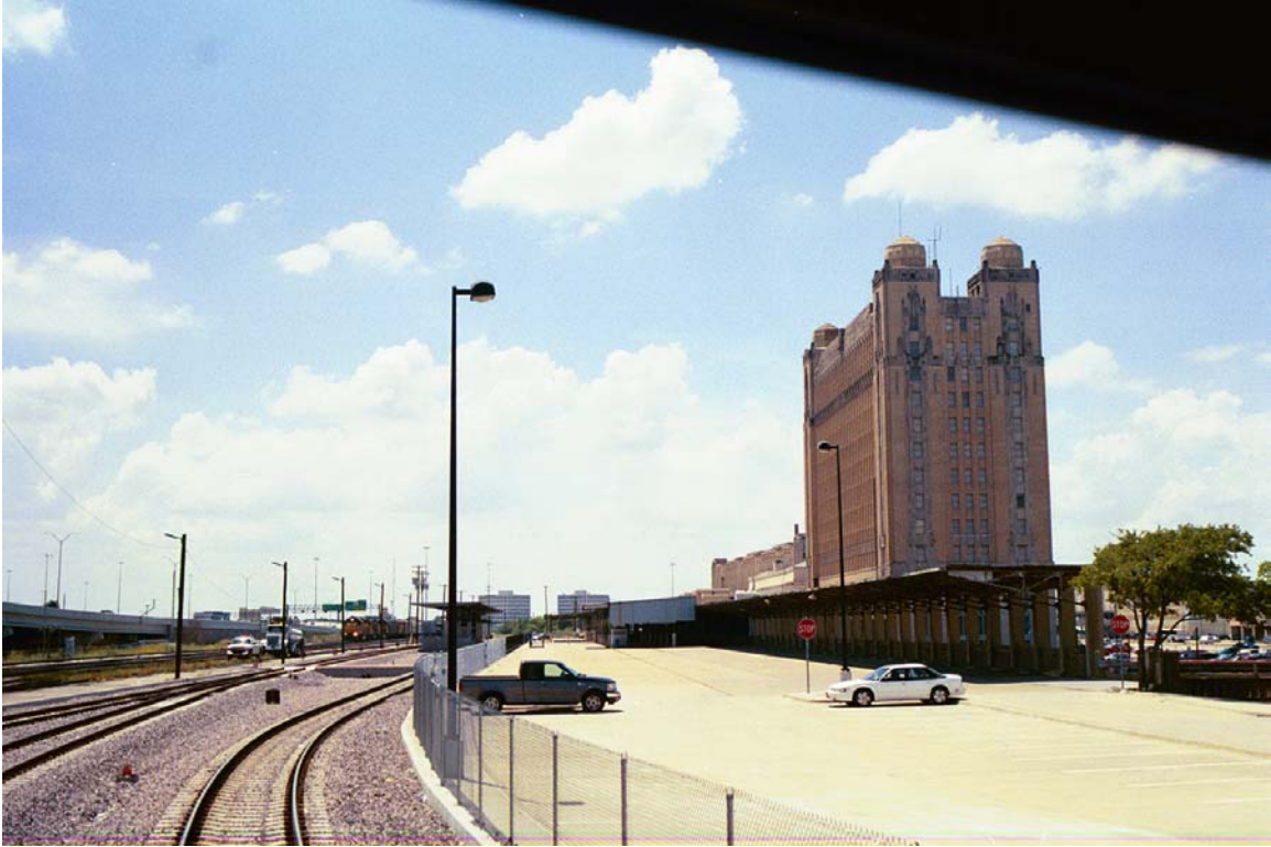
MP 610.5 T&P Depot in Fort Worth
