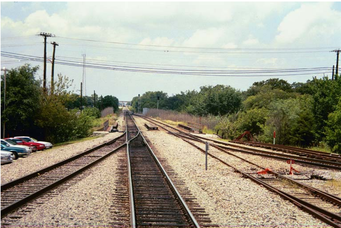
MP 634.4 WC Junction ,Sowers Rd crossing in distance
