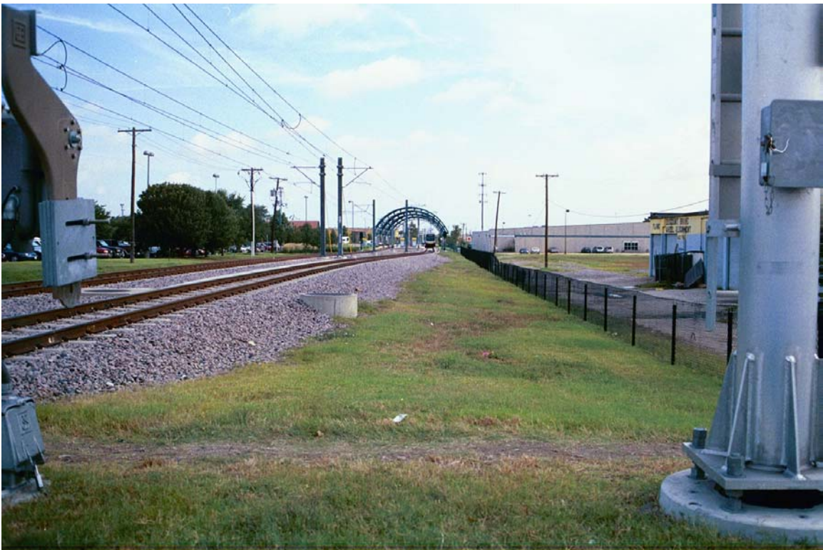
Looking North from Park Blvd. At Dart LRT Station in Plano
