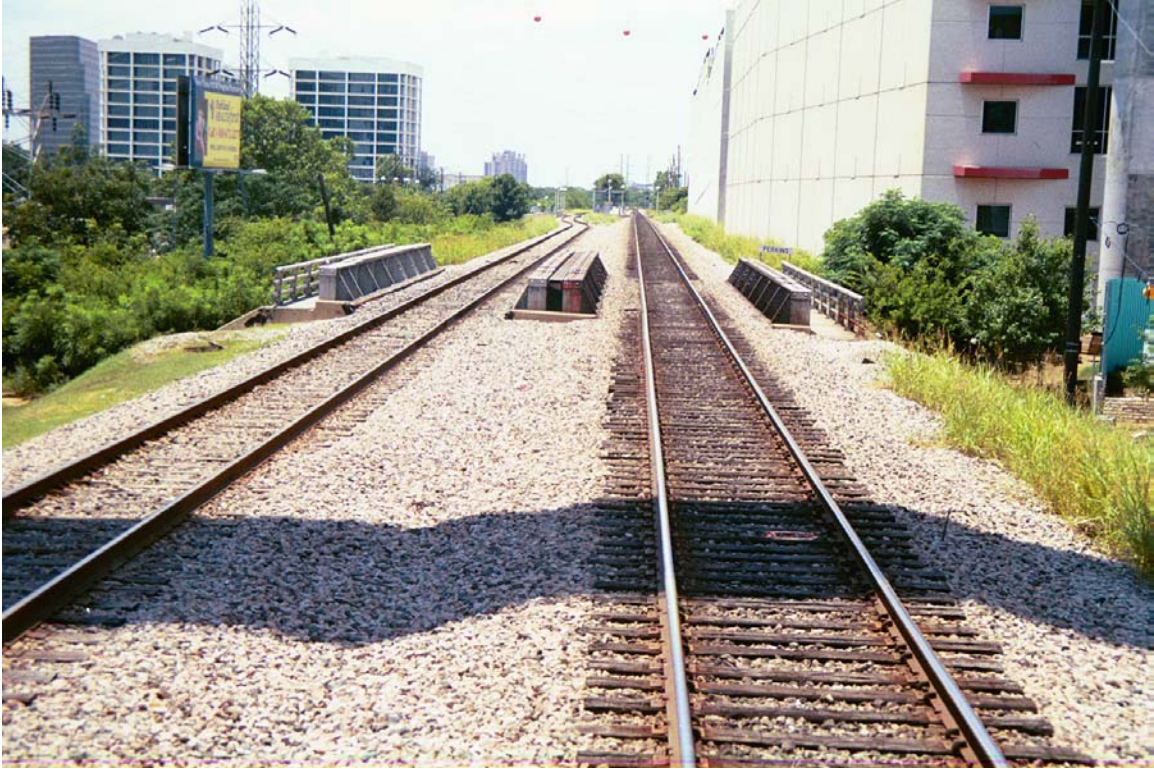
MP 641.6 Bridge over Market Center Blvd
