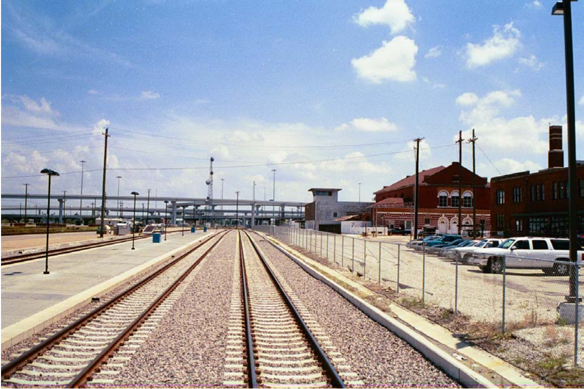
MP 610.8 Ex AT&SF Depot at right
