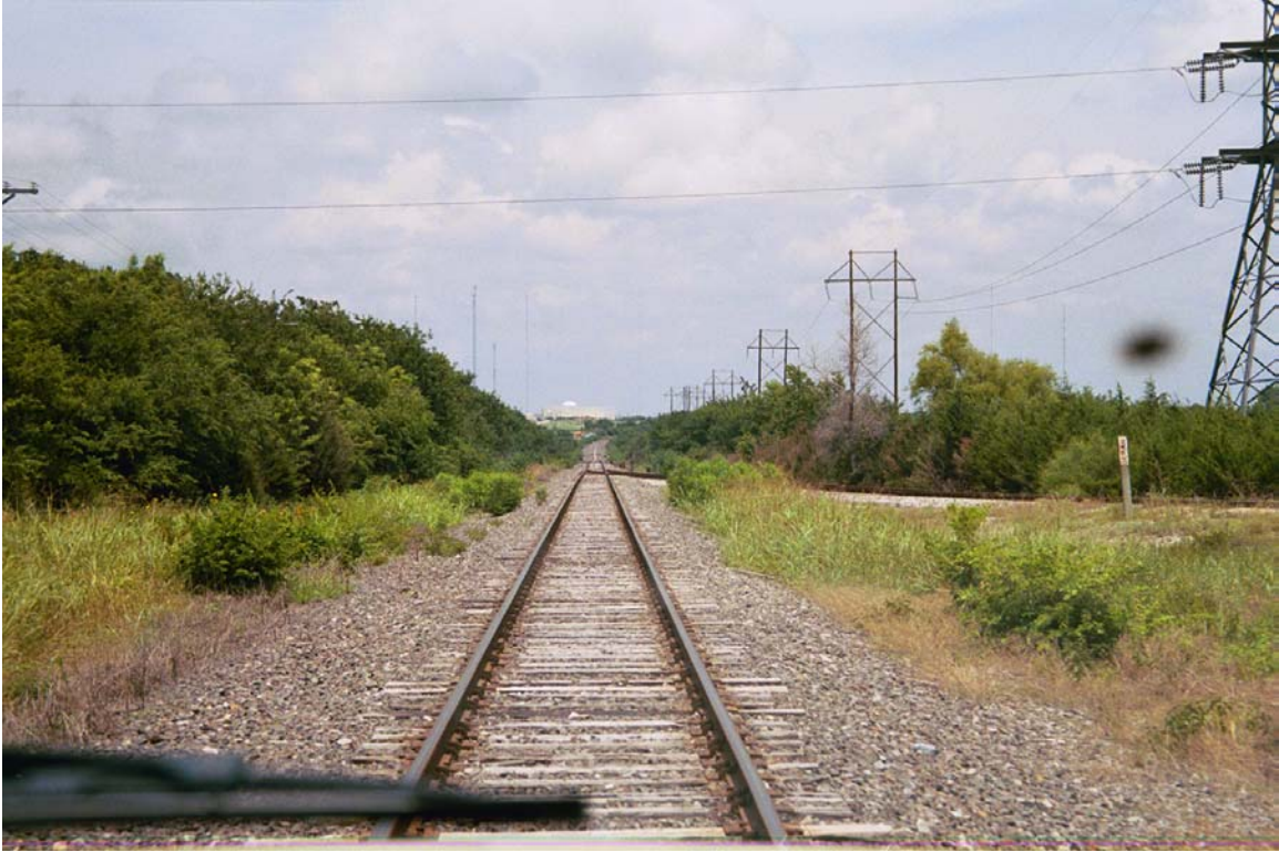
MP 29.4 Spur from cement plant
