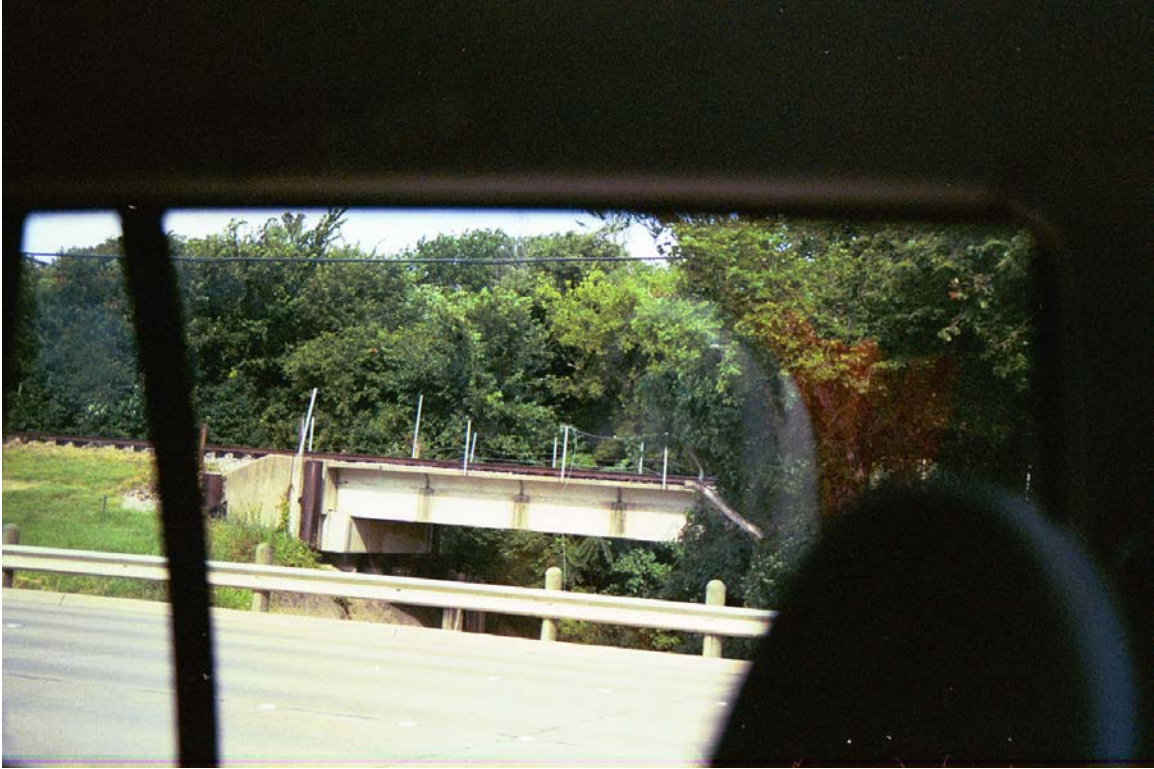
Rowlett Creek Bridge
