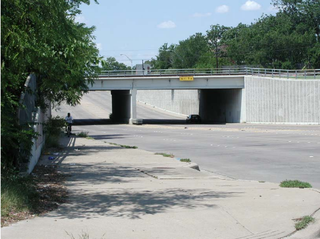
Looking at west bridge elevation of West Berry
