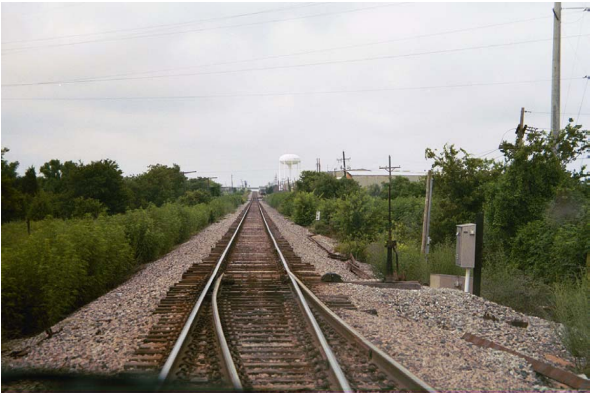
MP 794.0 between Service and Armaglass
