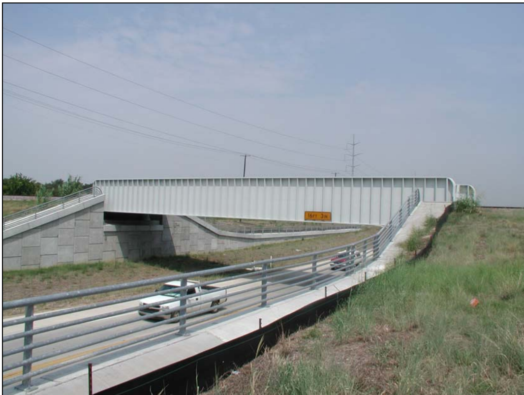
Looking North at Railroad Bridge over Business 114 (Loop 382)
