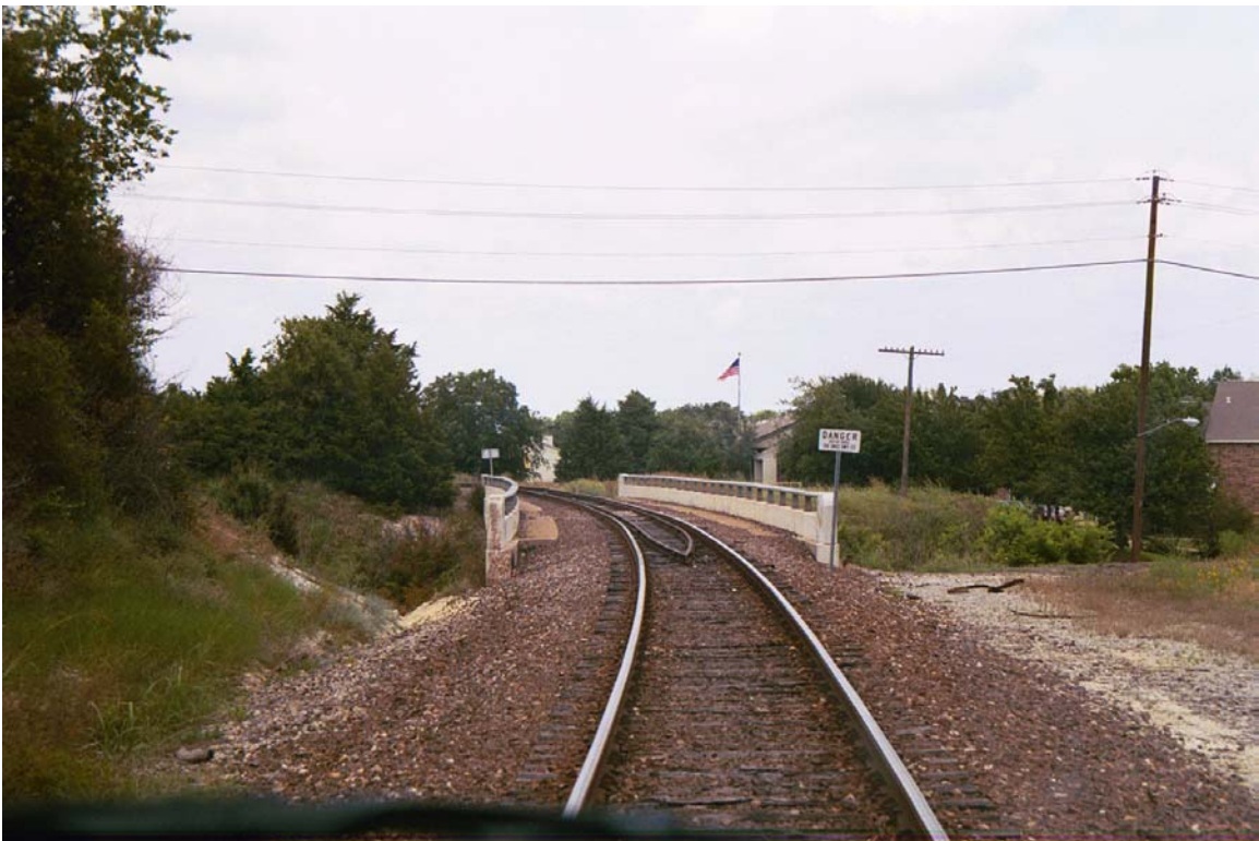
MP 42.6 Bridge over Ledbetter Drive
