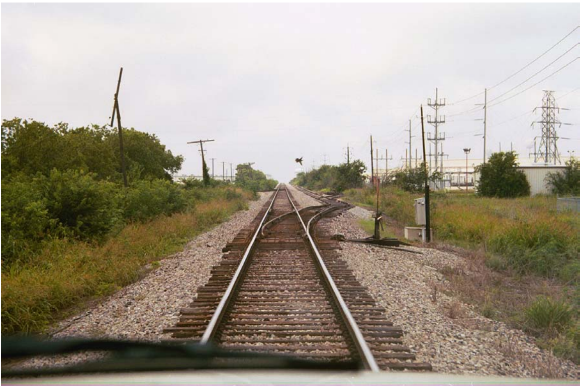
MP 793.2 North end of Service siding
