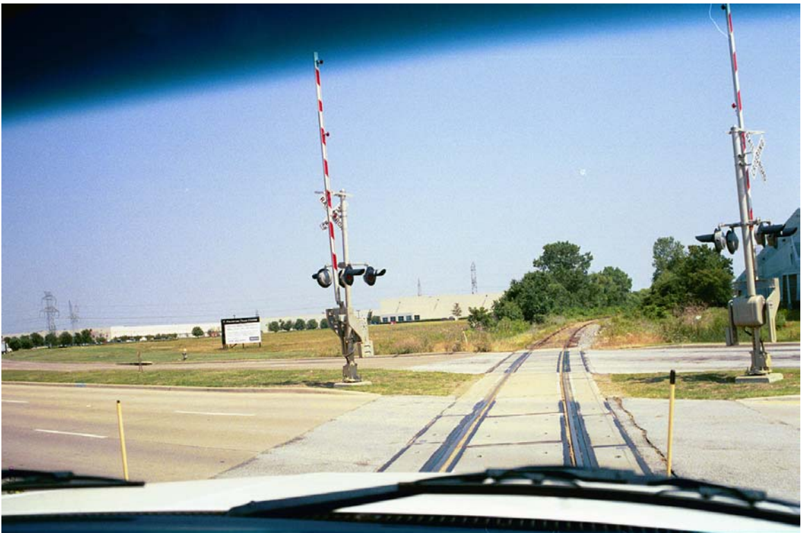
MP 741.8 - Frankfort Road crossing looking south. Potential passenger rail station site in southeast quadrant.
