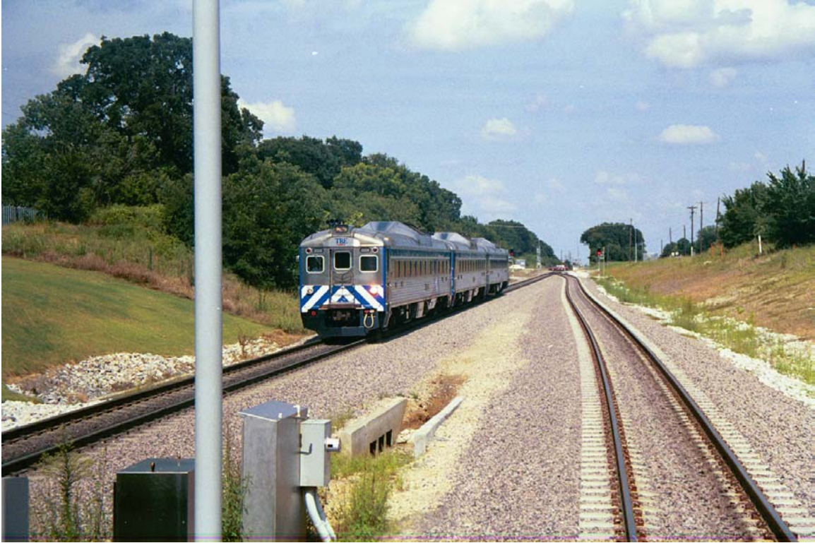
MP 631.4 W Irving Station Looking East
