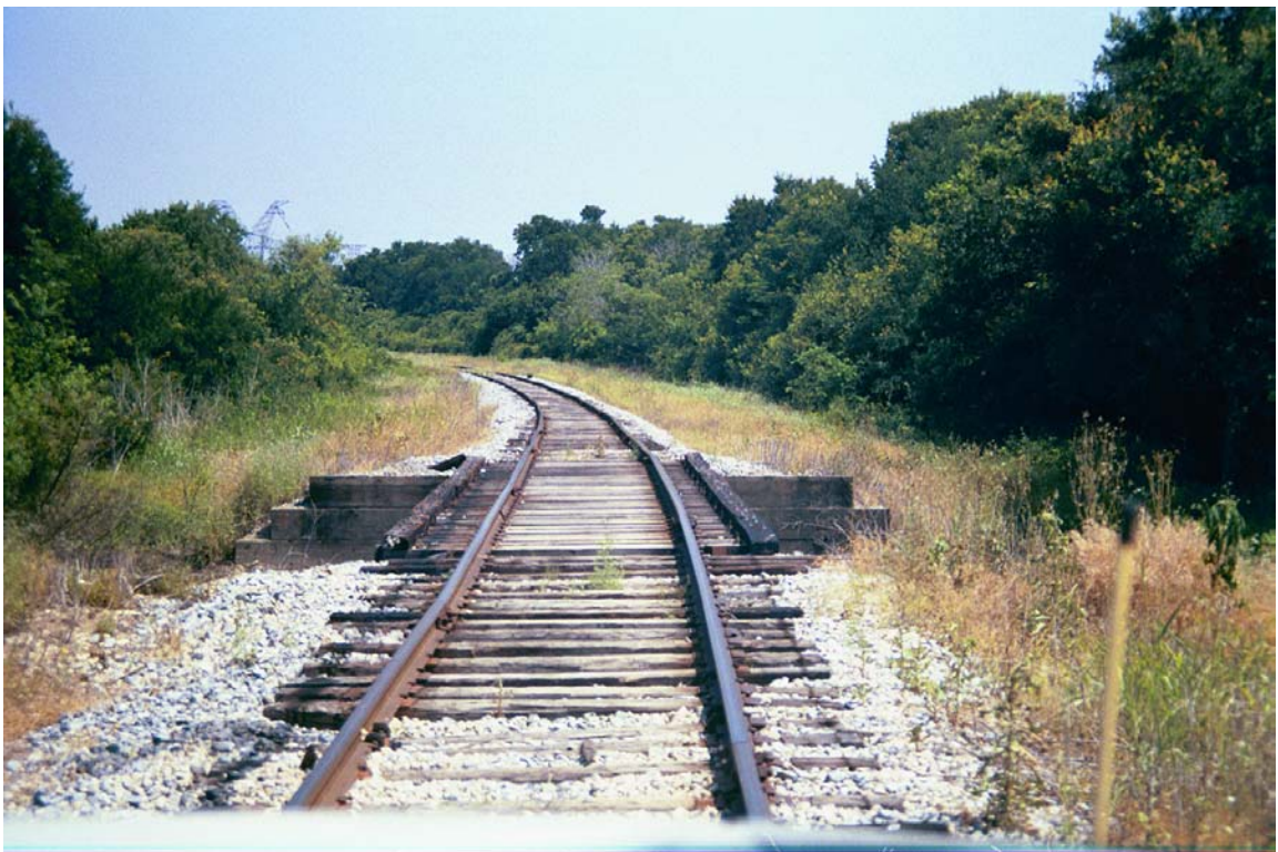
MP 740.6 – Bridge is 56' in length
