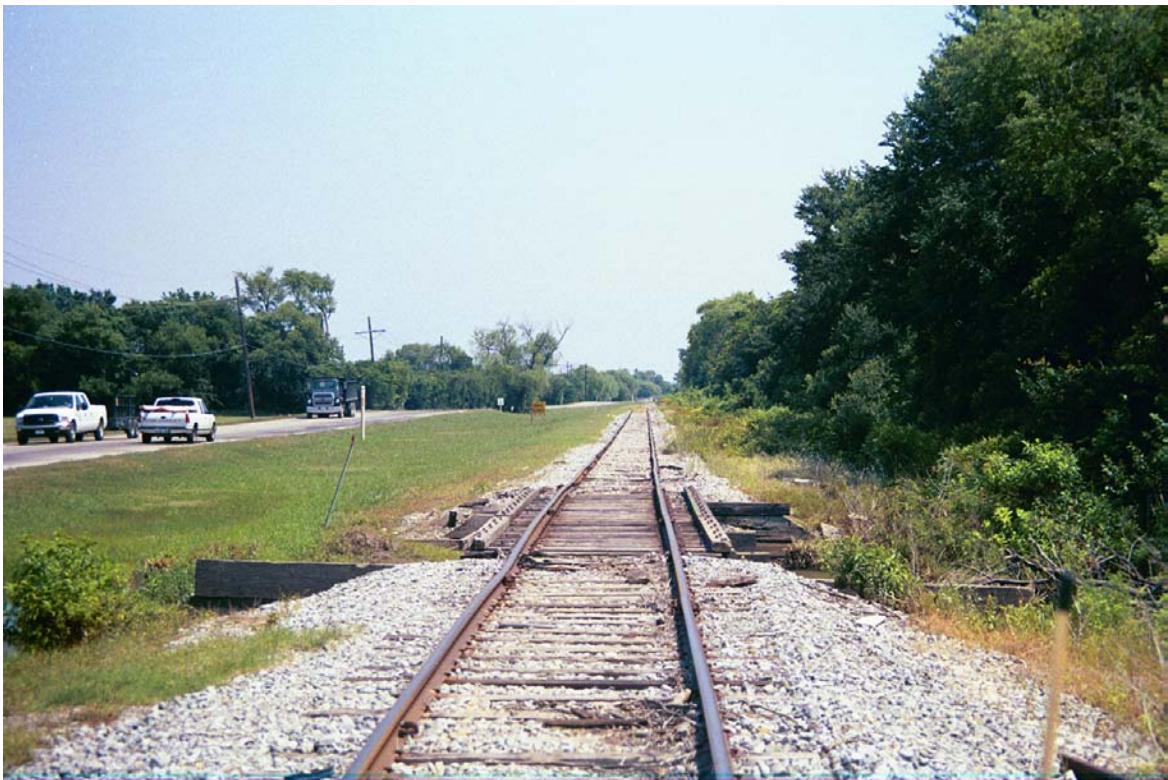
MP 738.5 – Bridge is 42' in length
