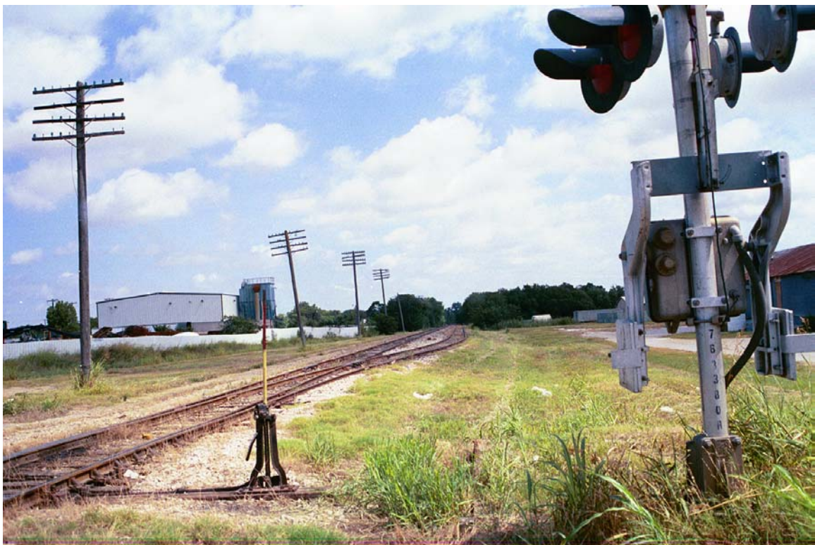
Looking North from Virginia St, Potential Station Site
