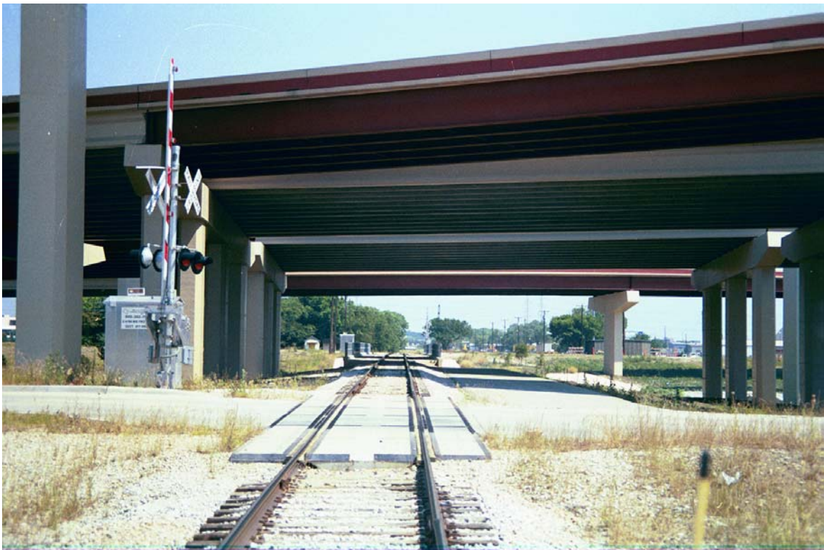
MP 742.4 – Trinity Mills Road crossing adjacent to SH-190 overpass.
