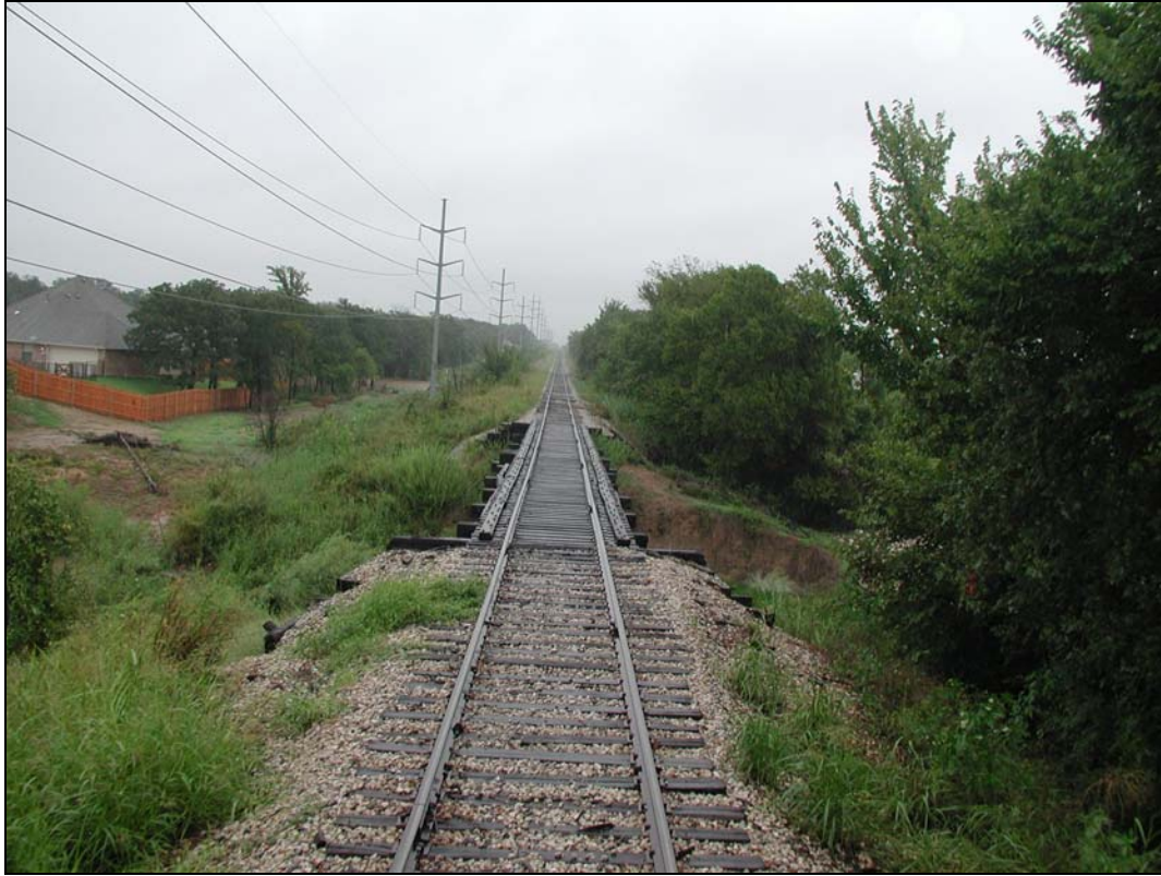
Looking East at Bear Creek Bridge – MP 17.5
