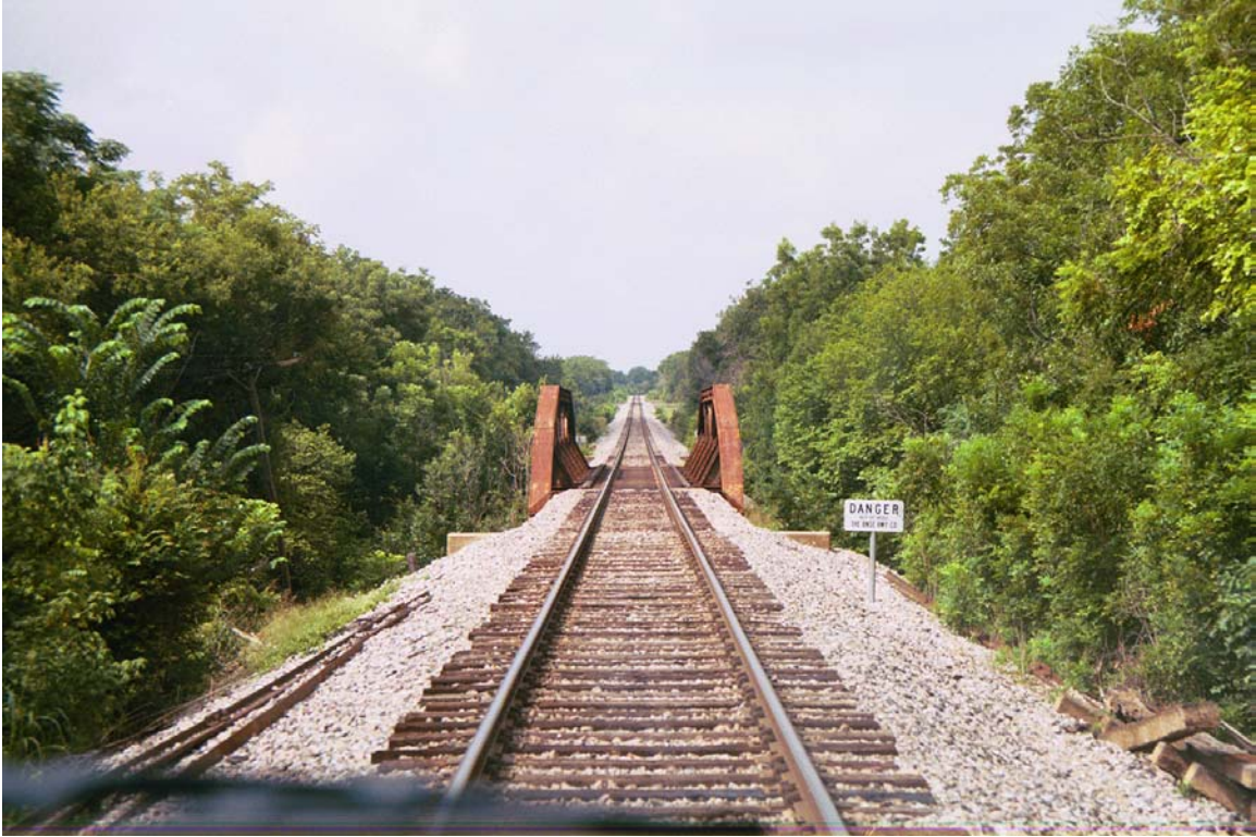
MP 789.1 Red Oak Creek bridge
