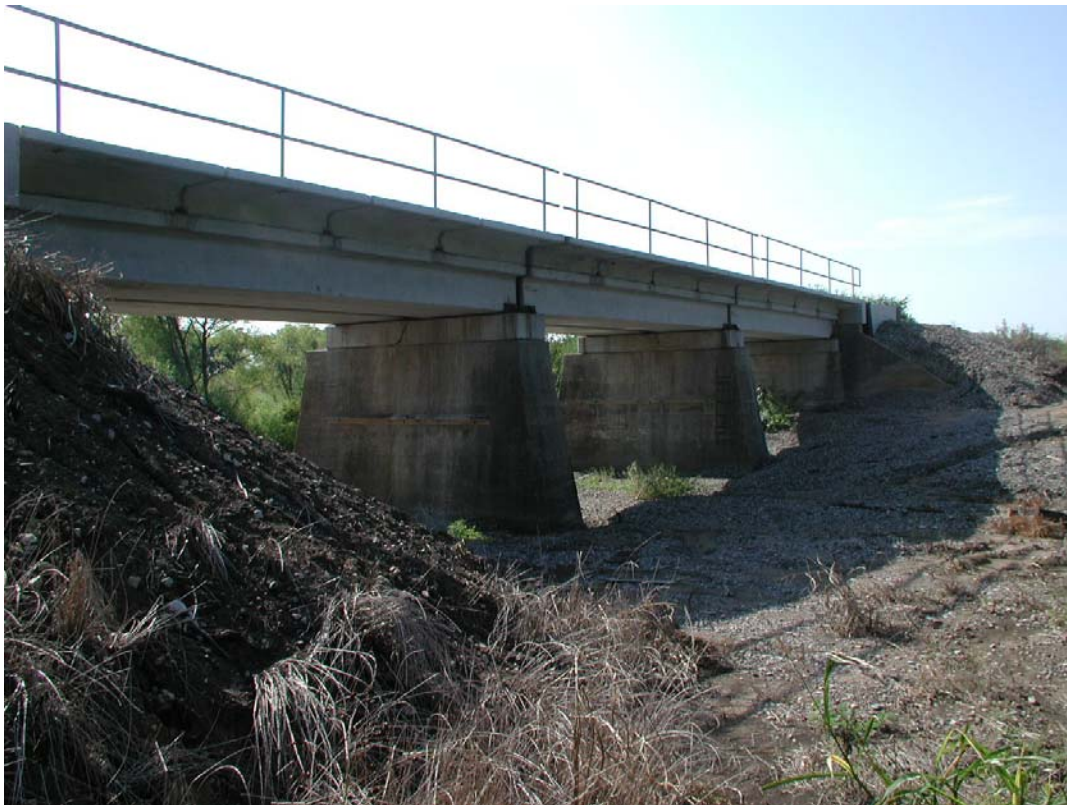
Looking at the west elevation of bridge at MP 322.6
