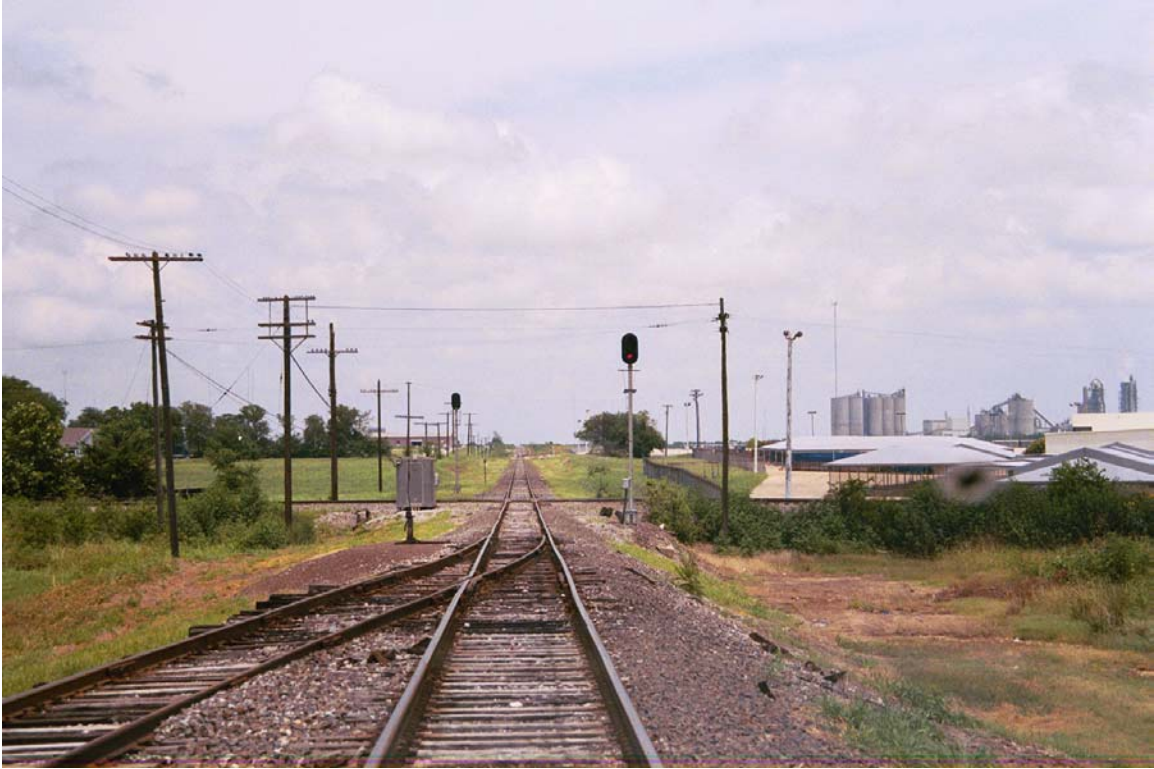
MP 27.3 SP crossing (now UP) of BNSF
