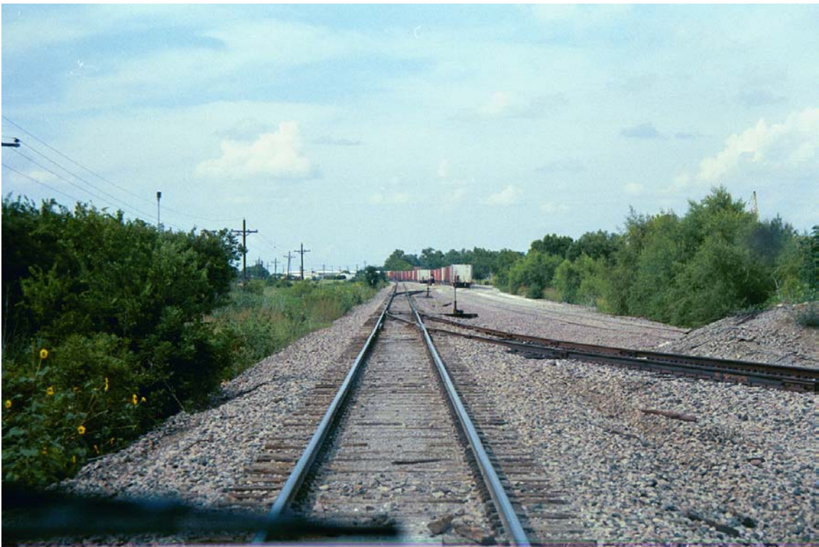
MP 686.3 Looking North toward Frisco
