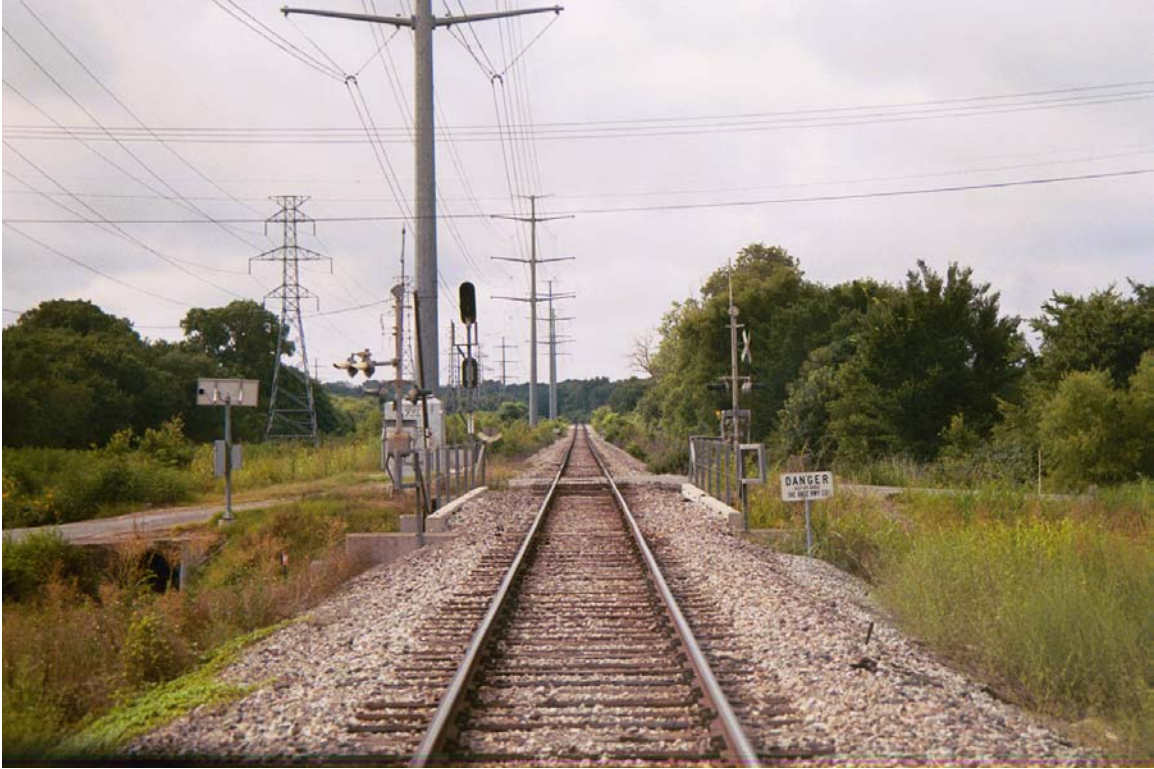
MP 771.1 Southerland Arena
