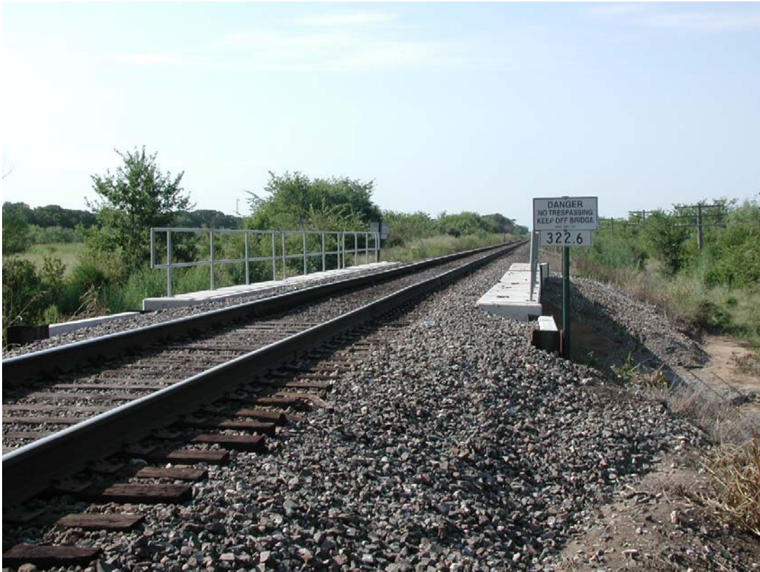
Looking South on bridge at MP 322.6
