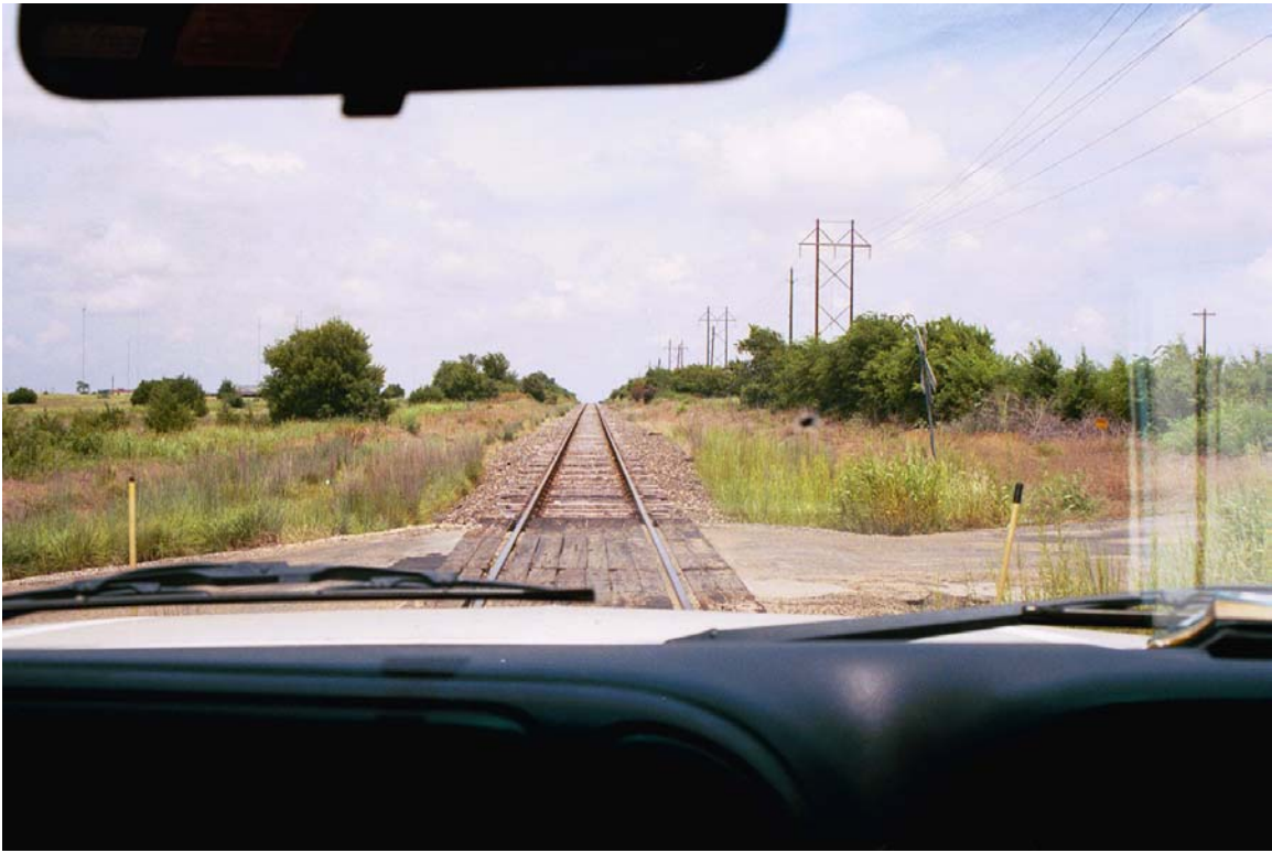
MP 30.6 Public crossing
