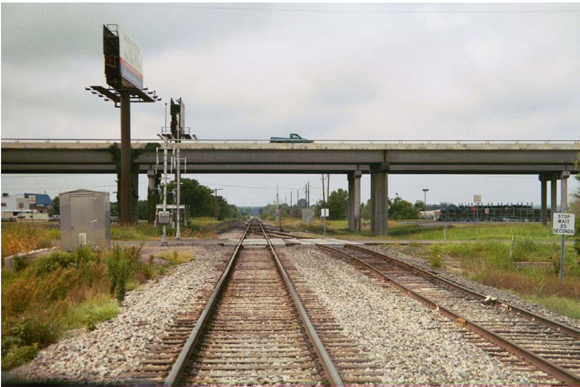
MP 794.9 HWY 287 overpass and access ramps on each side
