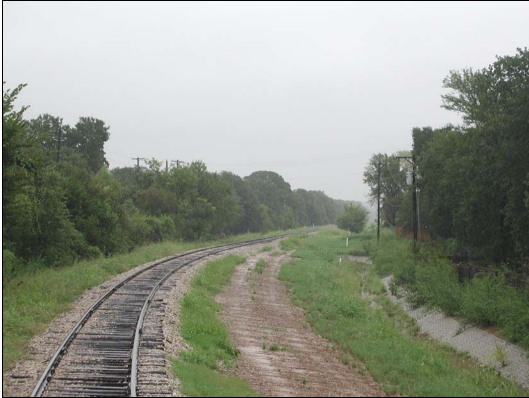
Concrete Culvert – Between John McCain & Pleasant Run
