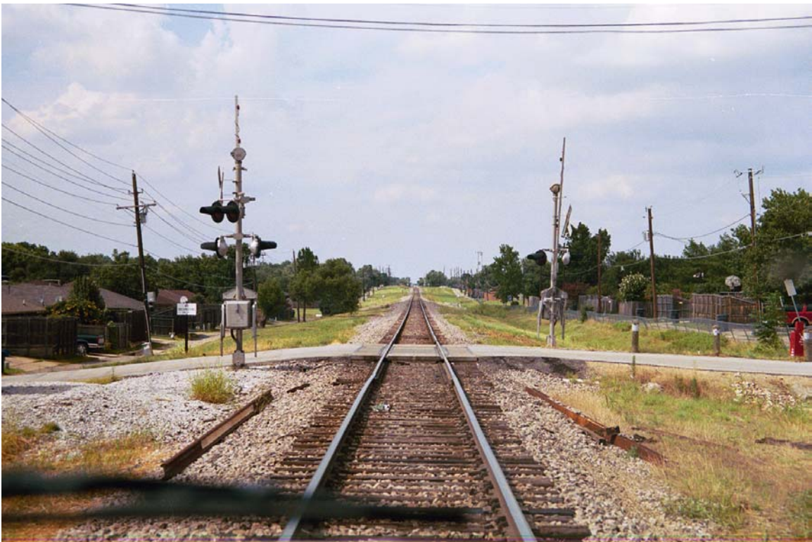
MP 697.2 Old Mills Rd
