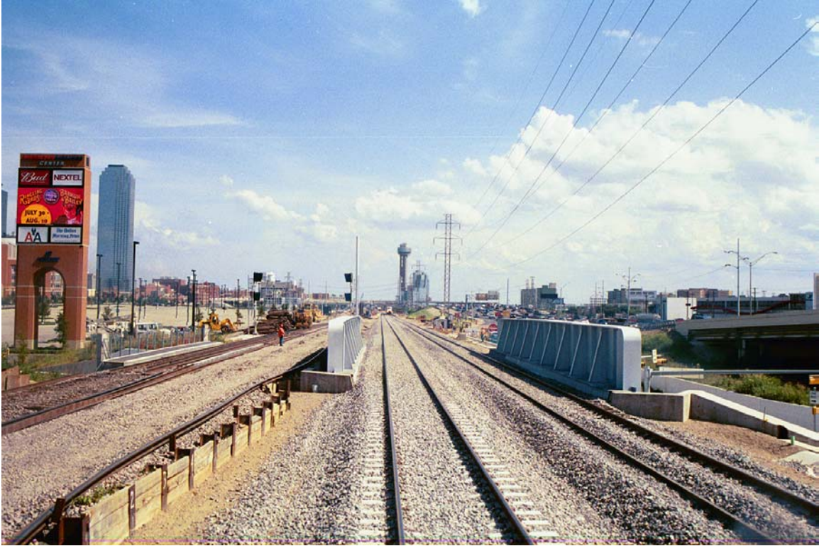
MP 642.6 New AA Arena Station under Construction in distance
