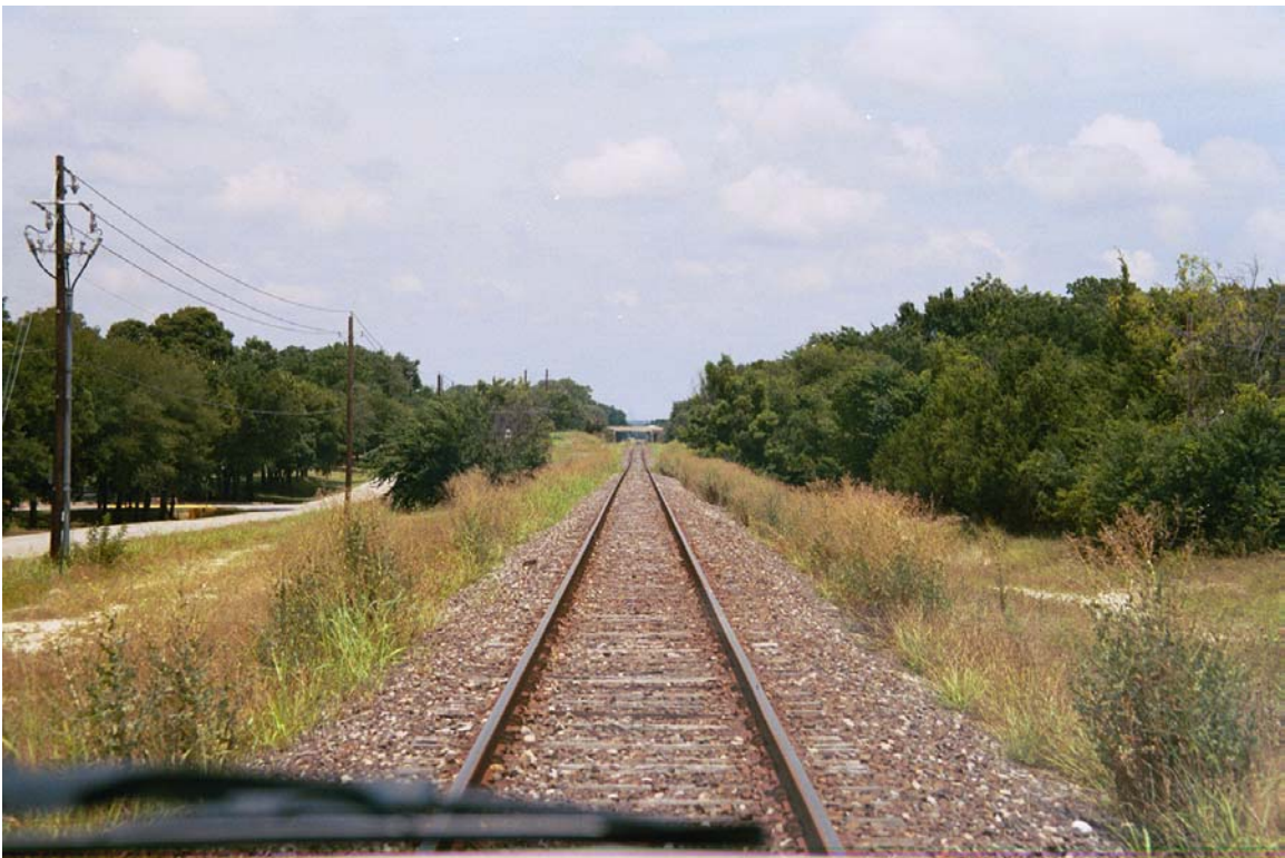
MP 35.5 FM 1382 overpass in distance
