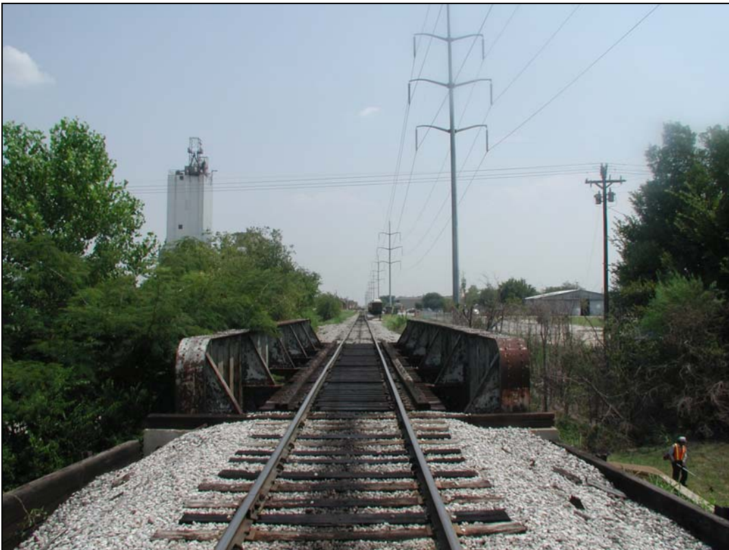
Looking East at RR over Hudgins St.
