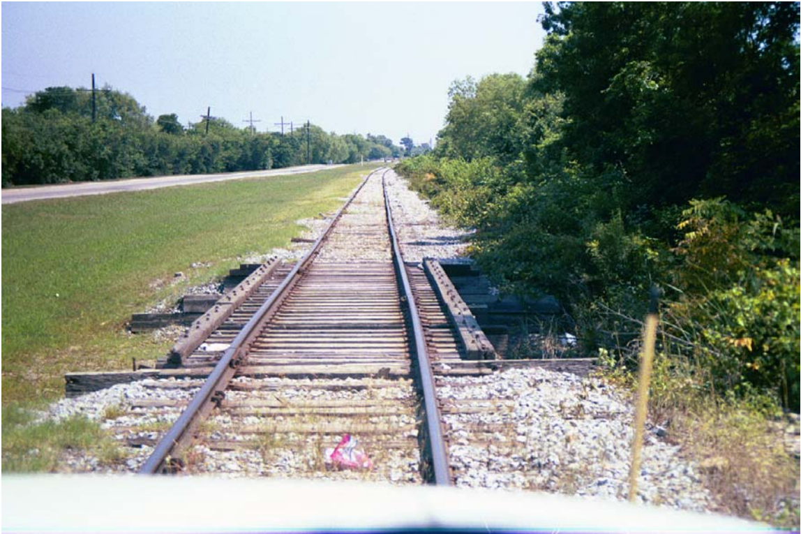
MP 738.6 – Fourth bridge within 0.3-mile is 42' in length
