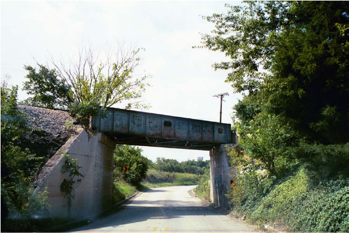
Texas State HWY 5 under railroad Looking NW
