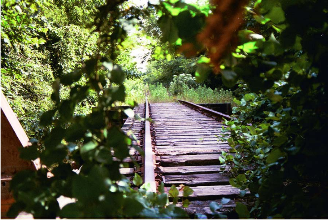
Cottonwood Creek Bridge Looking North
