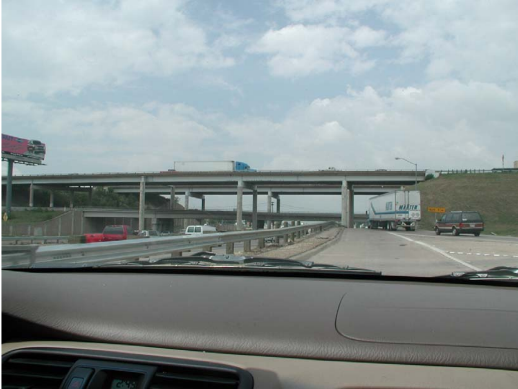
Looking North at south railroad bridge elevation over Loop 12
