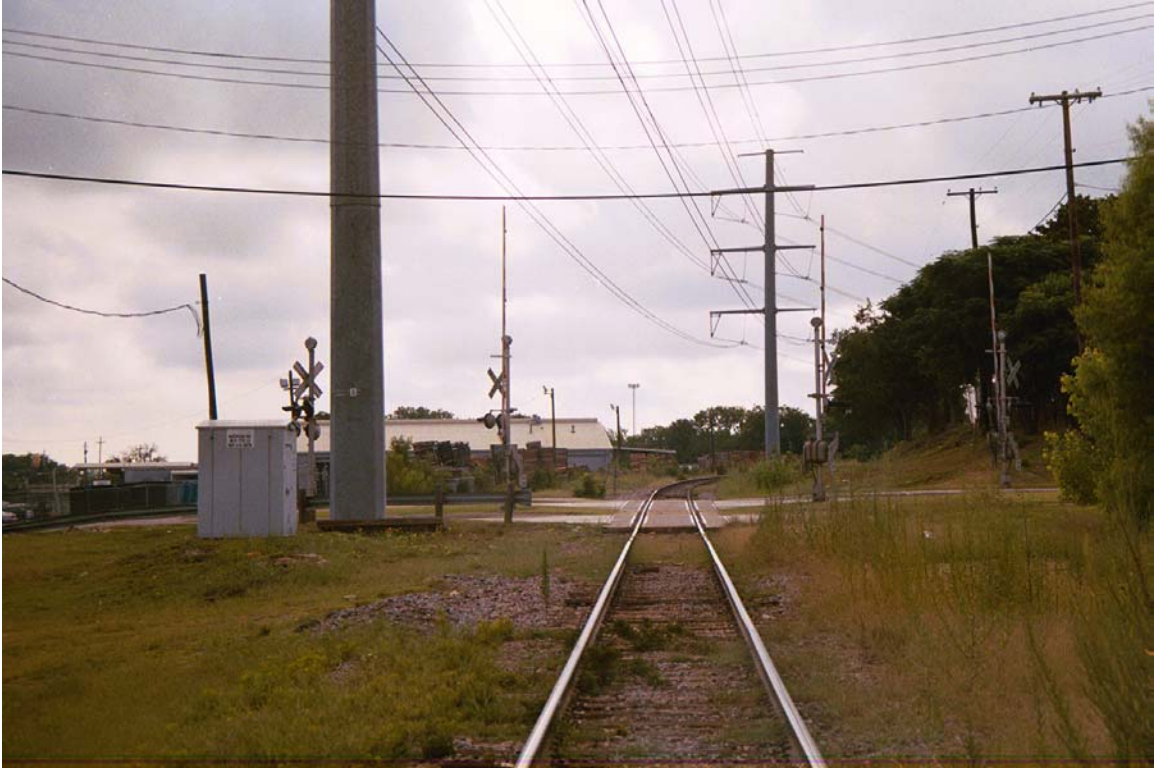
MP 772.1 Overton Rd
