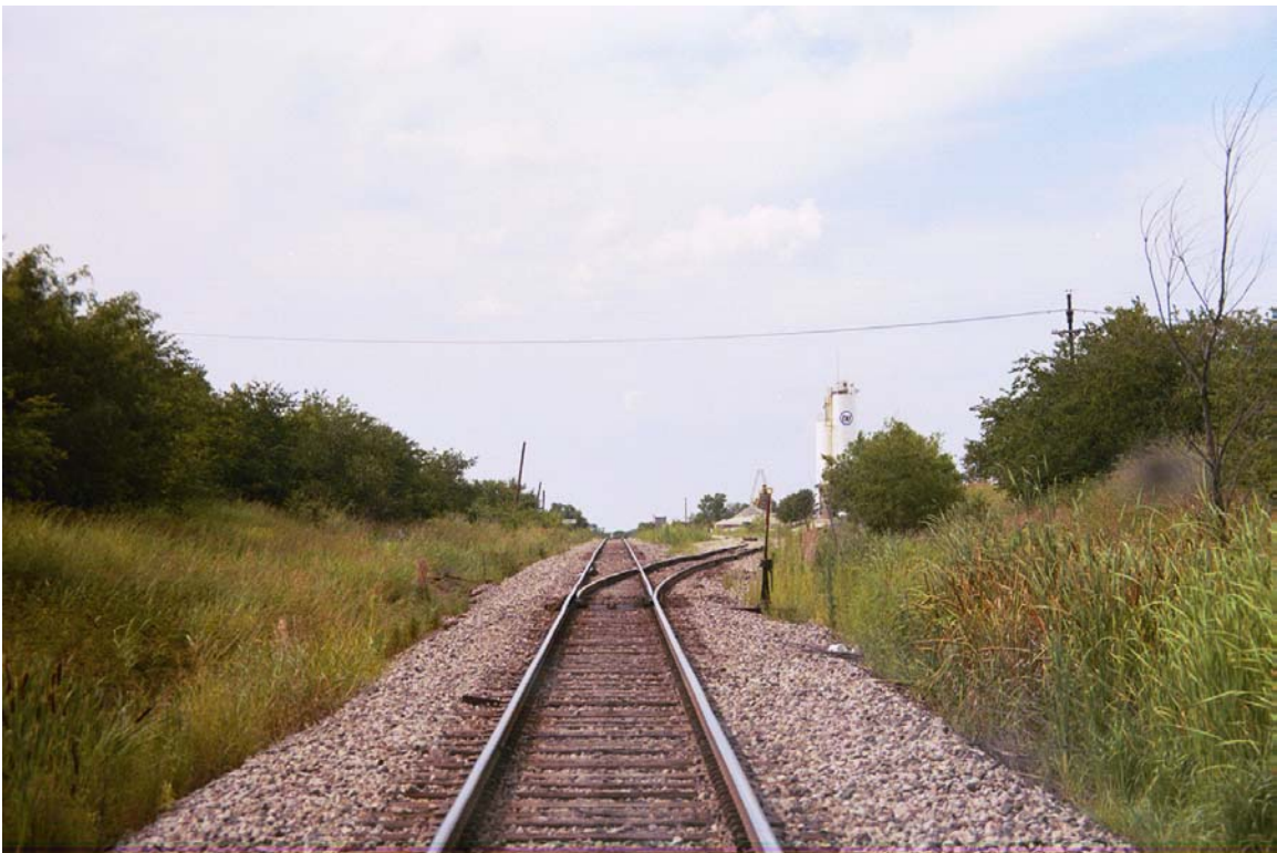
MP 690.8 South end of Camey Siding
