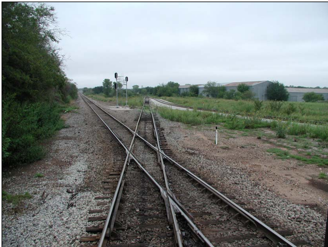
Looking east at BNSF/Cotton Belt Crossing
