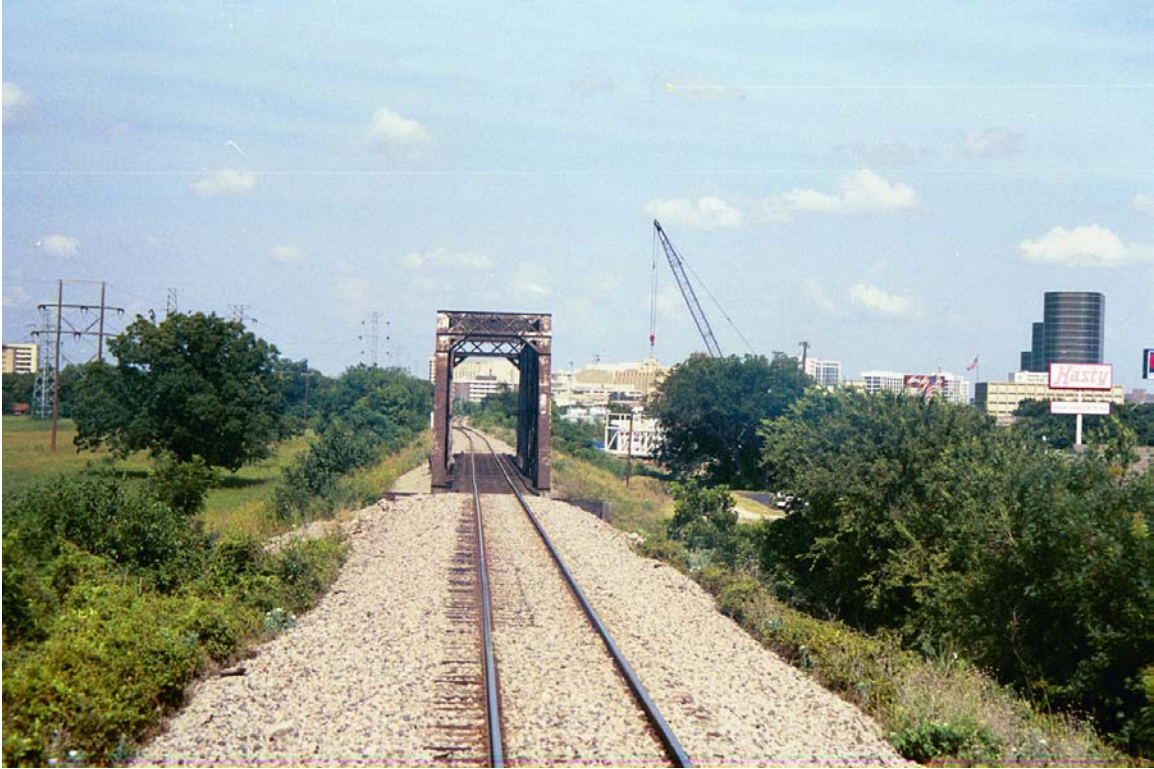
MP 639.9 Old Channel Bridge
