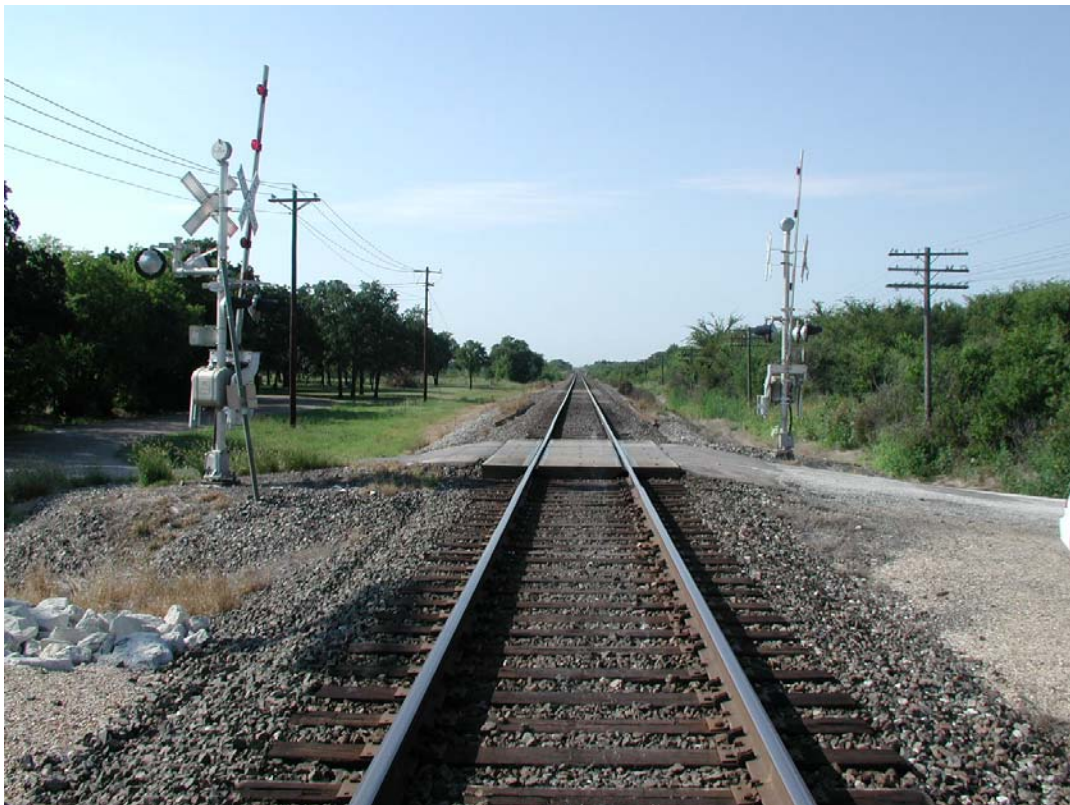
Looking West at CR903
