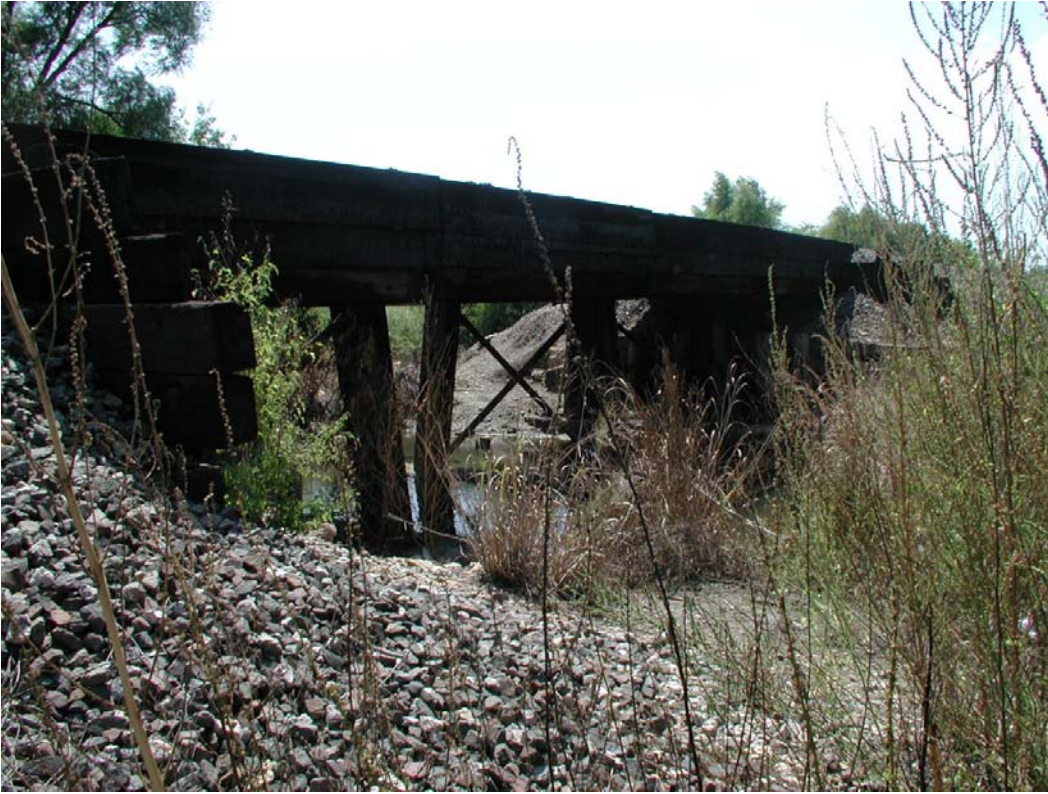
Looking at west bridge elevation on MP 336.7
