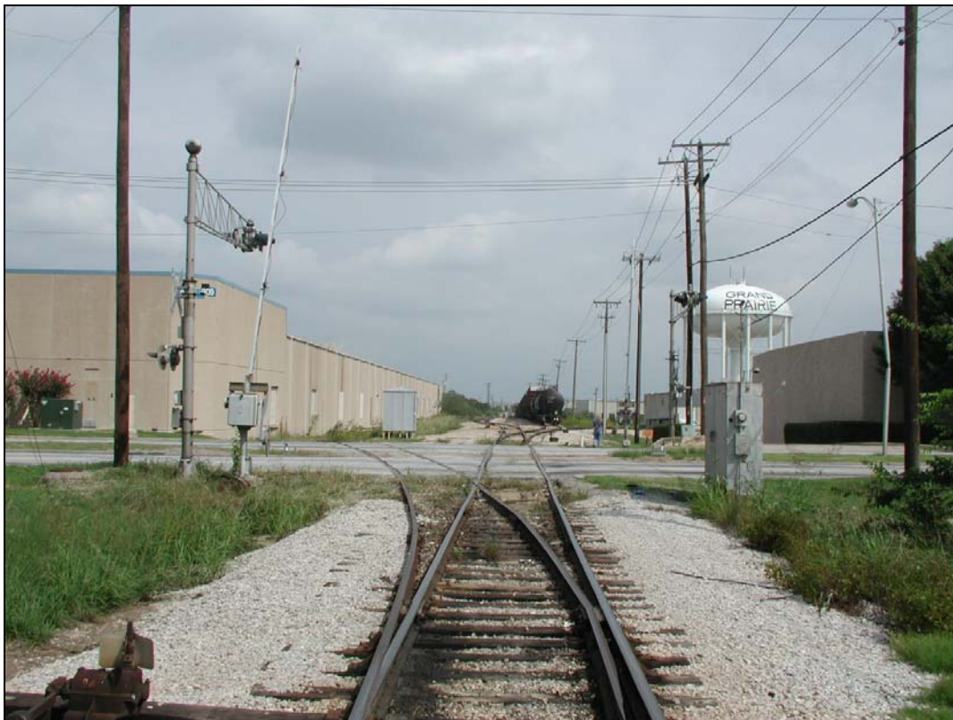
Looking north at North Carrier Parkway W.
