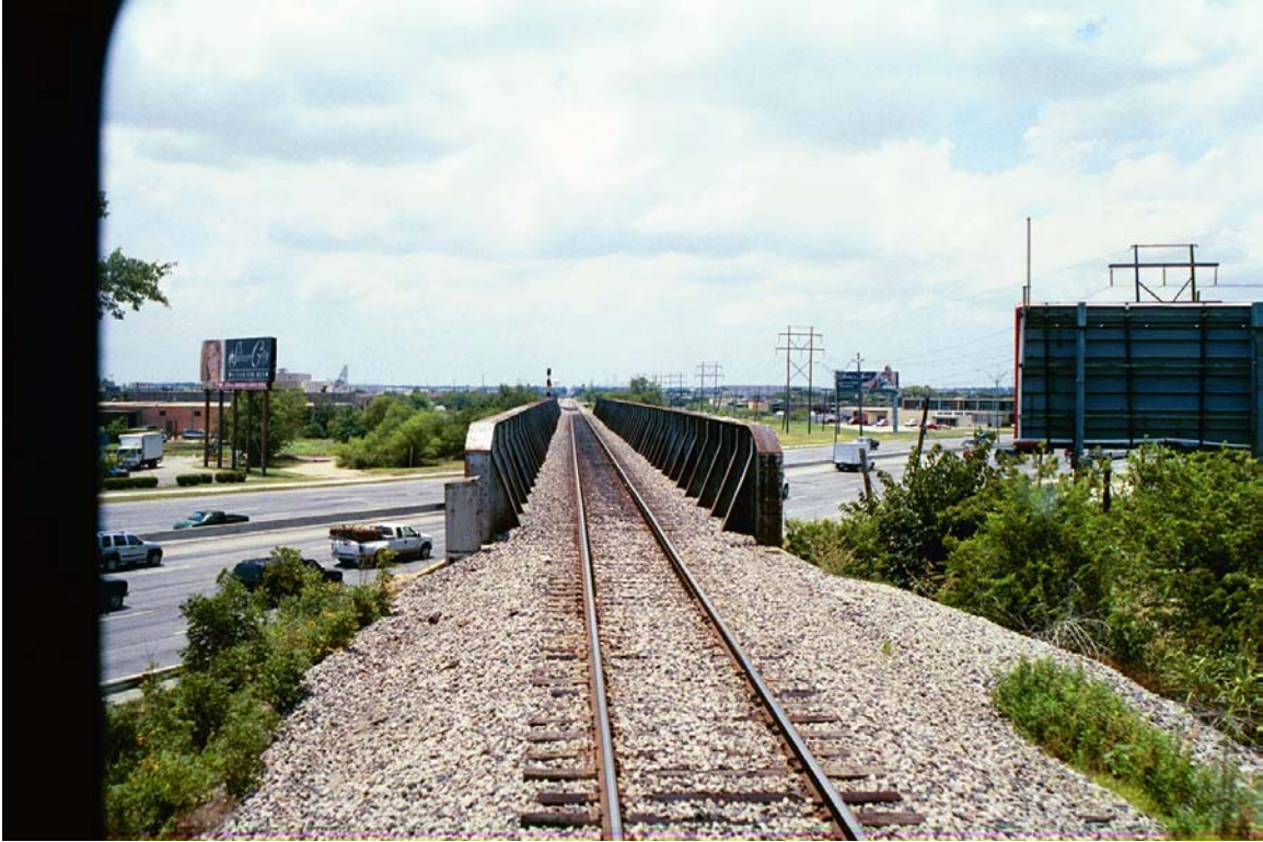
Near MP 640.0 Bridge over Stemmons Freeway
