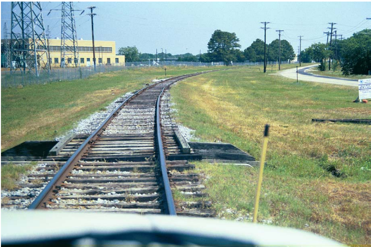
MP 743.2 – Timber culvert is 14 feet long with open deck
