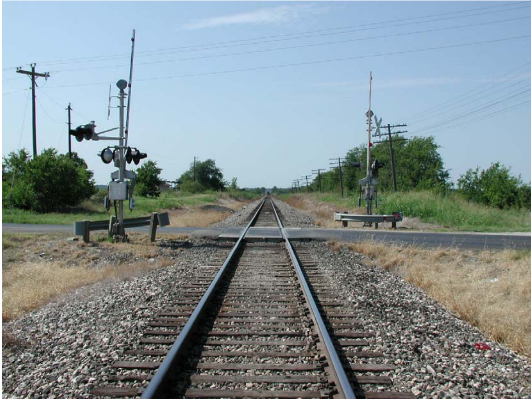
Looking South at CR921
