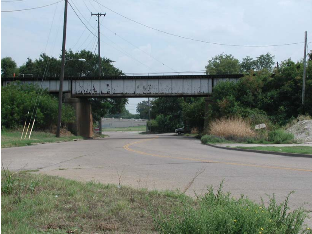
Looking South at north railroad bridge elevation over Beckley
