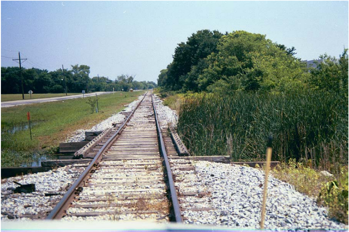
MP 738.4 – Bridge is 39' in length
