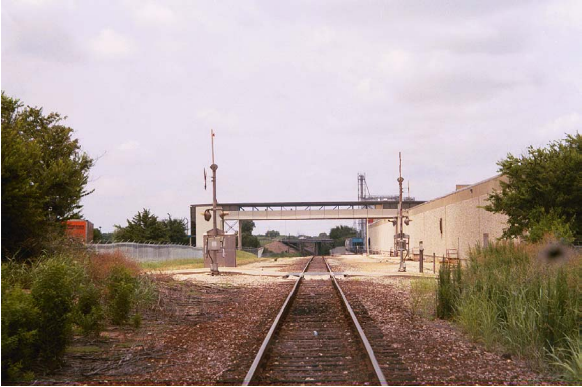
MP 43.3 Frito Lay Plant at Maglab
