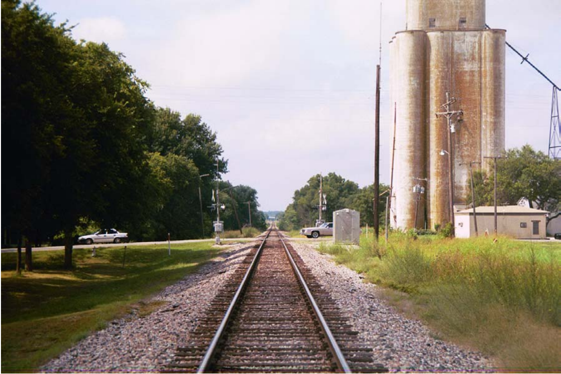
MP 780.9 Just North of Lancaster at Pleasant Run Rd crossing
