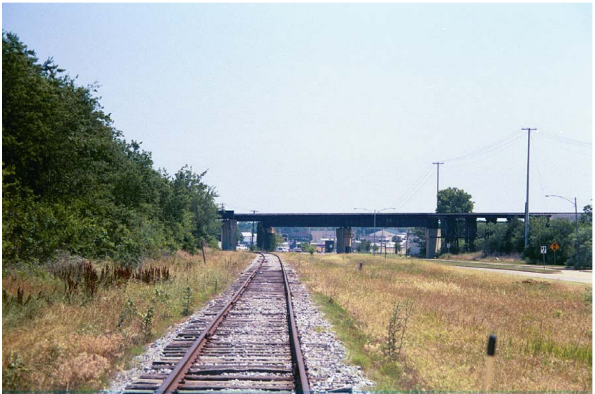
MP 735.4 – Looking south at KCS Railroad bridge
