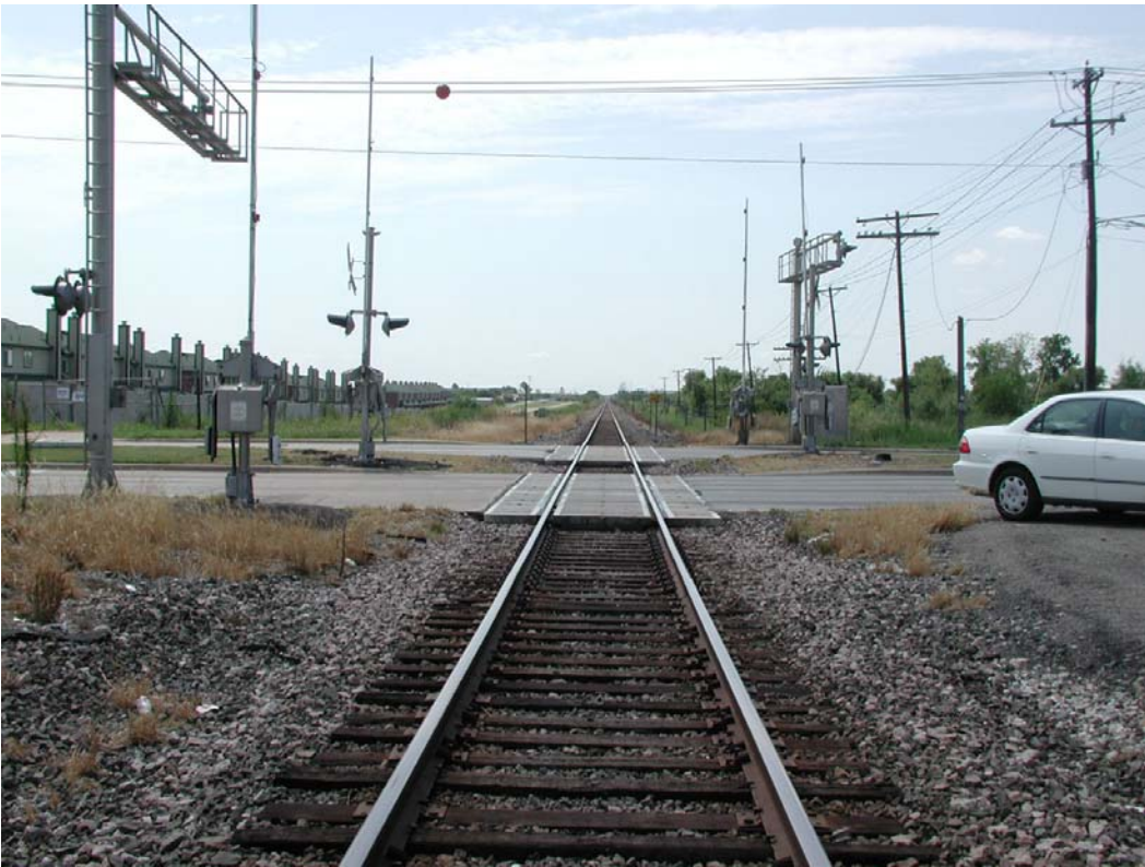
Looking South at Sycamore School Rd.
