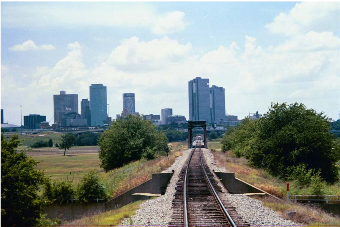
MP 612.4 Steel truss bridge over West Fork of Trinity River
