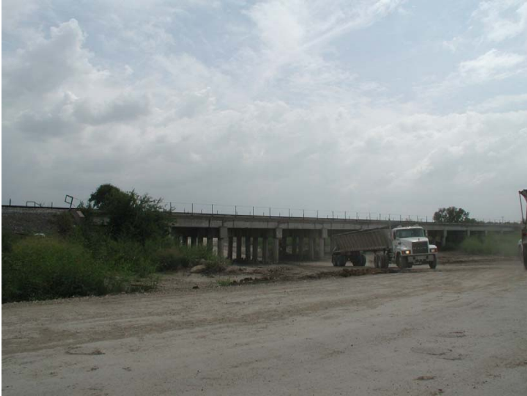
Looking South at north railroad bridge elevation at Sand Pit
