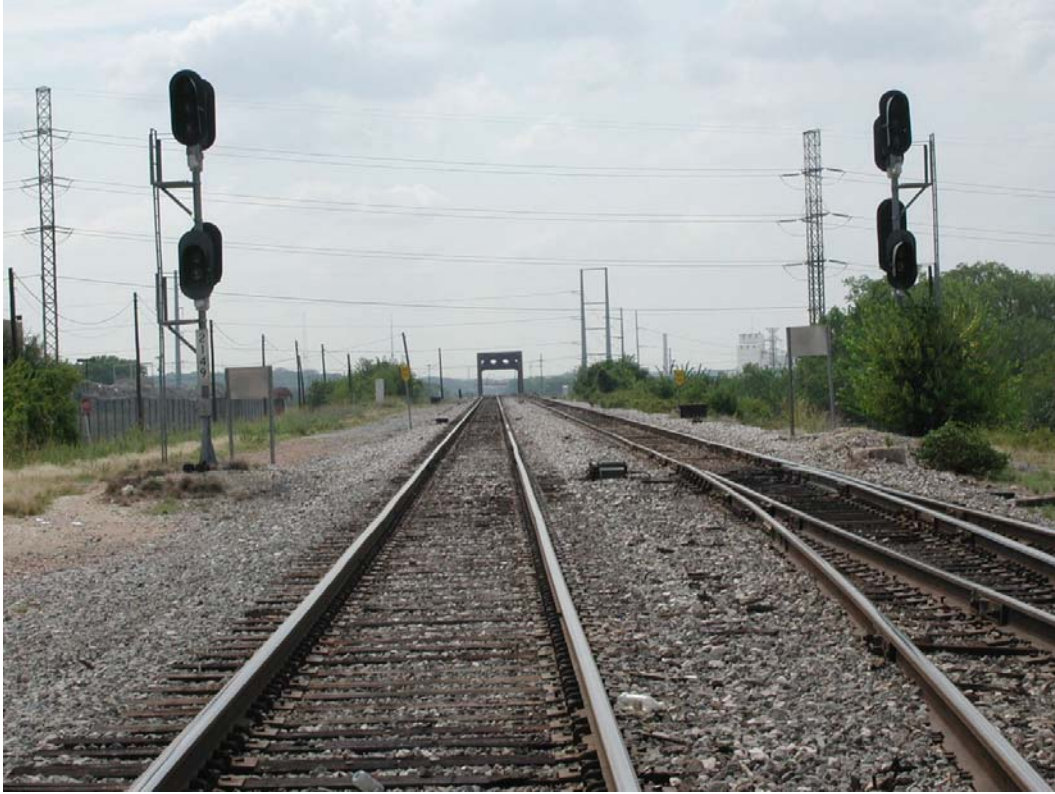
Looking West at railroad bridge elevation over Trinity River
