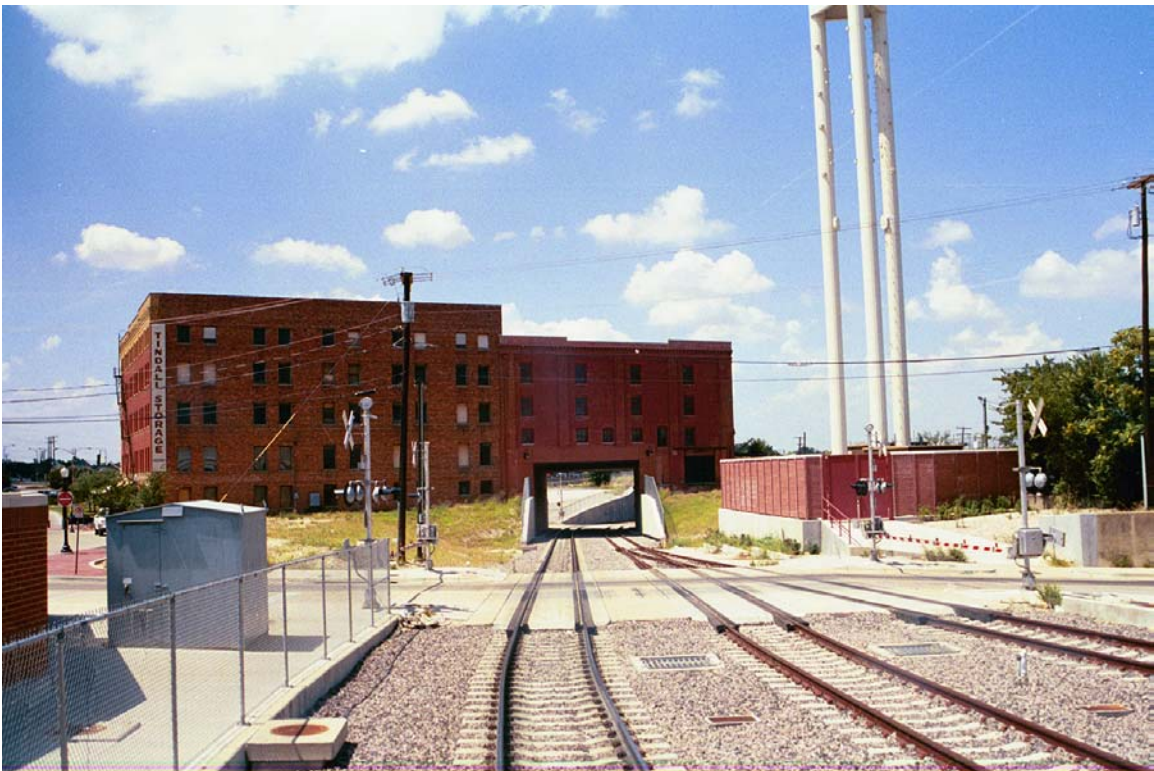
MP 611.4 9 th Street crossing Looking East
