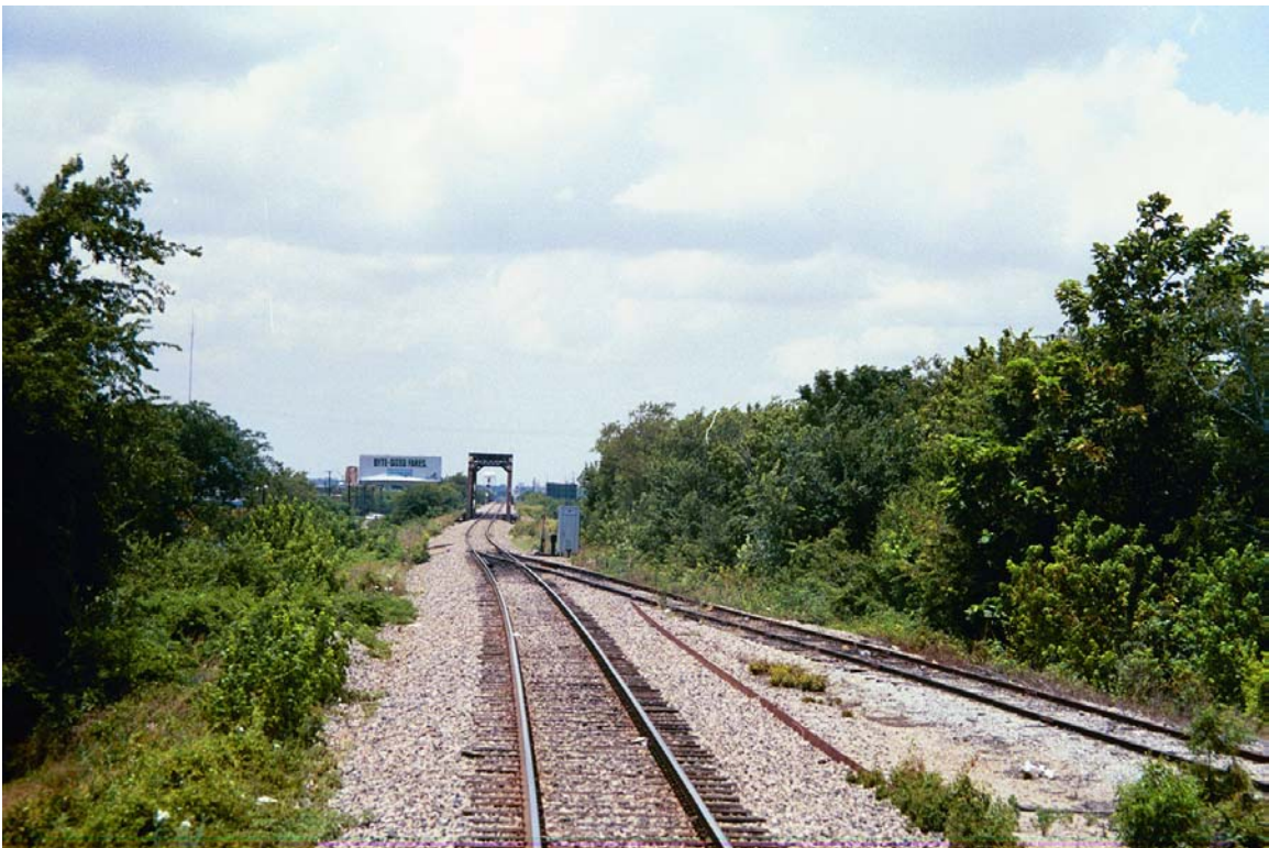
MP 640.2 Original Bridge over Old Fork of Trinity River
