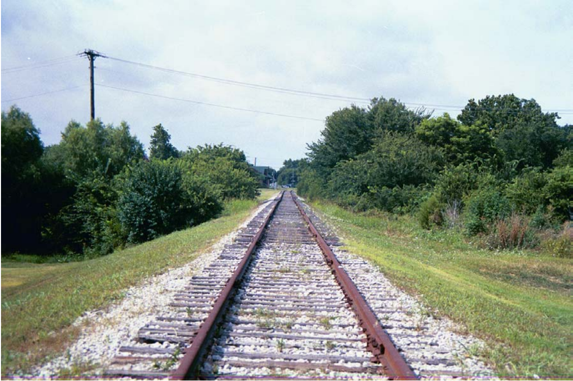
Looking South from Private crossing at Ash Street in Allen
