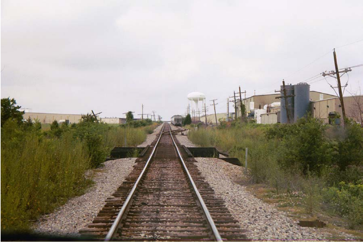
MP 794.2 North end of Armaglass siding
