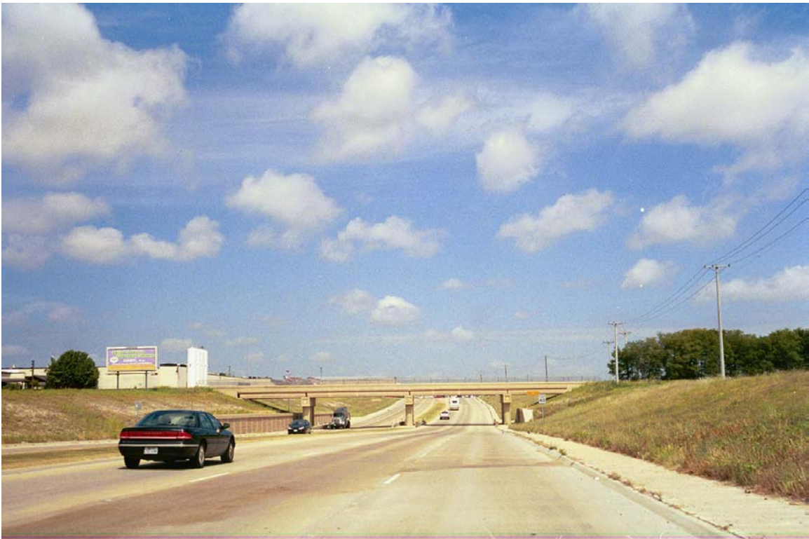
University Dr underpass Looking West, Potential end point for initial commuter rail service
