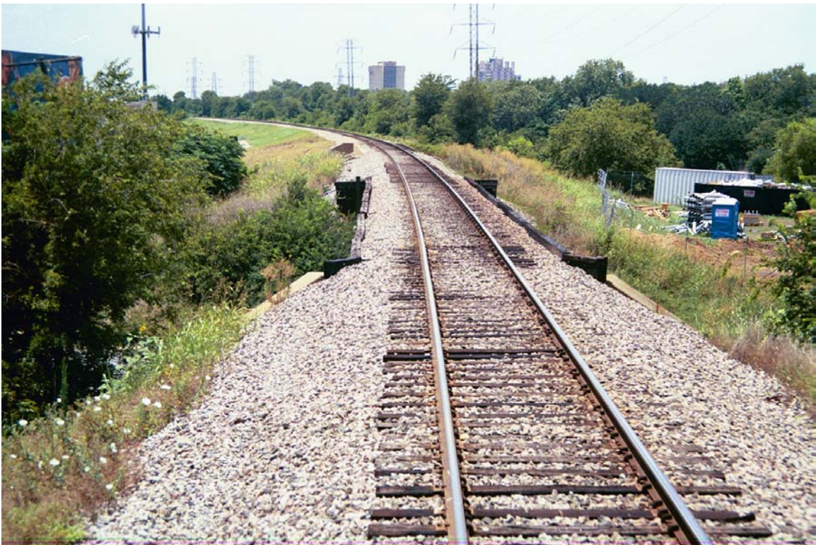
Near MP 640.4 Bridge over Inwood Road
