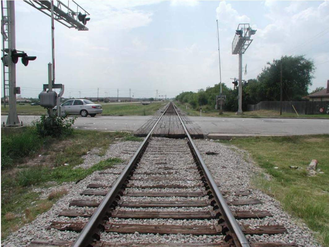
Looking West at Holiday Crossing
