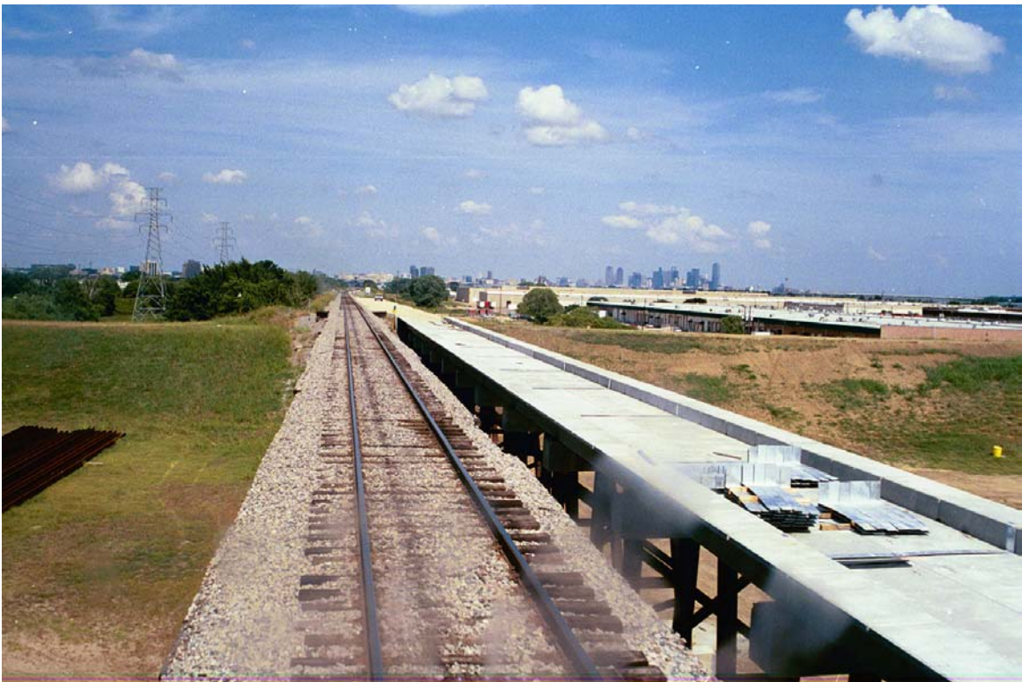
MP 637.0 New bridge over Elm Fork of Trinity River
