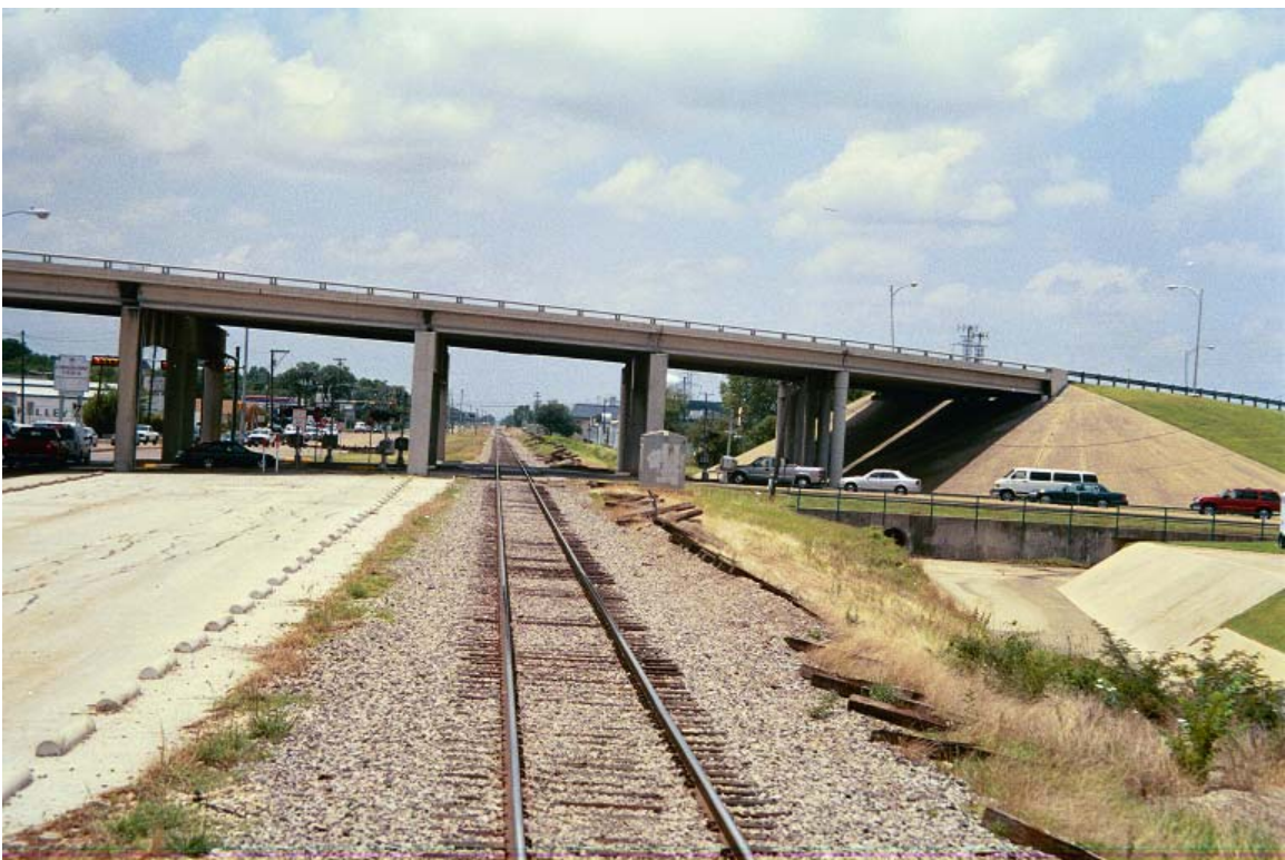
MP 633.9 HWY 356 overpass and McArthur Blvd crossing
