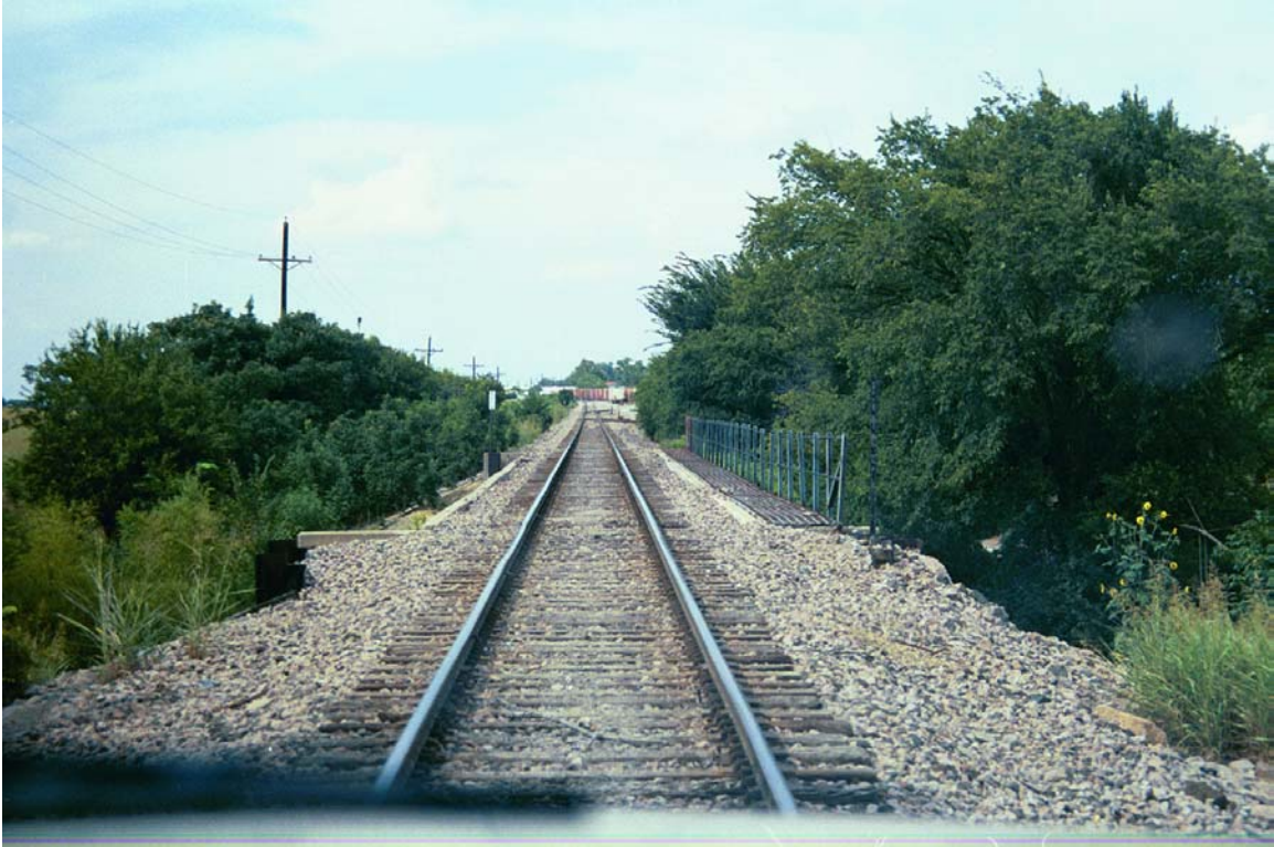
MP 686.4 Looking North at Stewart Creek Bridge
