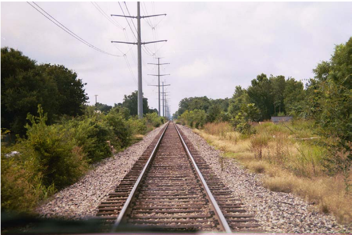
MP 773.4 HWY 12 Loop overpass in distance
