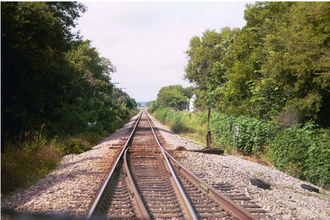
MP 781.0 South end of grain elevator spur
