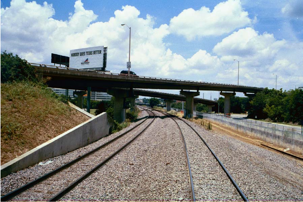
MP 642.5 Ramps are for Dallas North Tollway
