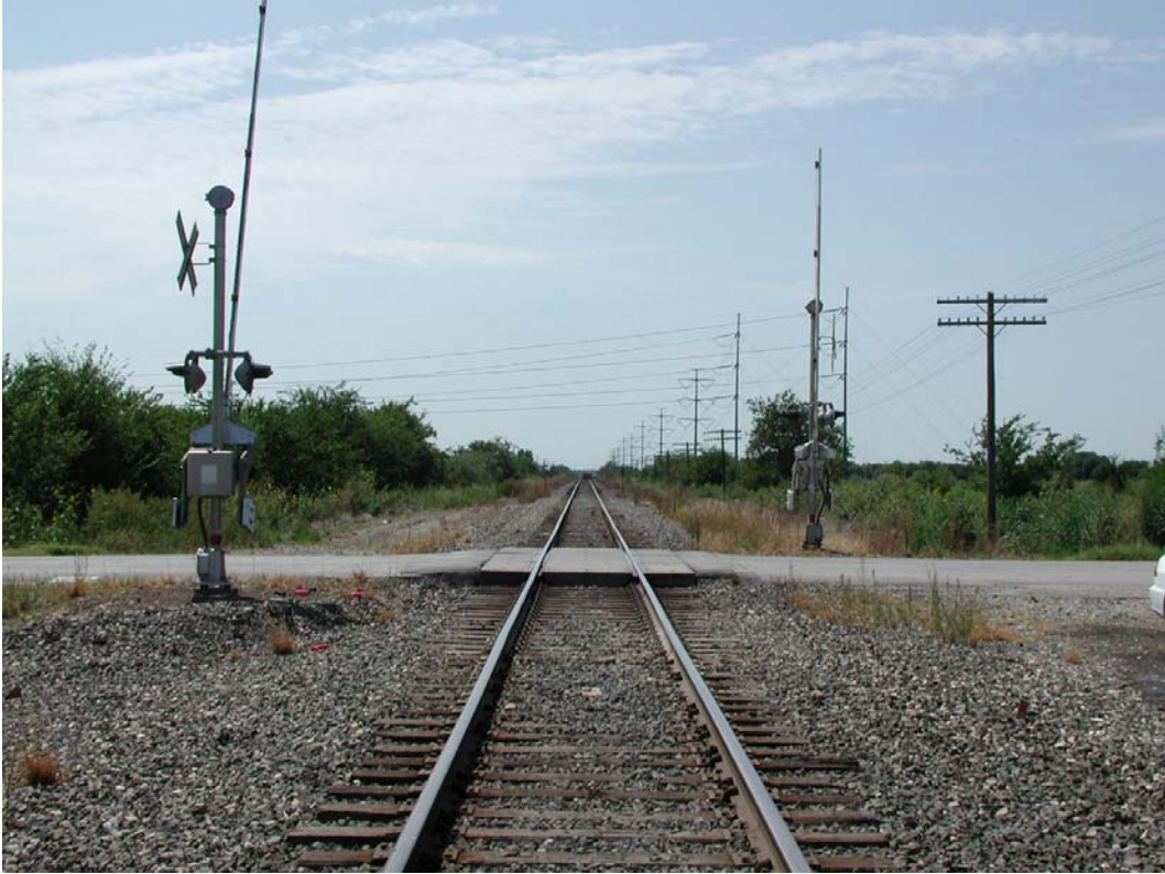
Looking South at Risinger
