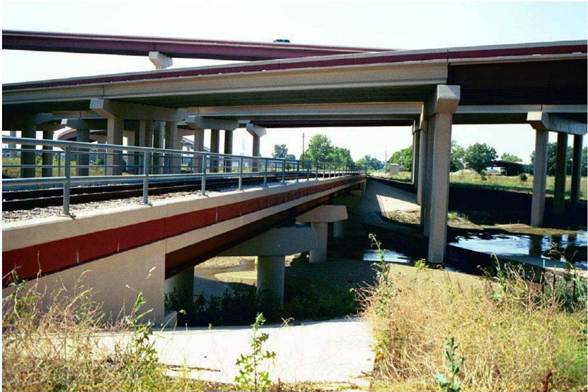
MP 742.4 – New bridge under SH-190 overpass
