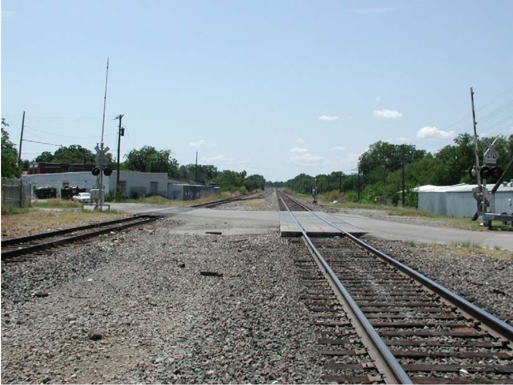
Looking South at Lipscomb
