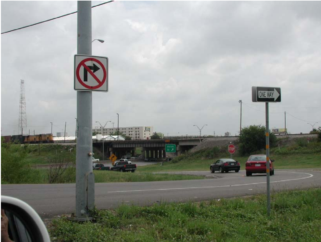
Looking South at north railroad bridge elevation at Hwy 360
