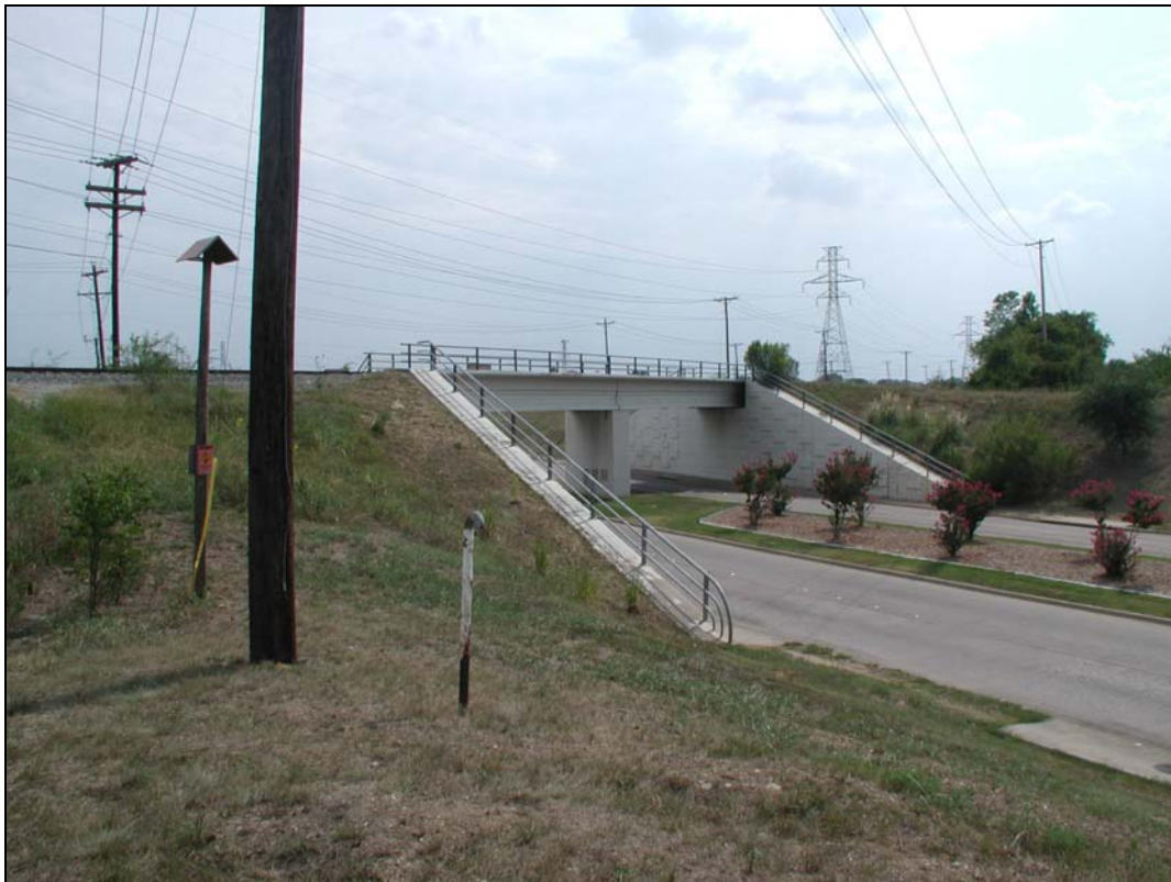
Looking southwest at Br. Over Hwy. 377
