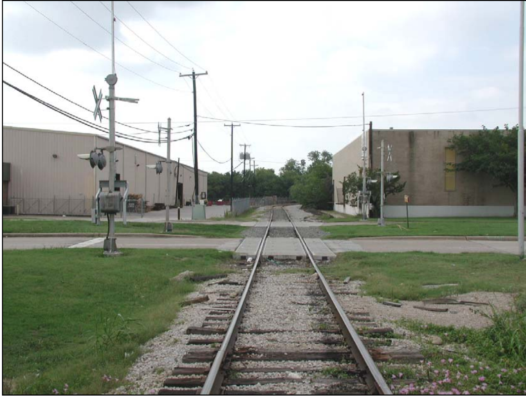
Looking south at Randol Mill Rd.
