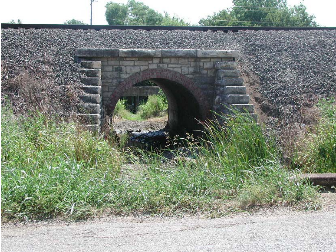
Looking at Masonry Arch bridge
