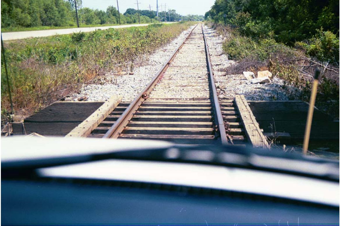
MP 738.0 – Traveling south with 60’ long bridge in foreground
