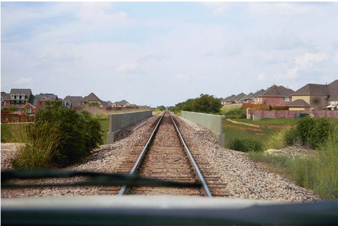
MP 688.5 Bridge over County Rd
