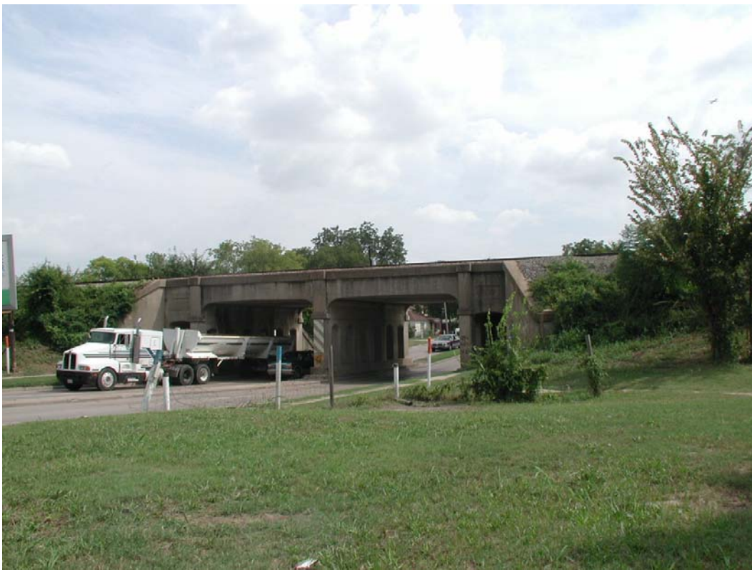
Looking South at north railroad bridge elevation over Sylvan
