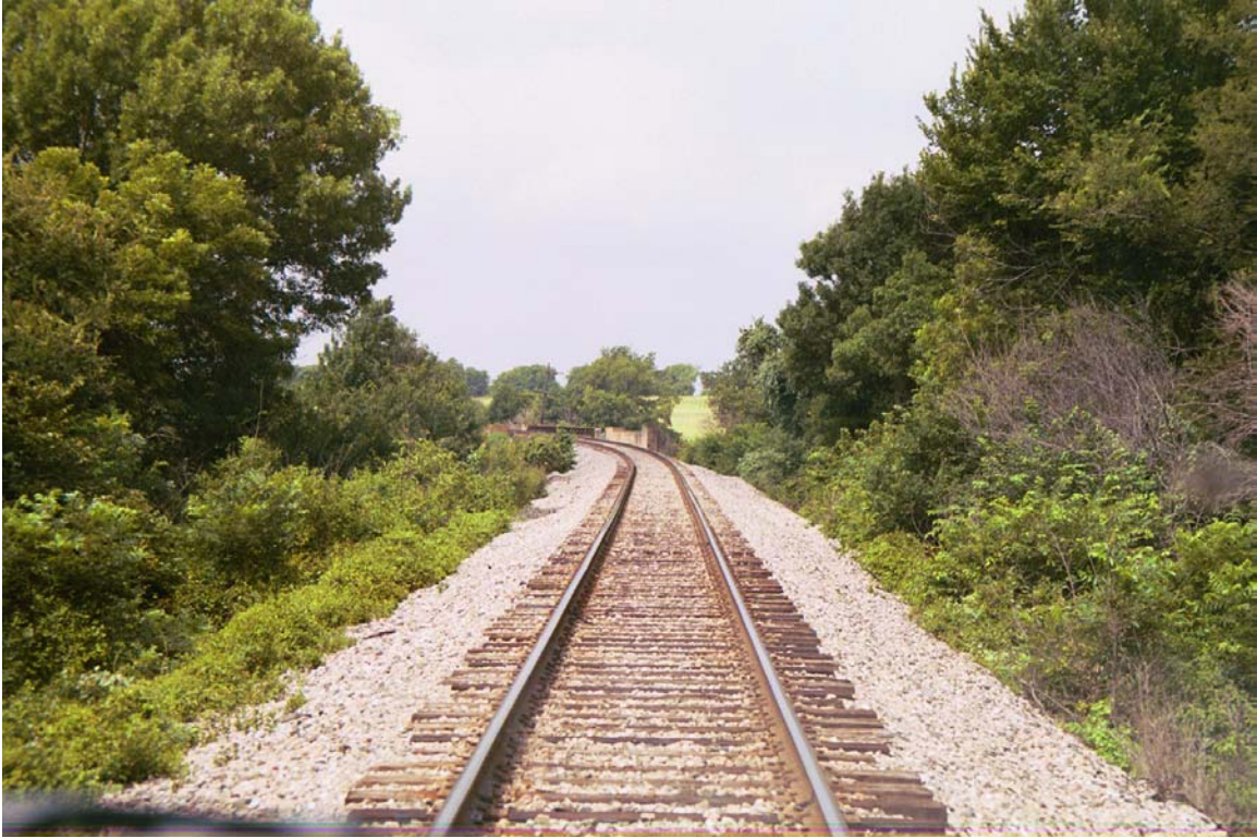
MP 789.8 with bridge over HWY 77 in distance
