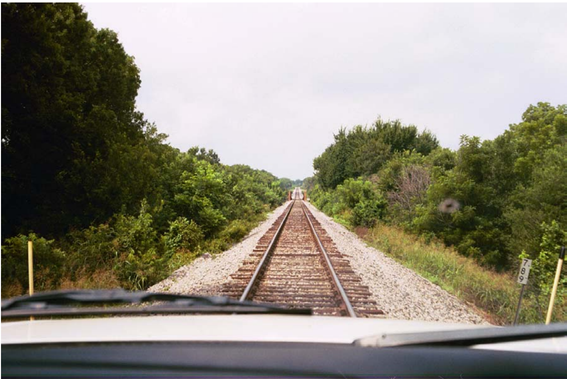
MP 789.0 Red Oak Creek bridge in distance
