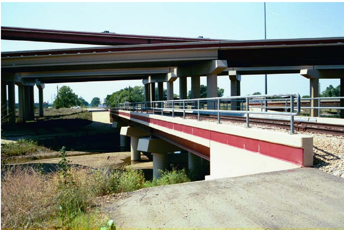
MP 742.4 - New bridge under SH-190 overpass
