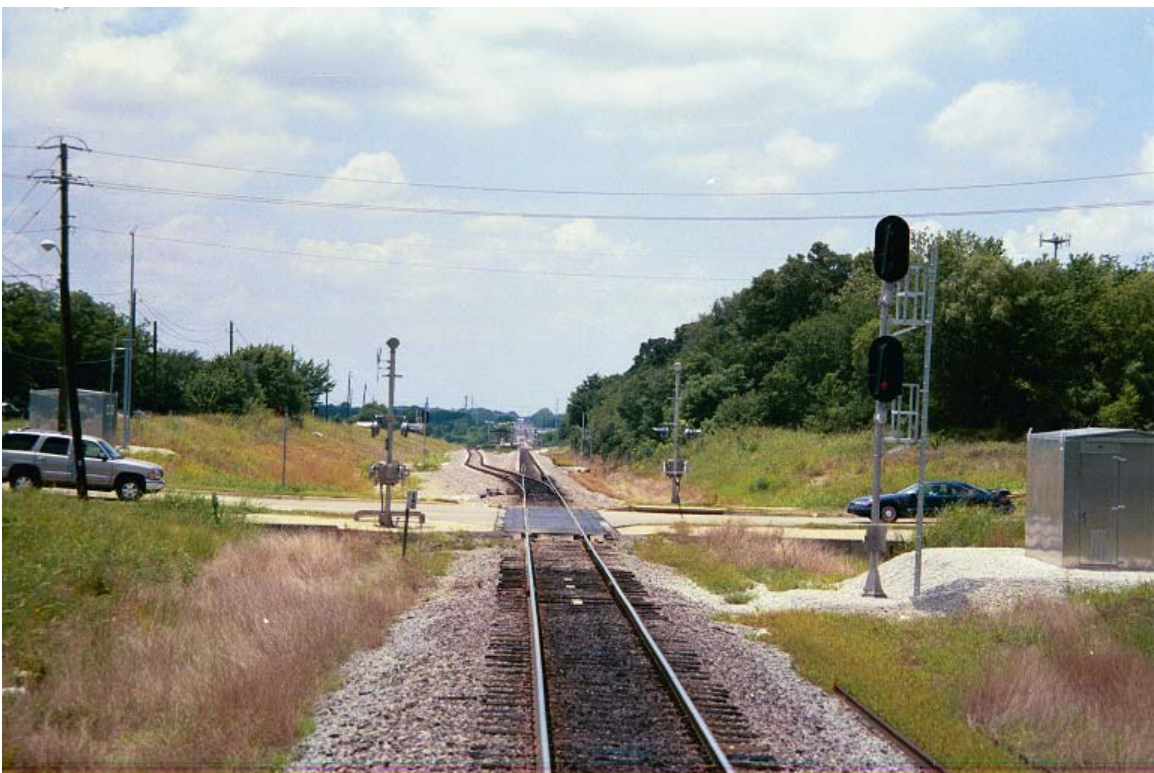
MP 631.5 Gilbert Rd crossing
