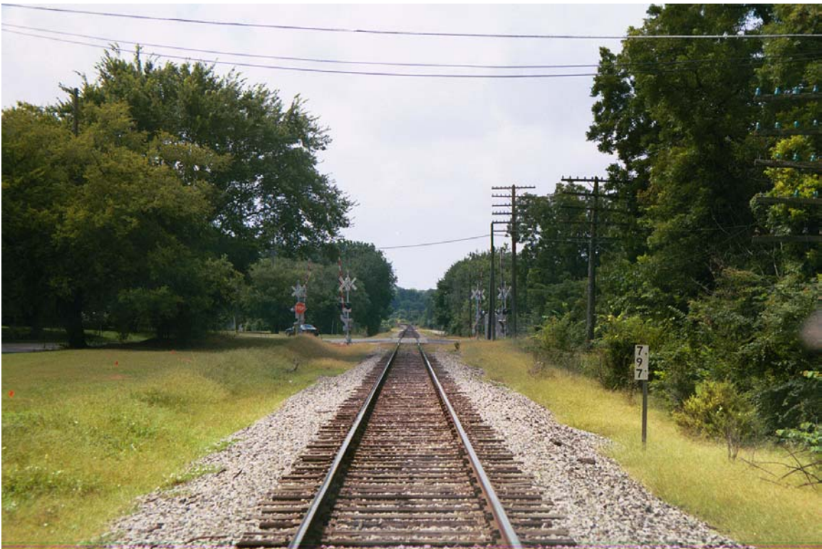
MP 797.0 East Main (HWY 287) crossing
