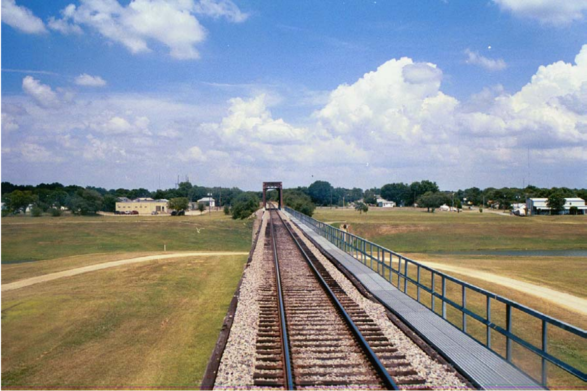
MP 612.4 Trinity River Bridge Looking East
