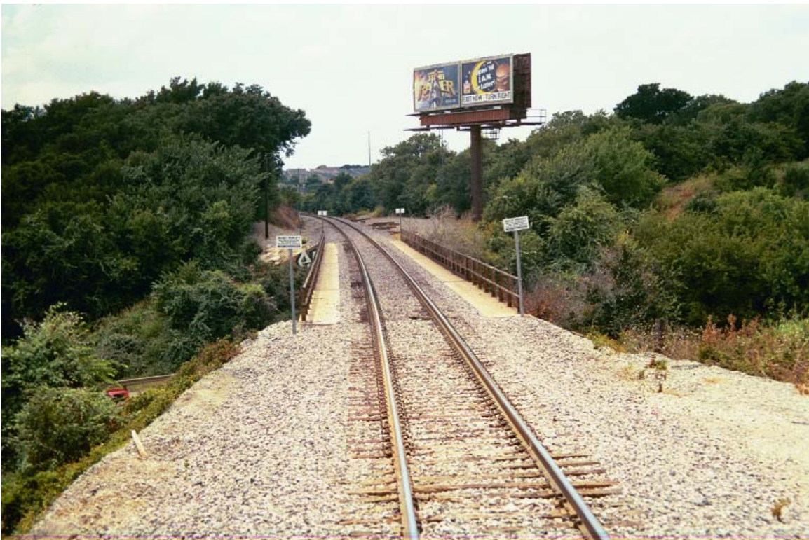
MP 628.2 HWY 360 Underpass
