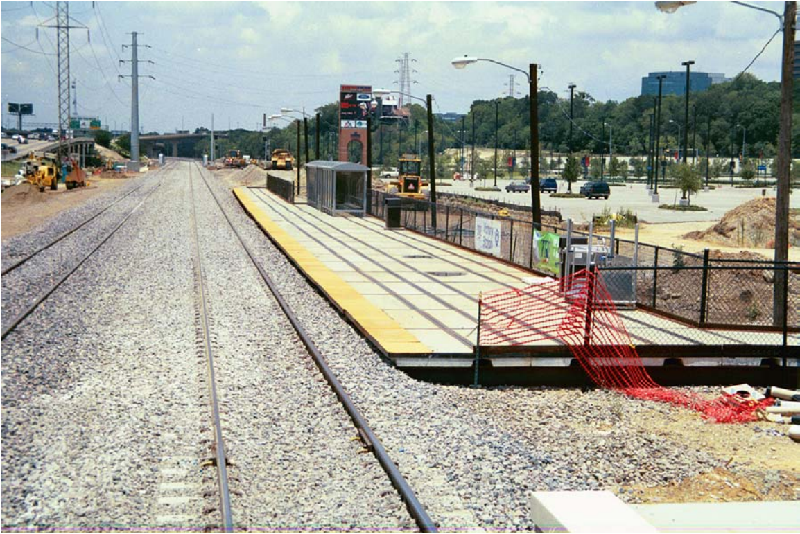
MP 642.7 Temporary Victory Station
