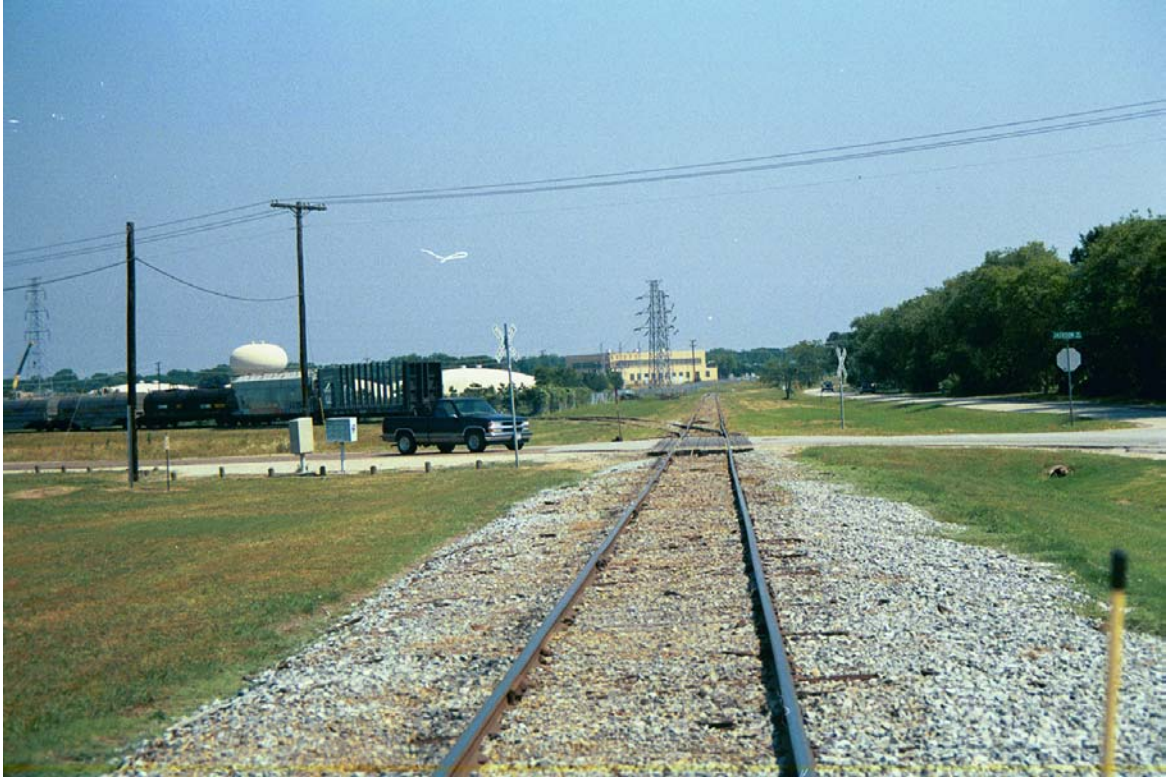
MP 742.9 – Jackson Road with spur track to Elm Fork Water Treatment Plant and Deseret Grain.
