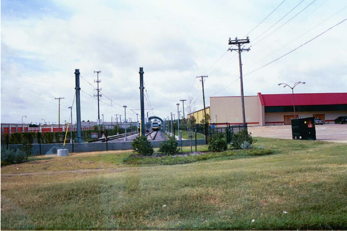
Plano Looking South at end of DART LRT from Parker Rd
