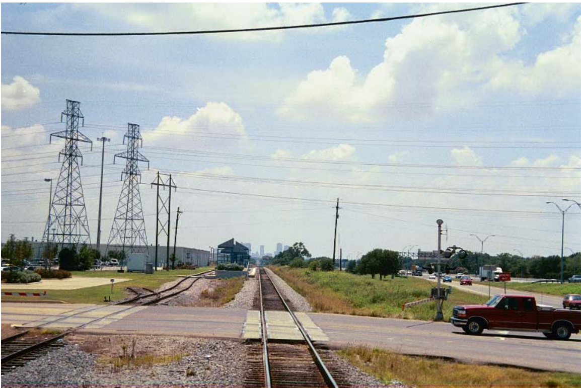
MP 618.5 Richland Hills Station and Handley Ederville crossing
