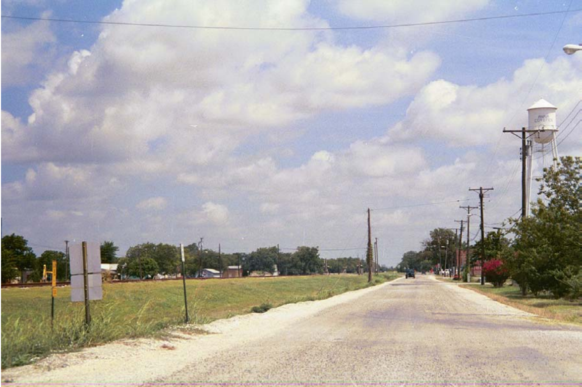
Looking north at 4 th St crossing in distance in Anna
