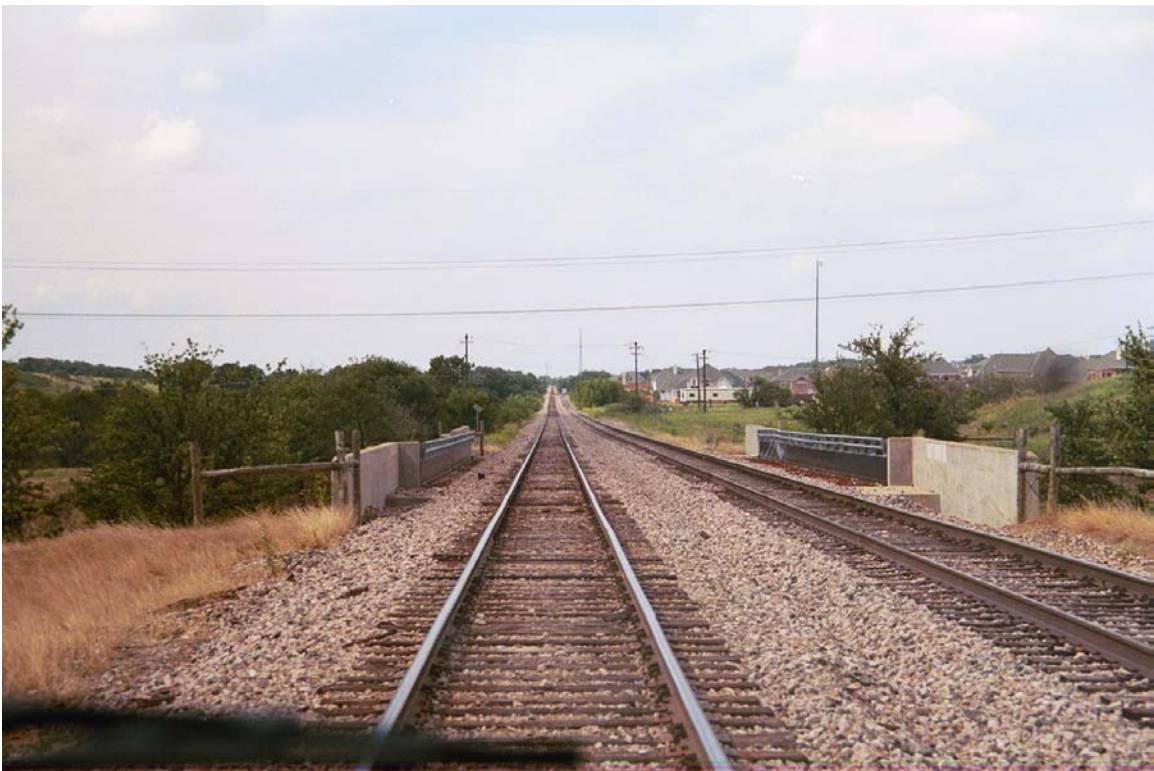
MP 692.5 over Windhaven Parkway
