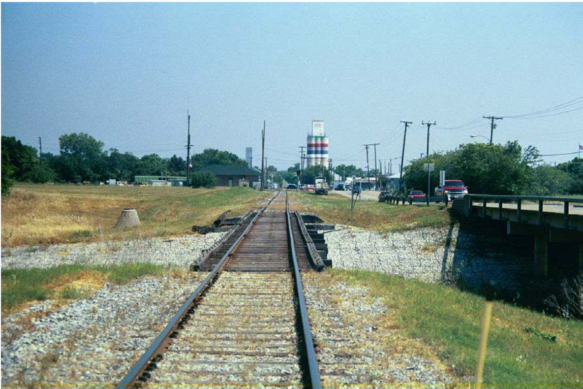
MP 744.4 – Bridge in Carrollton is 130 feet in length
