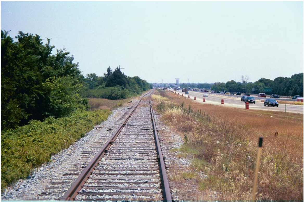
MP 731.3 Looking south with I-35E, Stemmons Freeway at right
