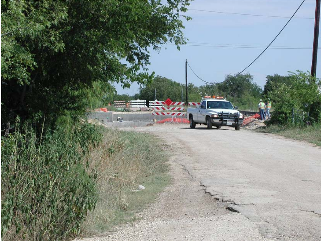
Construction of bridge over railroad at Hampton
