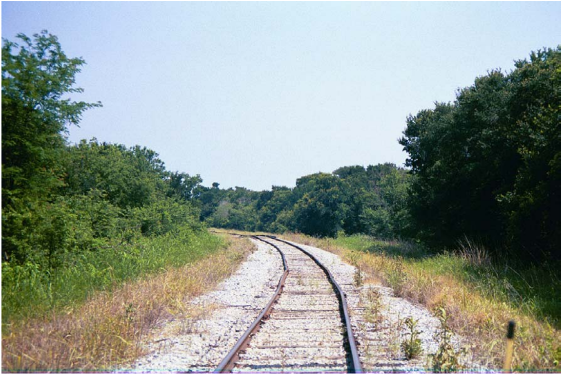
MP 740.5 – South of SH-121. Note poor track condition.
