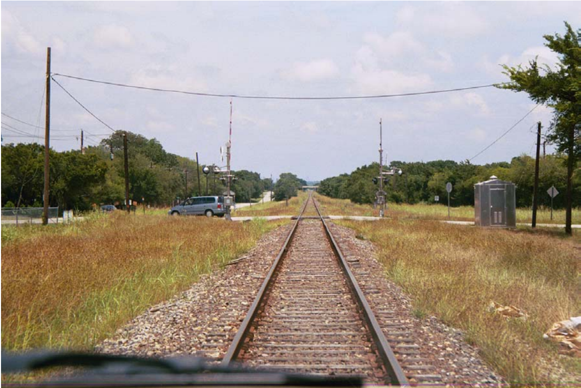
MP 35.4 New crossing between Wilfy St and FM 1382 overpass
