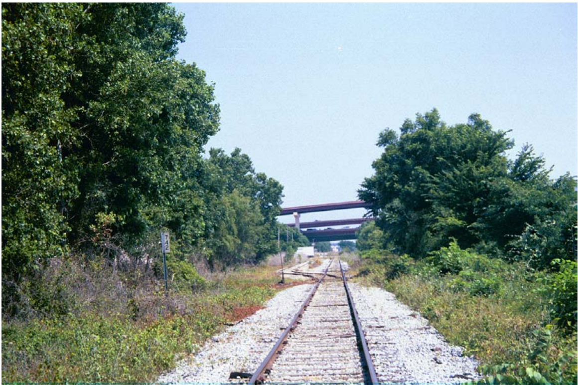
MP 742.1 – Siding and spur track to Vanguard with SH-190 in distance.
