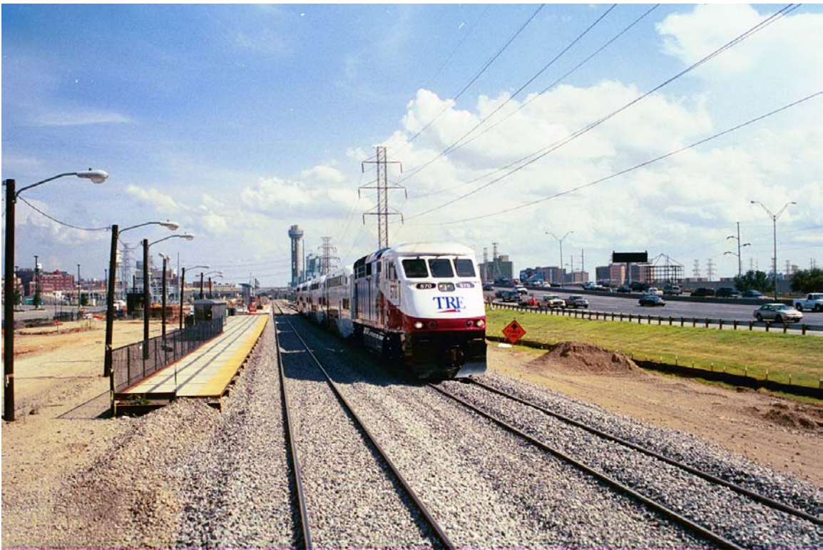
MP 642.7 Temporary Victory Station
