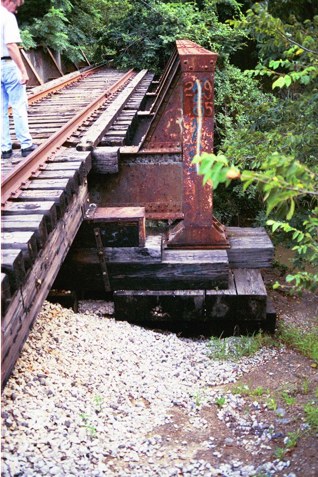
Bridge at Cottonwood Creek Looking North
