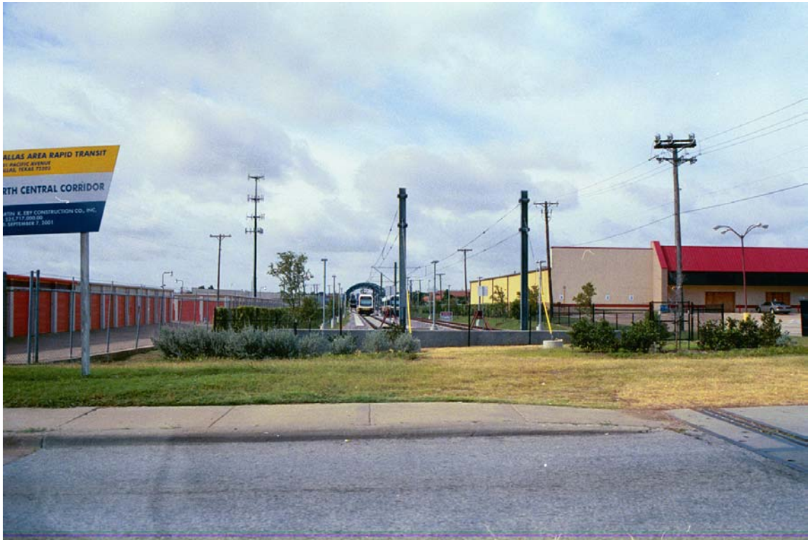
Plano Looking south at end of LRT at Parker Rd
