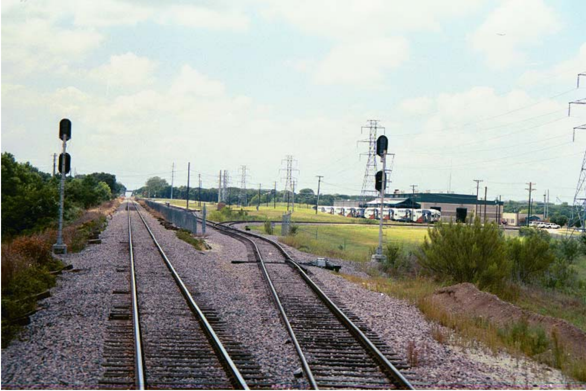
MP 630.6 East end of TRE Irving Yard
