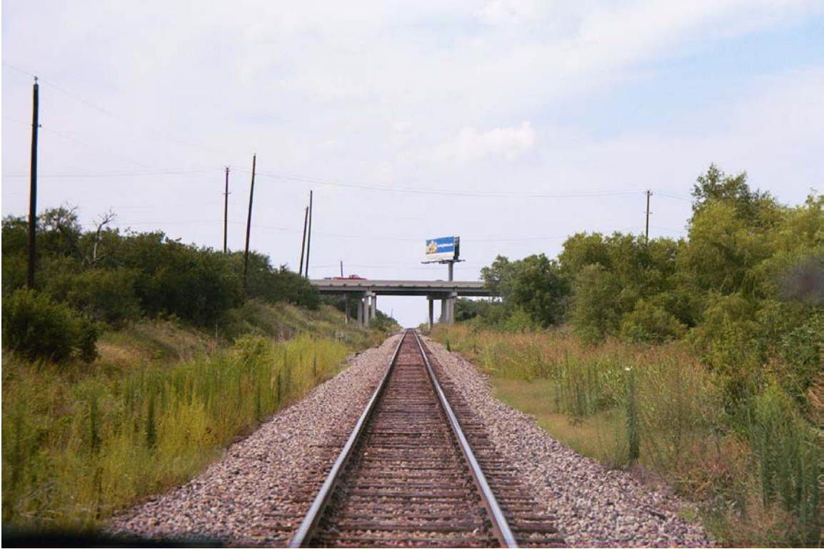
MP 690.9 HWY 121 Overpass
