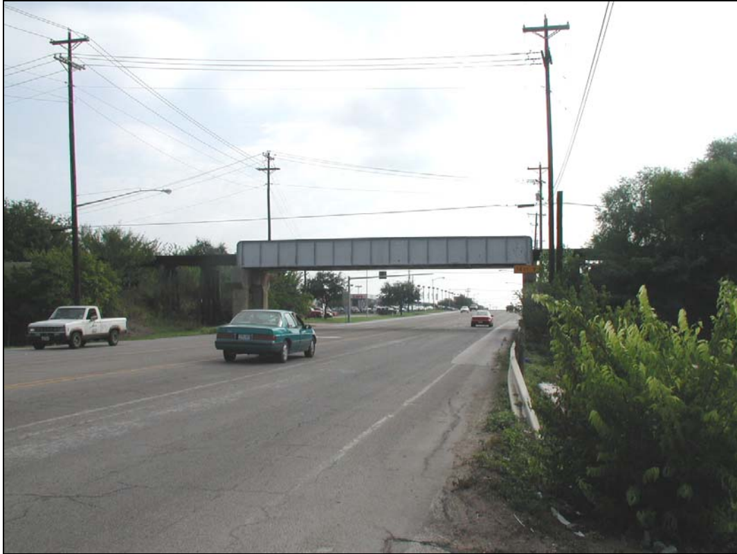
Looking east at railroad bridge over Division St. E
