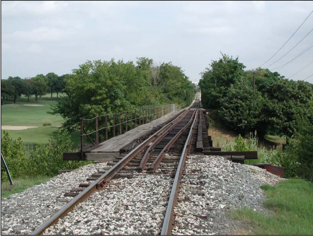
Looking north at railroad bridge over Johnson Creek
