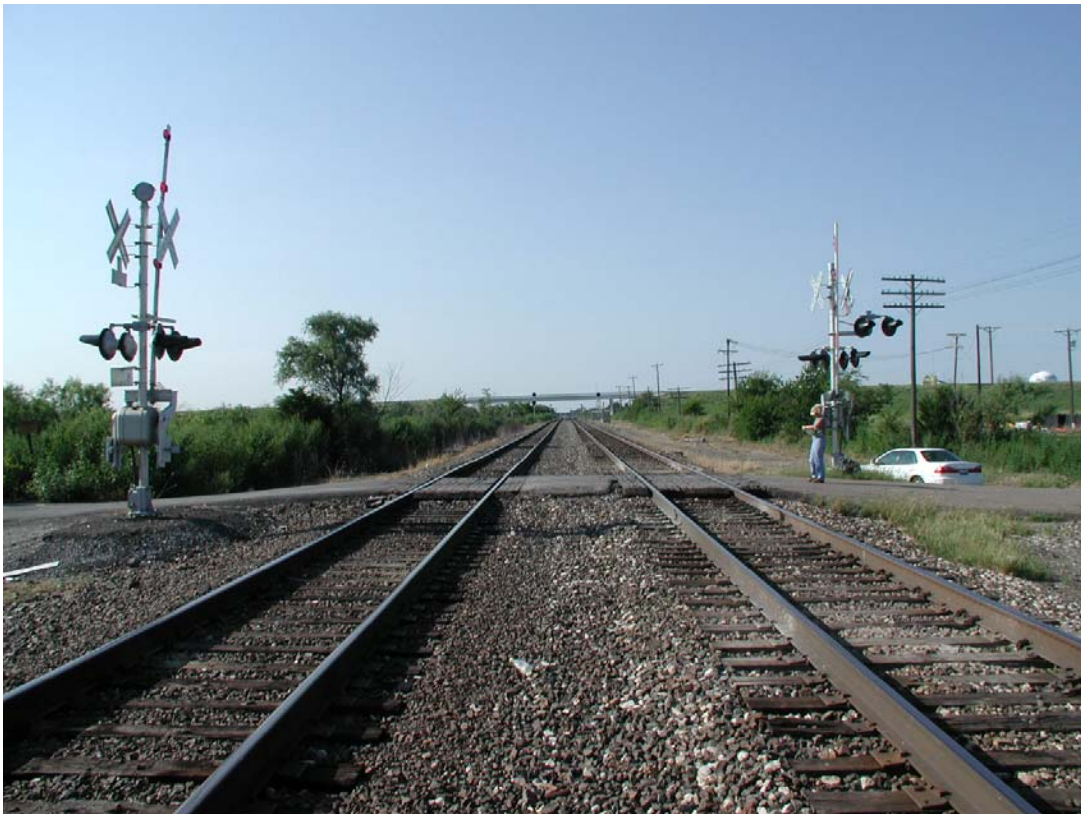
Looking West at CR700
