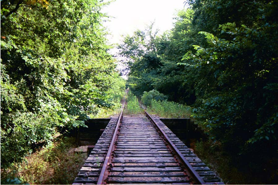
Cottonwood Creek Bridge Looking North
