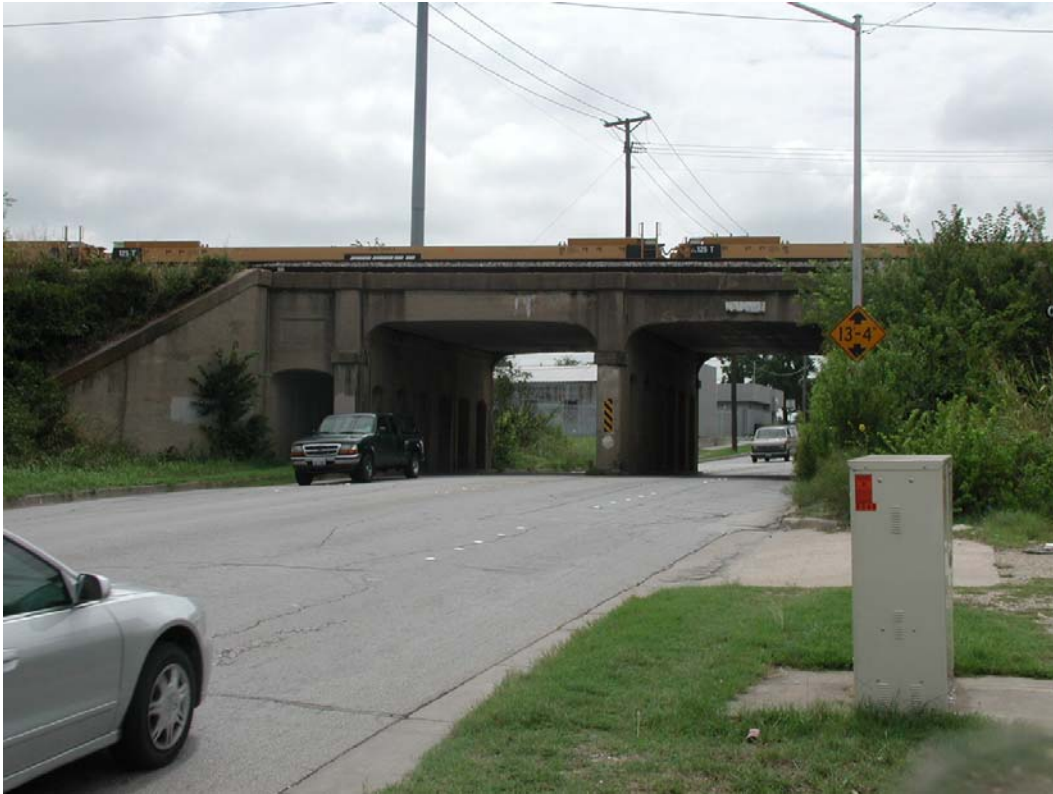
Looking South at north railroad bridge elevation on Riverside Dr.
