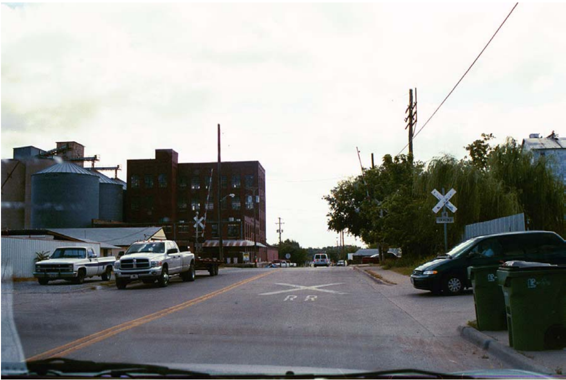
Louisiana St crossing Looking North
