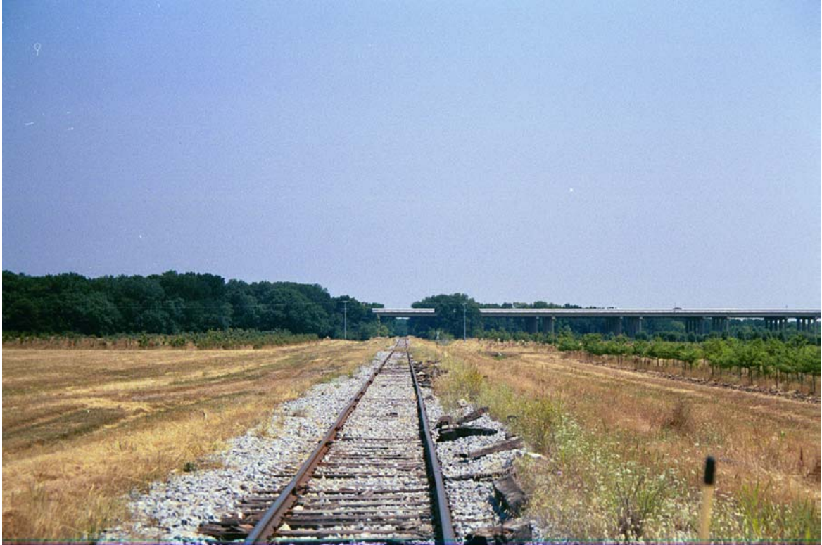
MP 740.1 – Looking south at SH-121 / Vista Ridge overpass in distance
