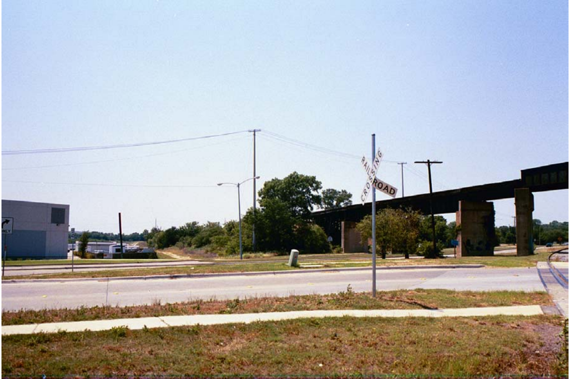
MP 735.6 – Looking northwest at KCS Bridge with Cowan Street in foreground
