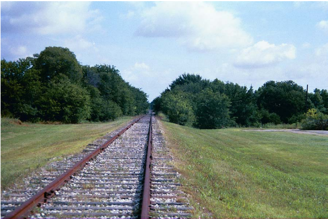
Looking North from private crossing at Ash Street in Allen
