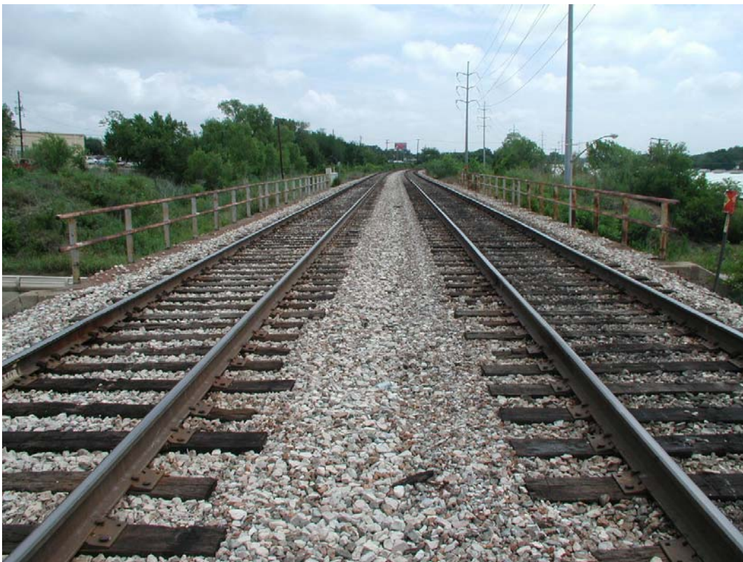
Looking NE at railroad bridge over Beach St.
