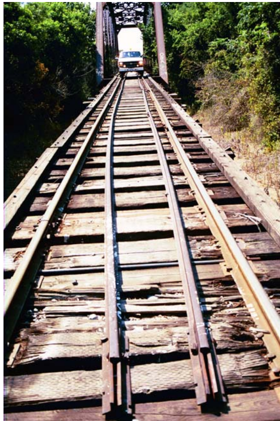
MP 741.1 south end of Trinity River Bridge, looking north
