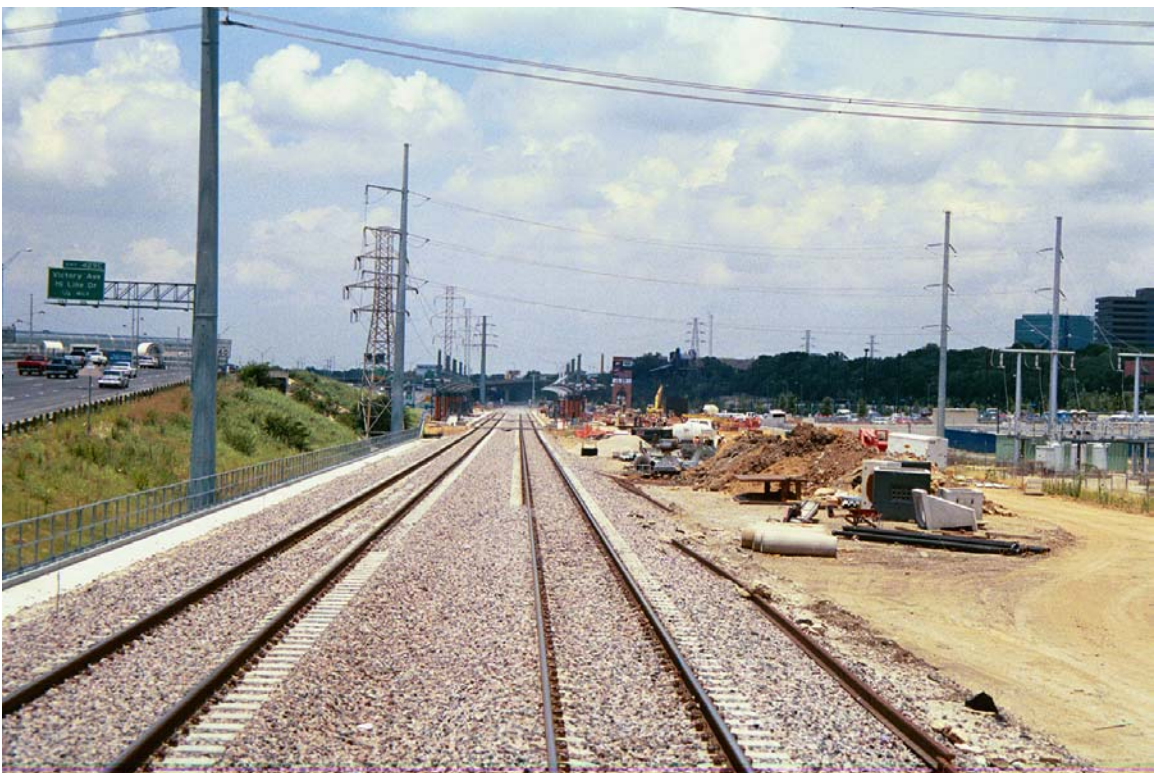
New Arena Station under construction in distance
