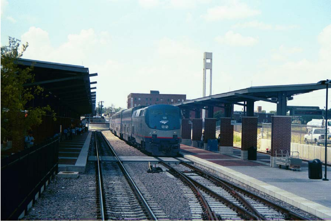
MP 611.4 ITC Station In fort Worth Looking East
