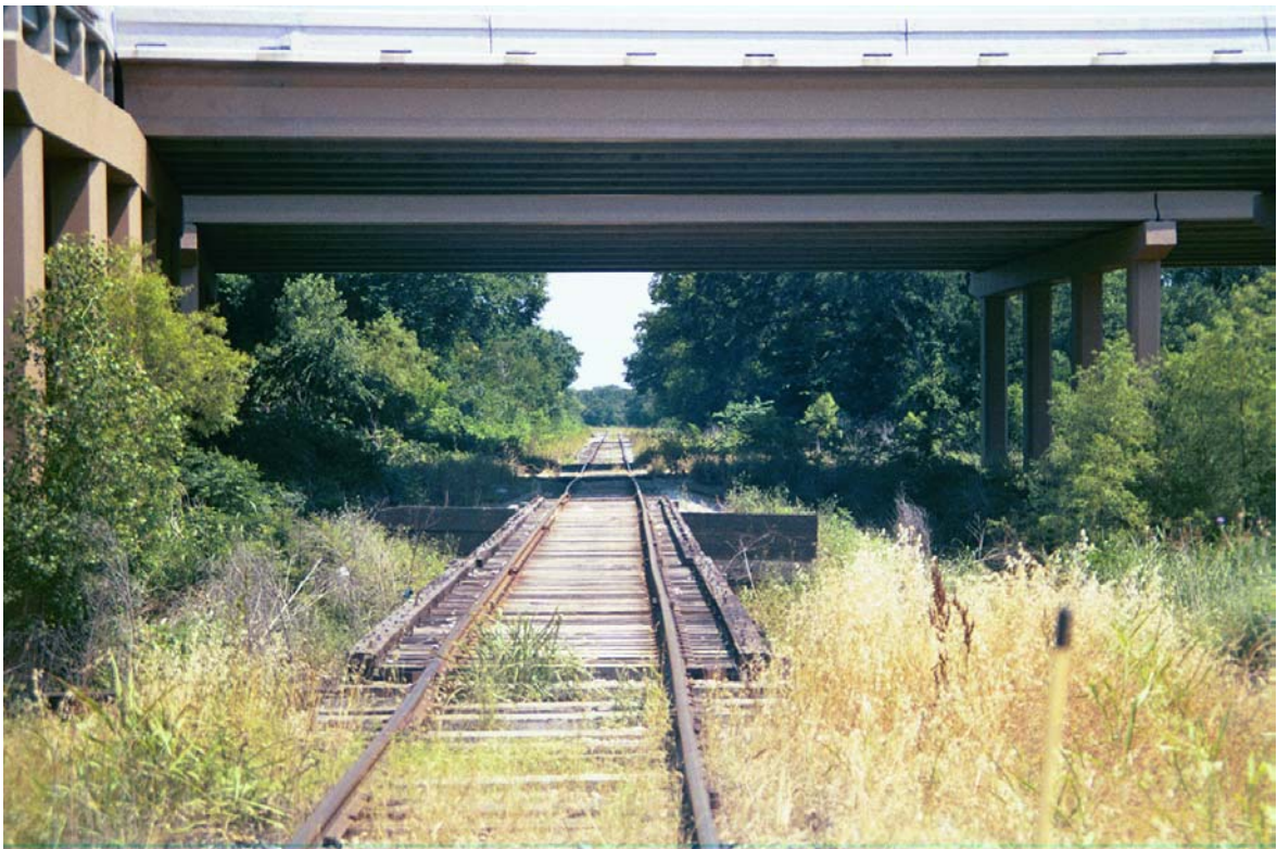
MP 740.2 – SH-121 overpass with 117' long bridge in foreground
