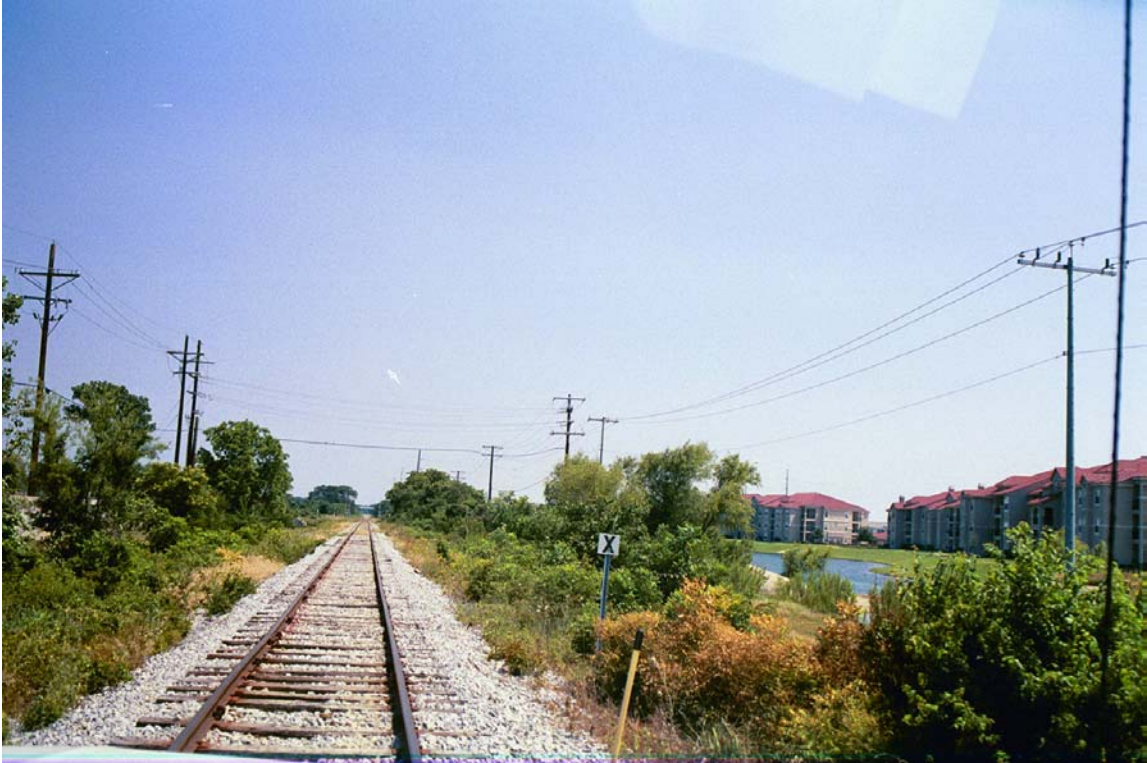
MP 739.2 – Looking south approximately one-half-mile north of Hebron Parkway with apartments at right
