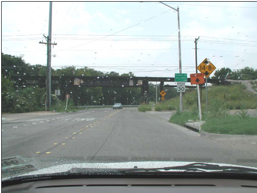
Looking East at Railroad Bridge over Trail Lake Dr.
