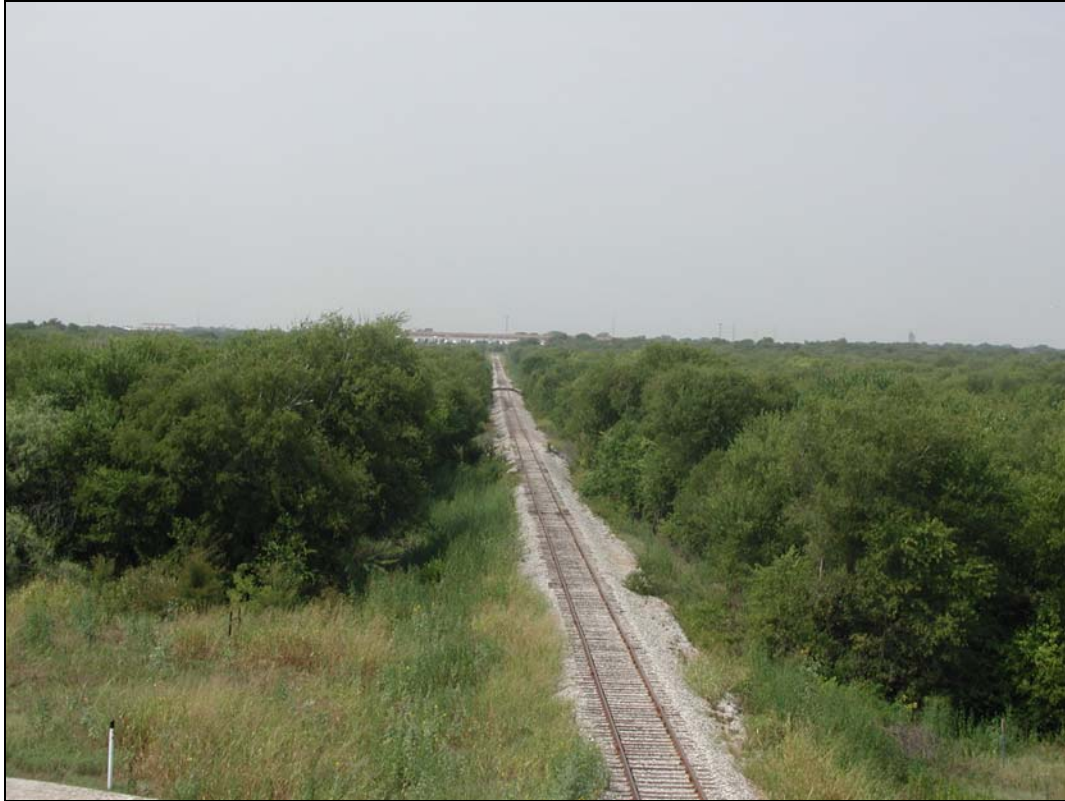
Looking East from Hwy. 121 Bridge
