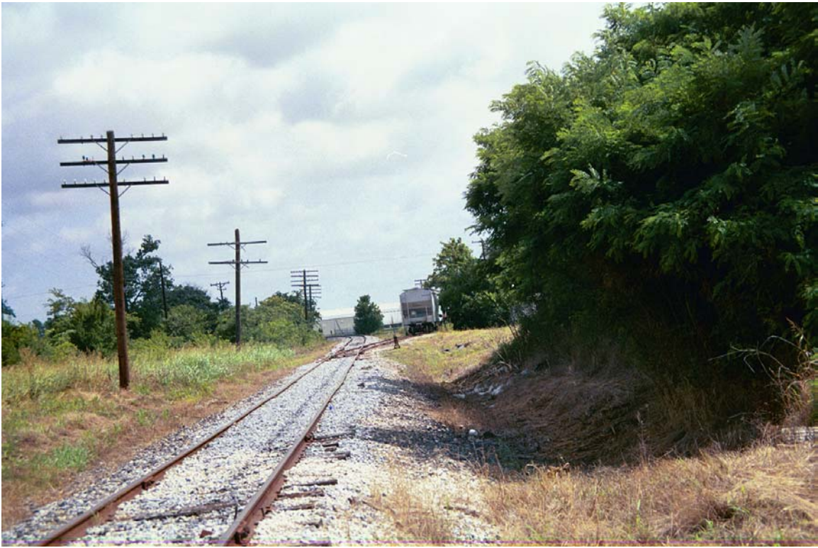
Looking north from Industrial Blvd.
