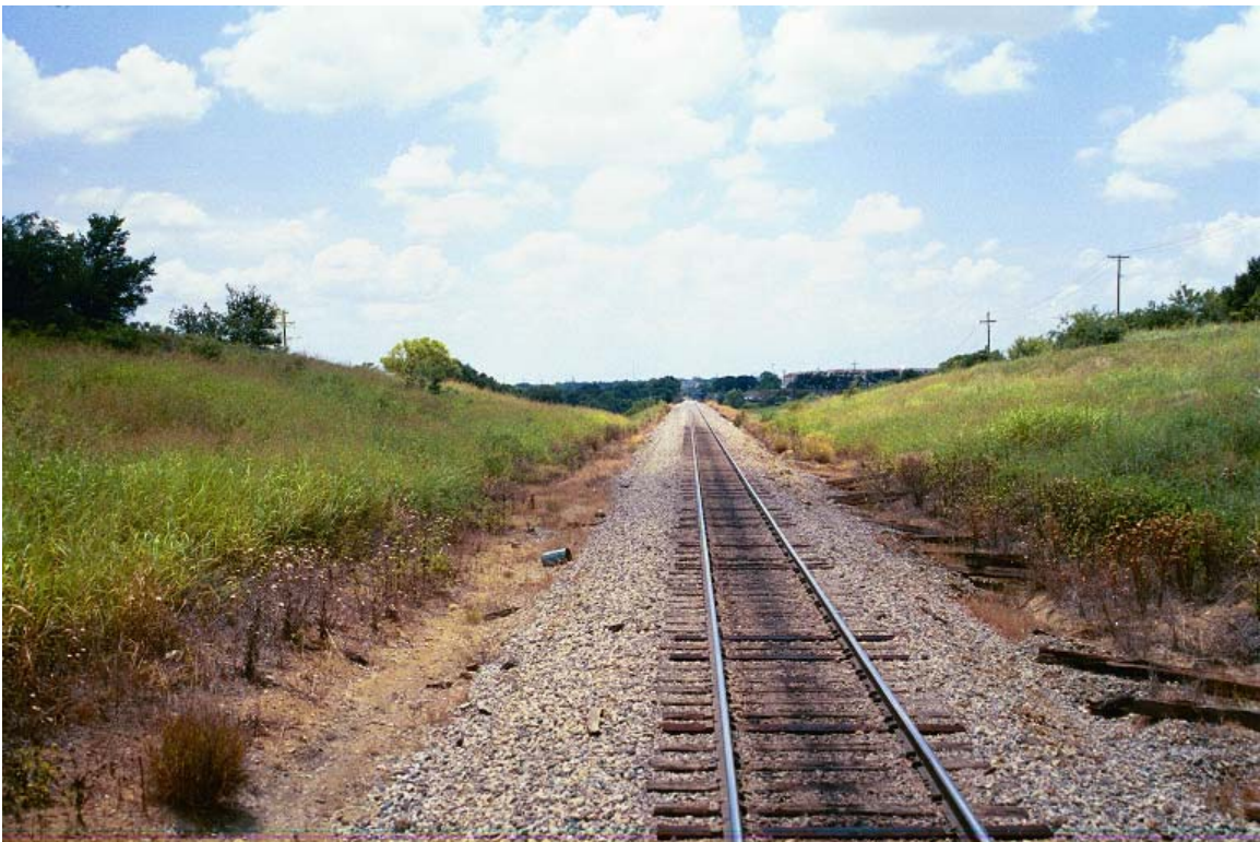
Near MP 629 Dorothy Sink (10 MPH speed limit) fill over removed trestle
