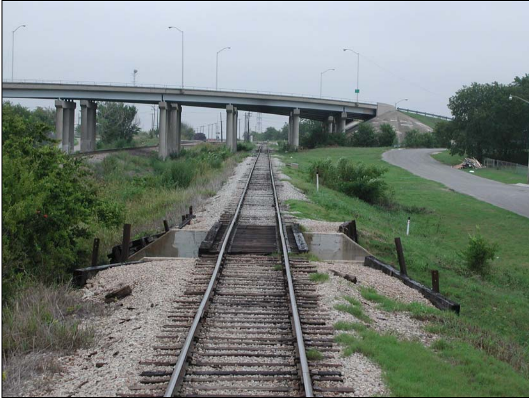
Railroad Bridge west of Long Avenue
