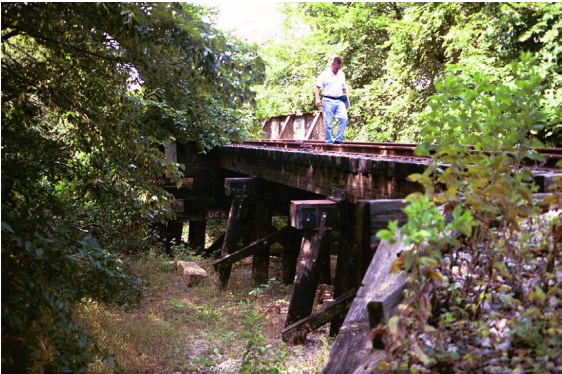
Cottonwood Creek Bridge Looking South
