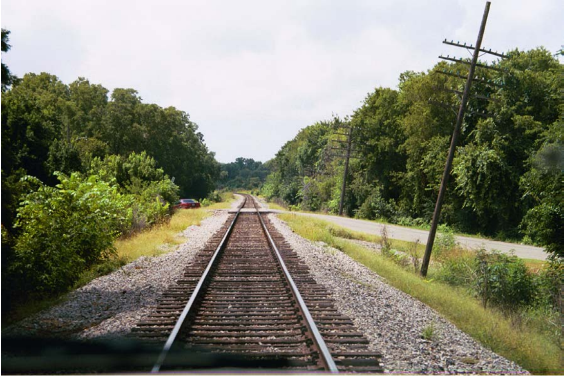
MP 797.2 East Jefferson crossing
