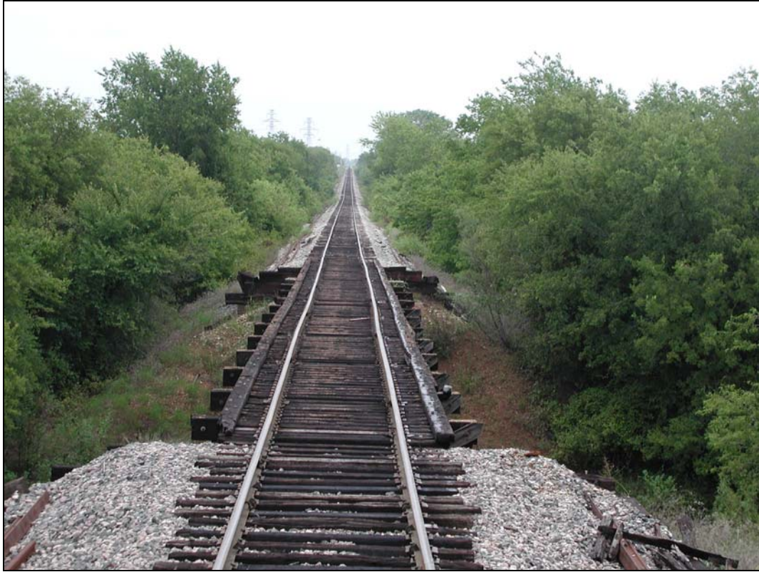
Looking east at Little Fossil Creek Bridge (West Track Crossing)
