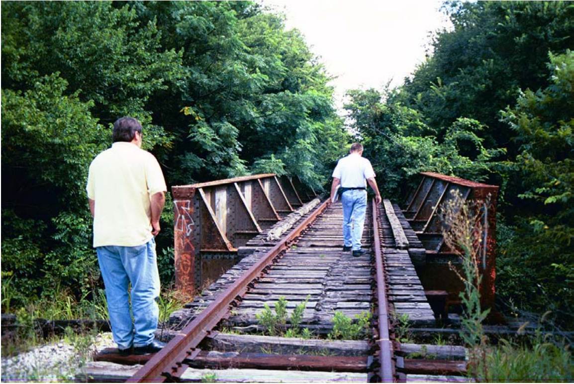
Bridge at Cottonwood Creek looking North
