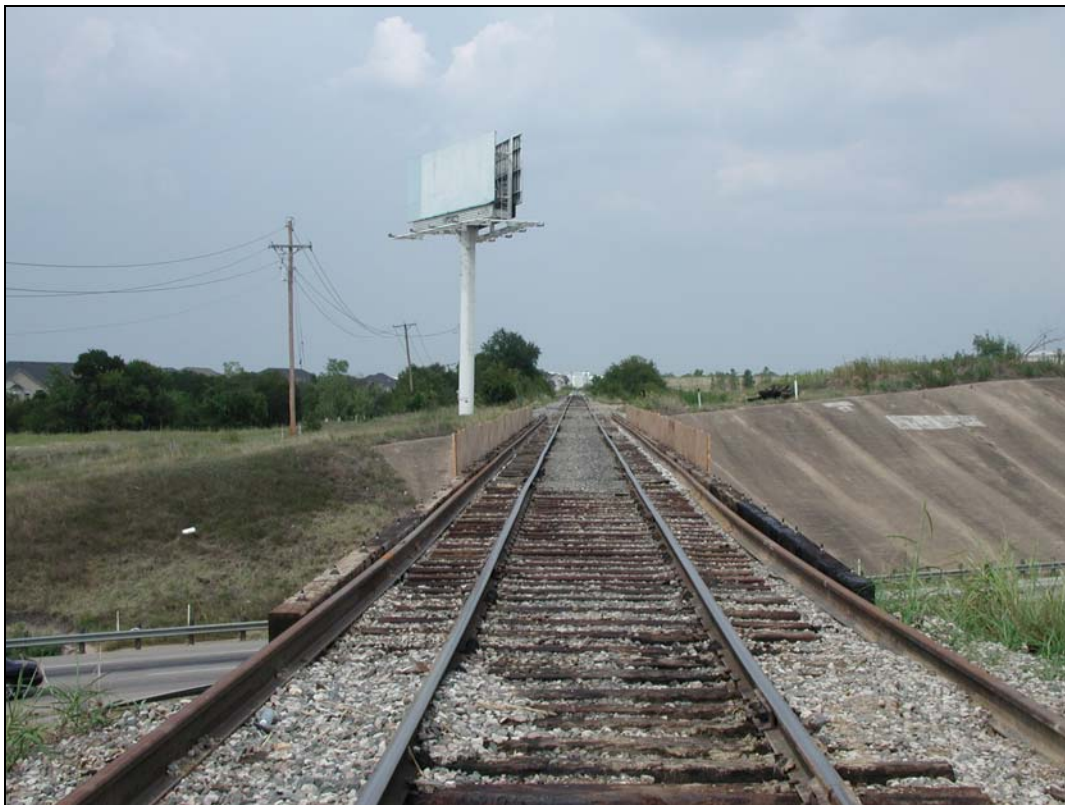
Looking south at Loop 820 Railroad Overpass
