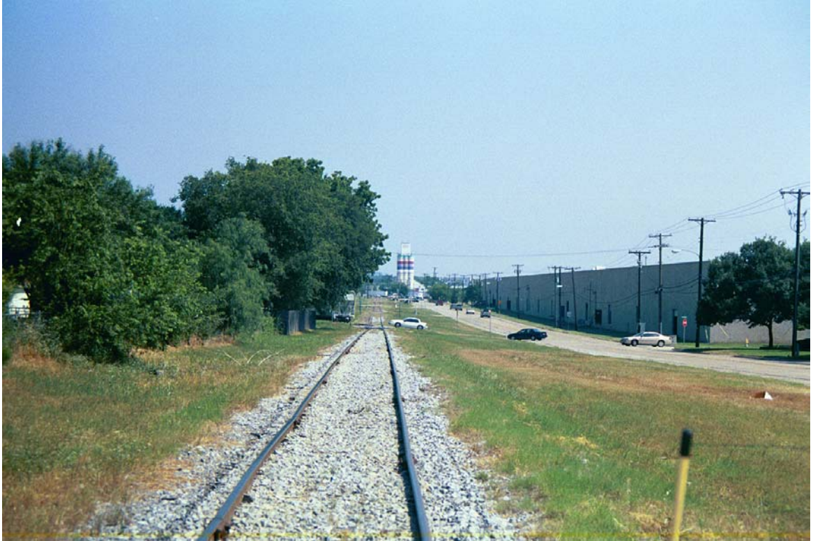
MP 744.2 – Northside Drive and spur track to Vinylex Plastics
