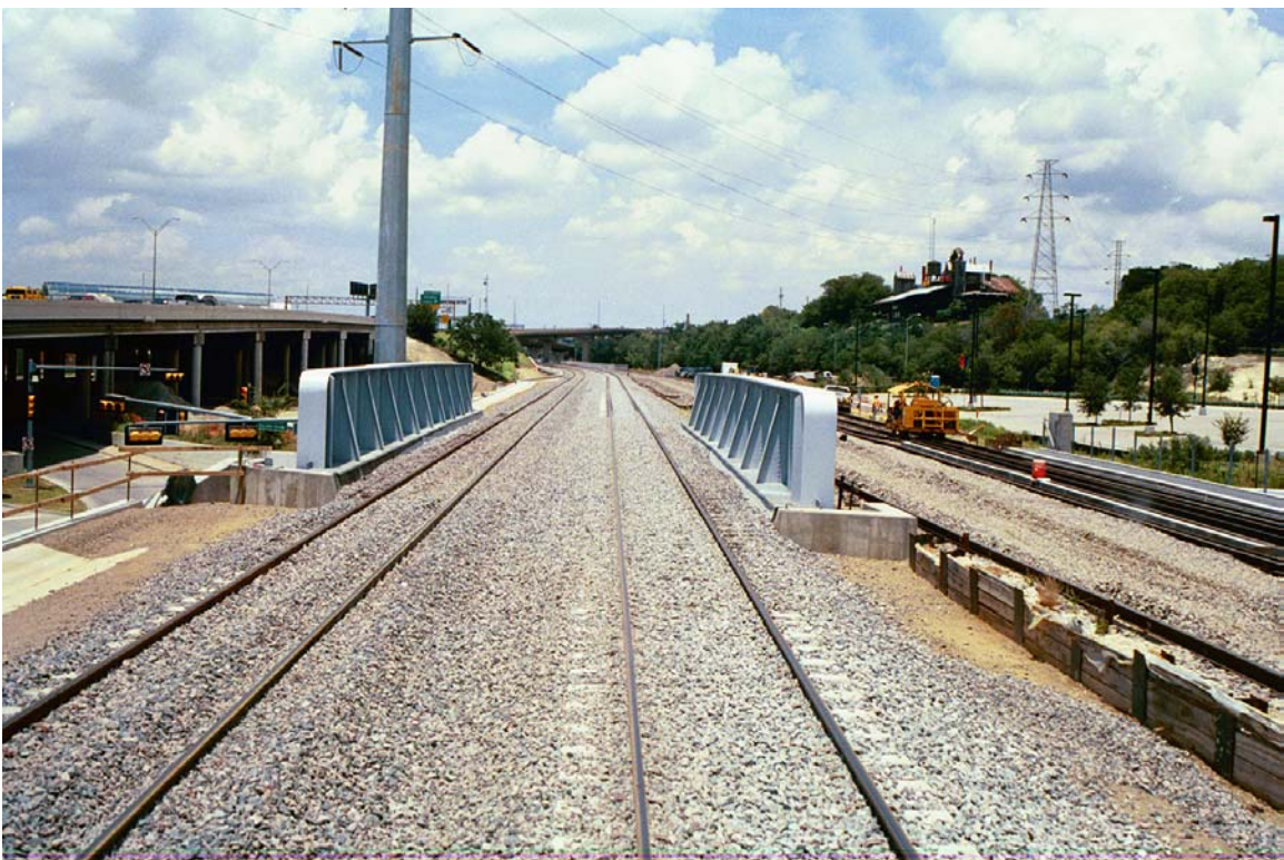
MP 642.6 bridge at Dallas Jct.
