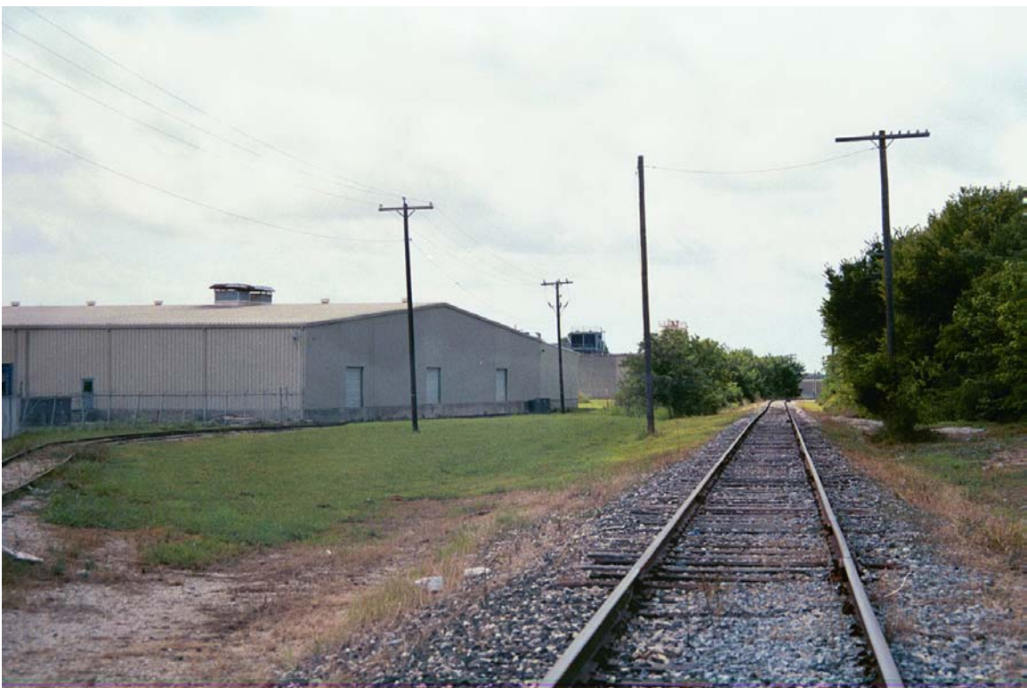
Looking South from Elm in McKinney
