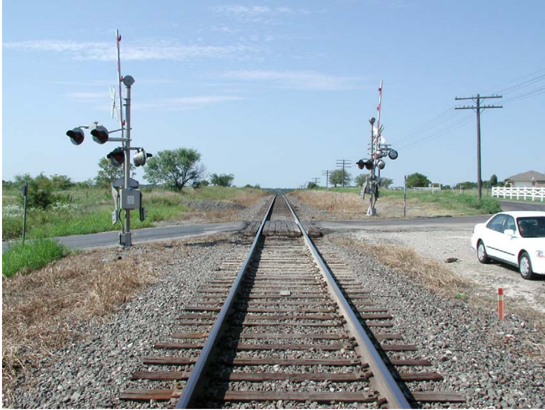
Looking South at CR1021
