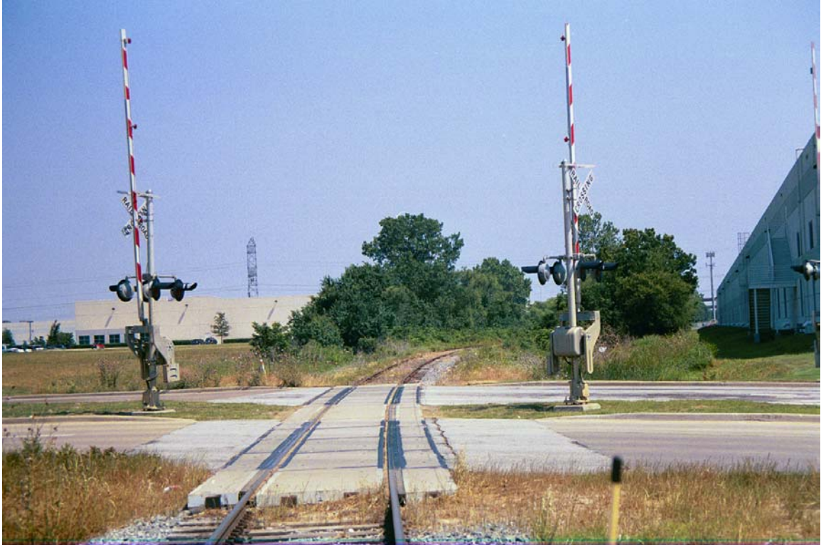
MP 741.8 – Frankfort Road crossing looking south.
