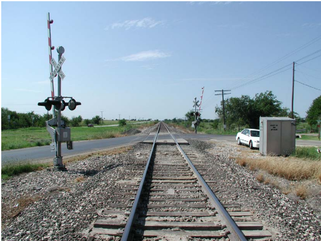
Looking South at CR1016
