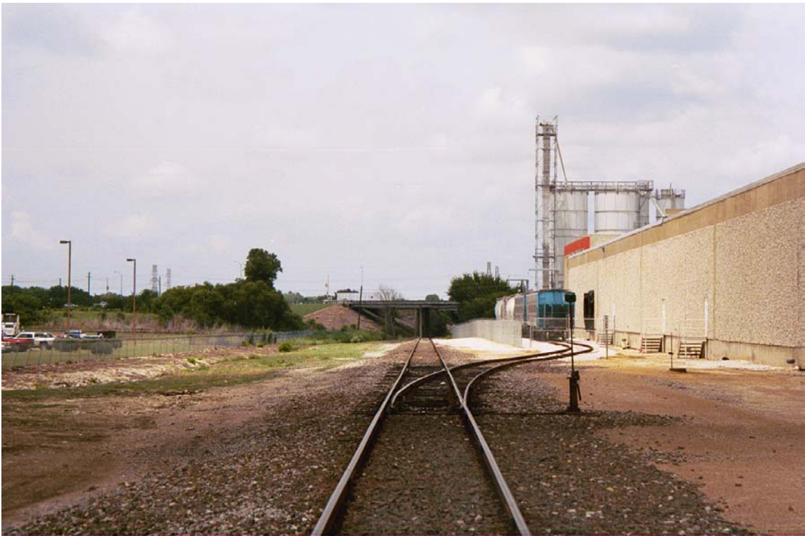
MP 43.4 Frito Lay Plant at Maglab, HWY Loop 12 overpass in distance
