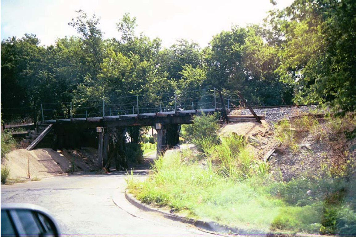
Broad St Looking NE Under railroad
