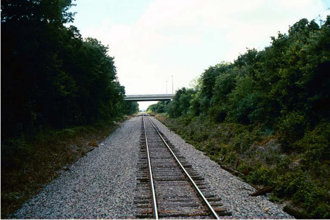
Near MP 629.5 new Trinity Rd Overpass is approximate Dallas/Tarrant County Line
