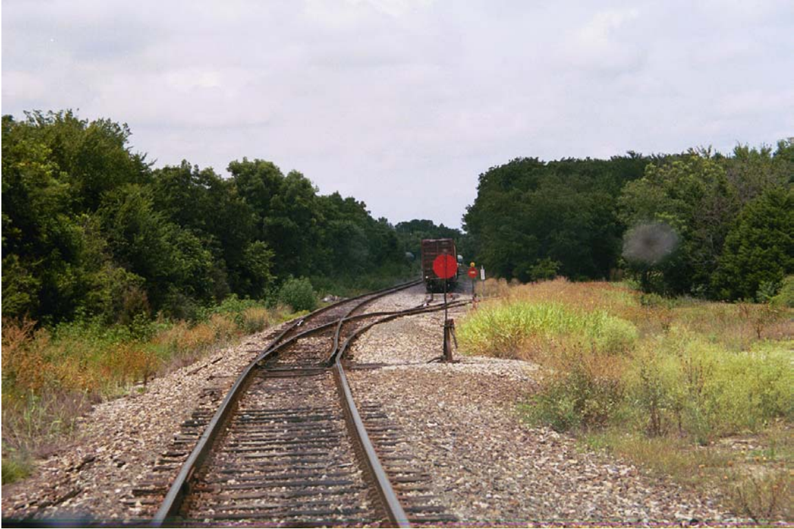
MP 42.2 Red Bird Industrial Park
