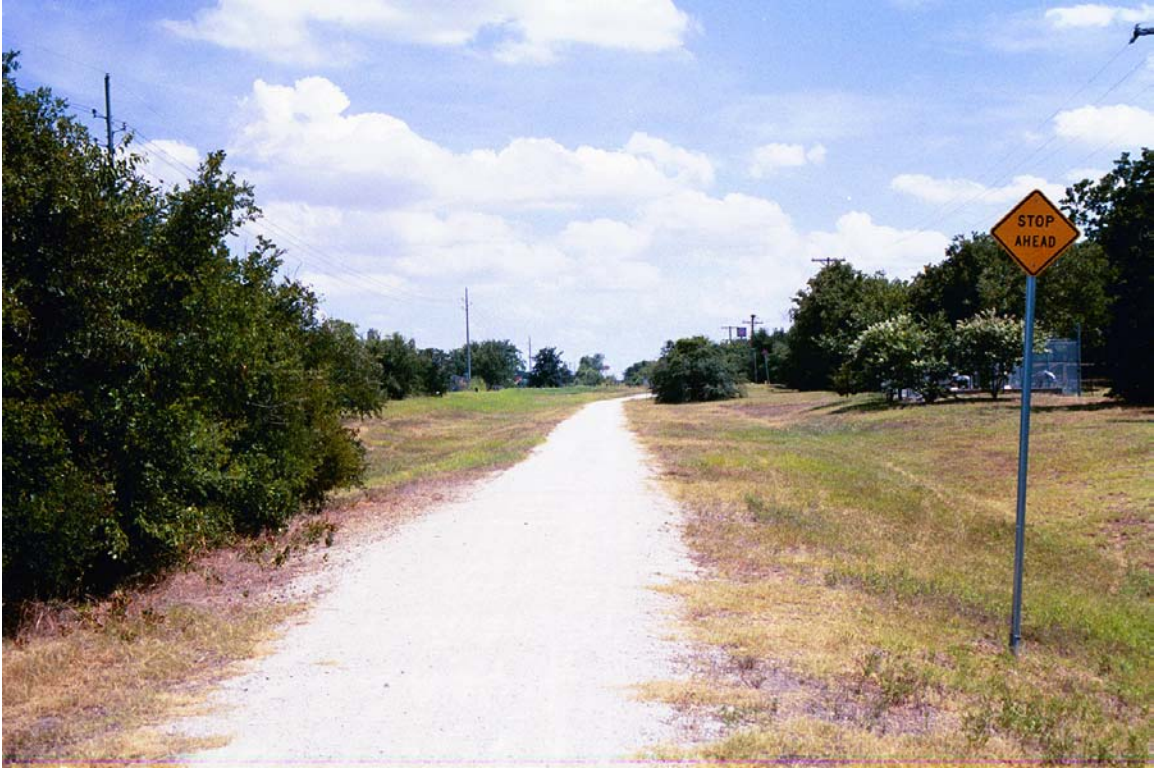
Looking SE from Bridge near Burl Street
