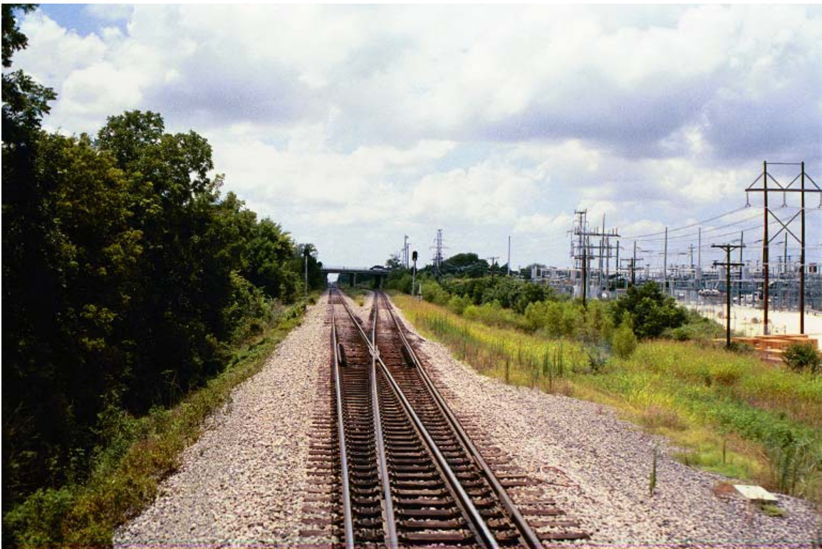
Near MP 635.8 EC Jct, Loop 12 overpass in distance
