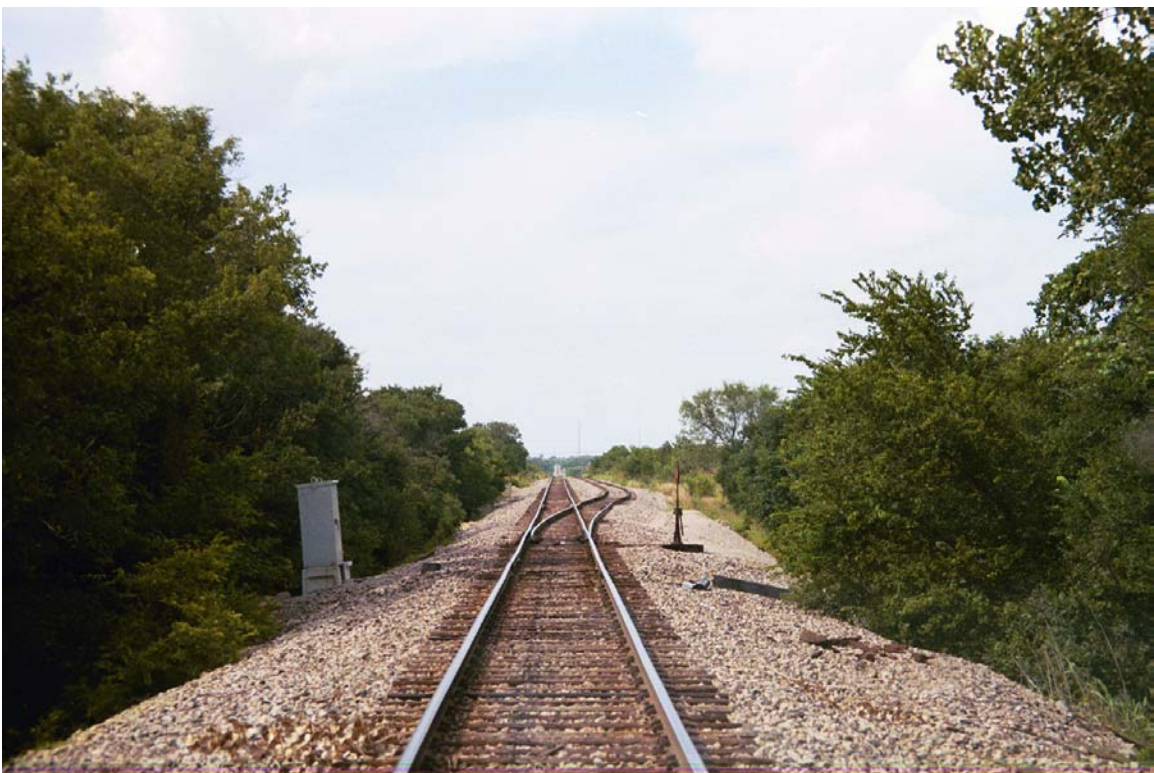
MP 693.2 South end of Hebron Siding
