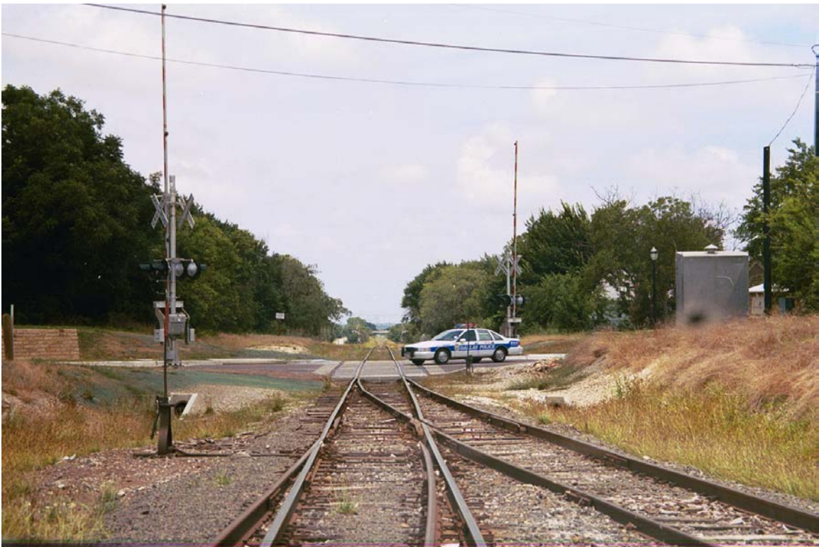
MP 34.9 Wilfy St crossing
