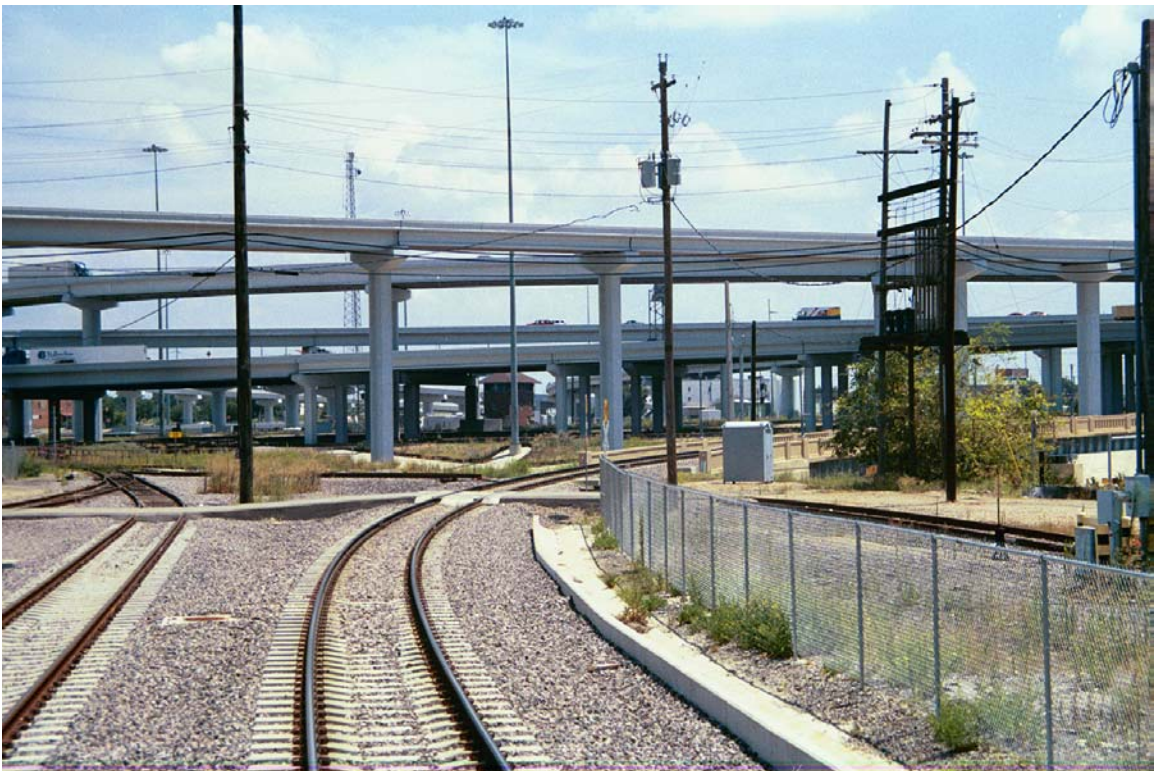
MP 610.7 Tower 55 under HWY 30
