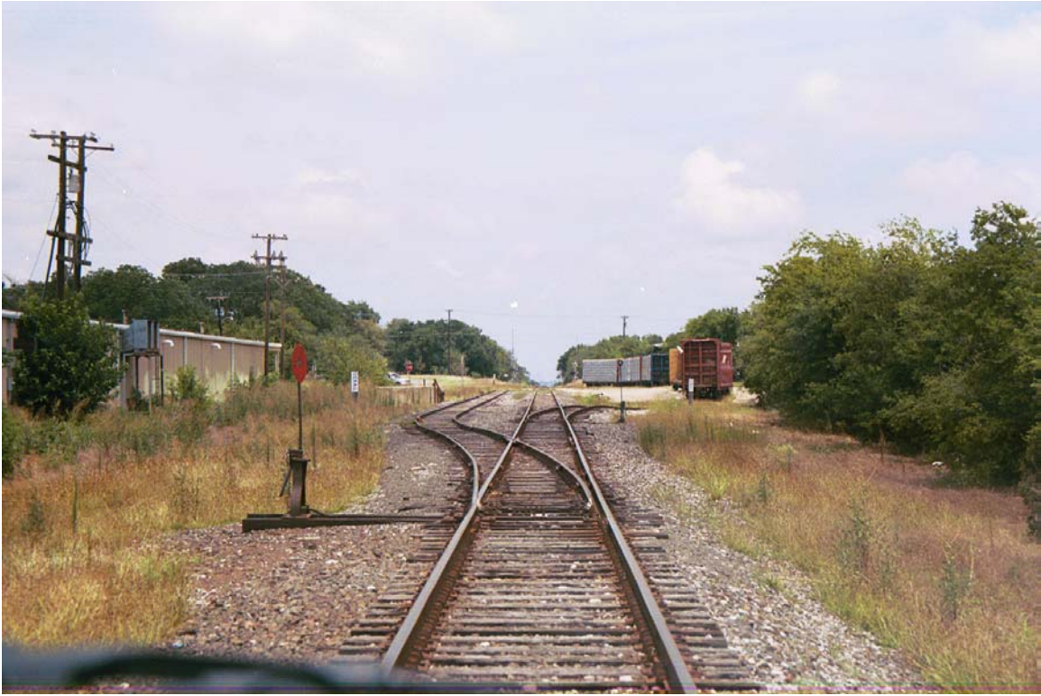
MP 34.6 Cedar Hill Belt Line Rd crossing in distance
