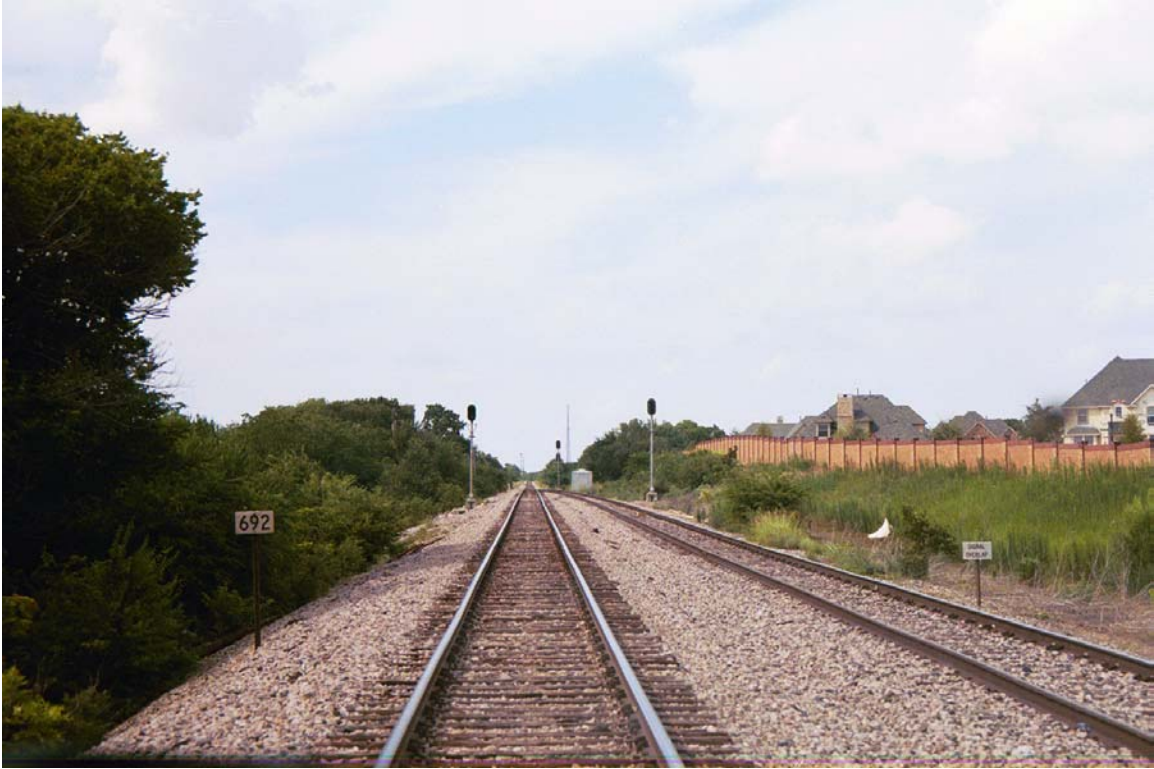
MP 692 North end of Hebron Siding
