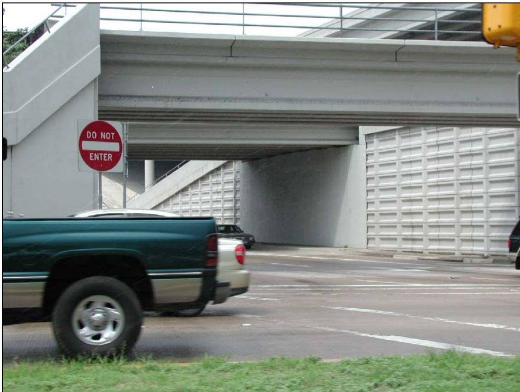
Railroad Bridge over Loop 820 SW/I 20 Service Road
