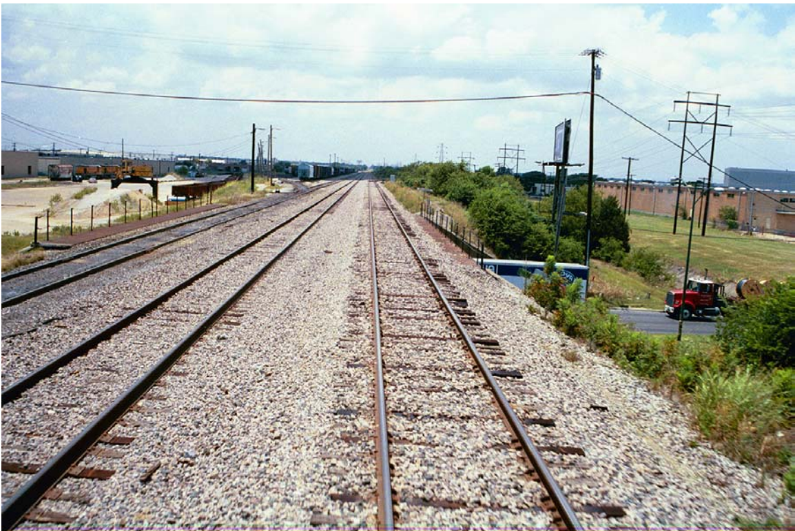
MP 638.1 Mockingbird Yard. Mockingbird Lane under tracks
