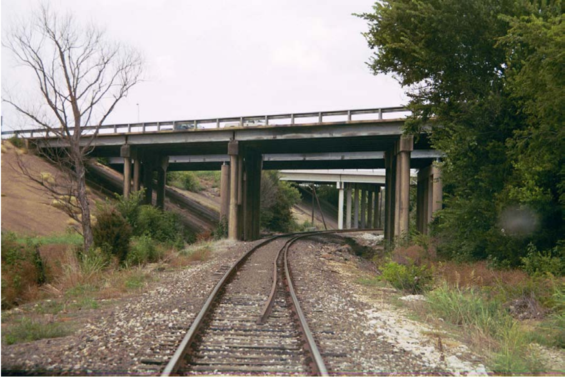
MP 43.7 HWY Loop 12 overpass
