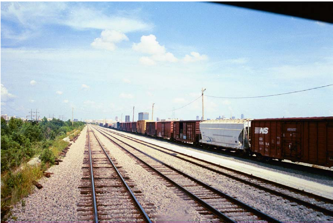
MP 638.0 Mockingbird Yard Looking East
