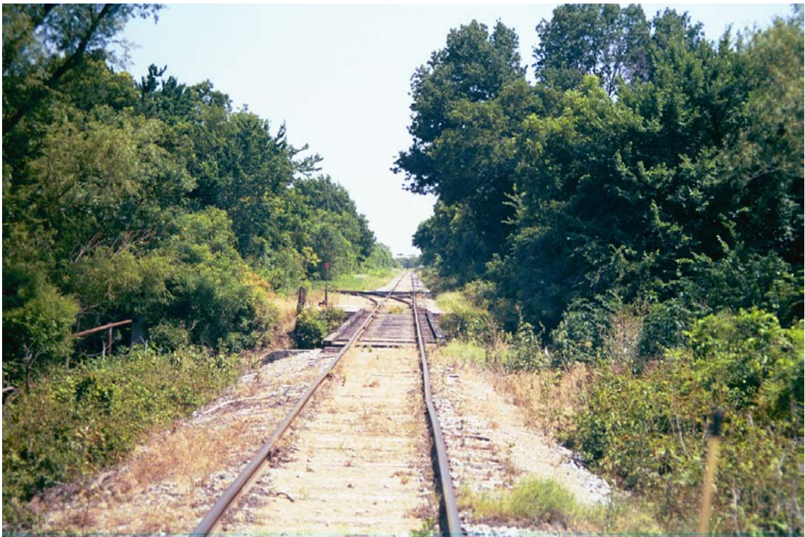
MP 736.2 – Approaching 84' long bridge and ISG industrial siding
