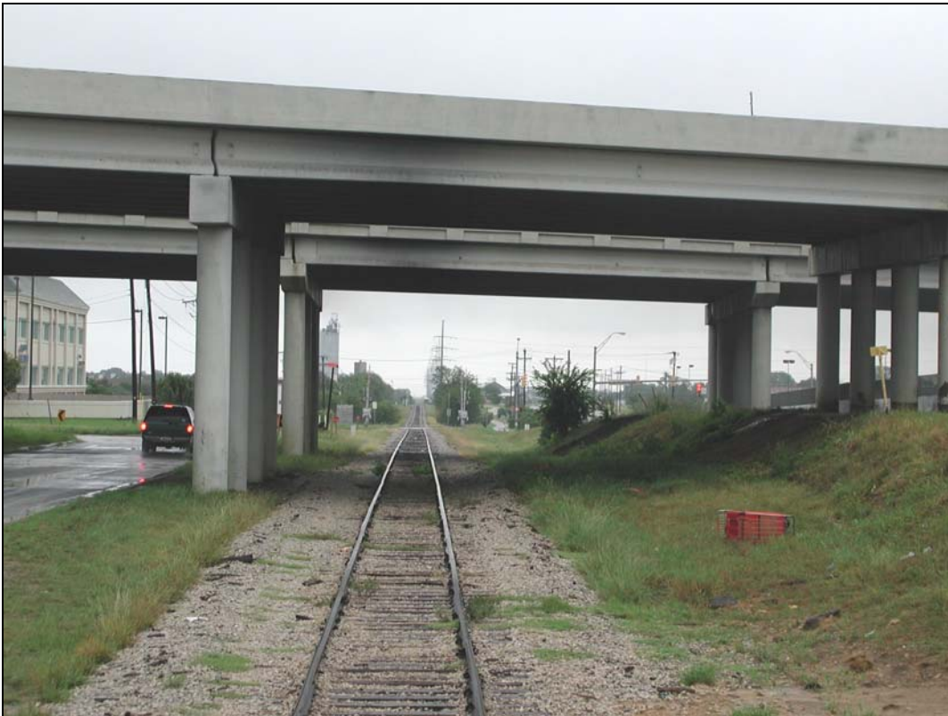
Looking East at Hwy. 114 Overpass
