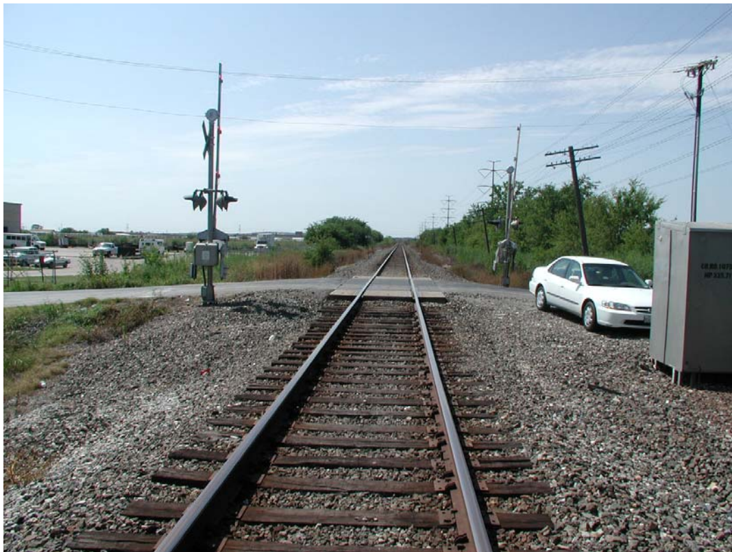
Looking South at CR 1075
