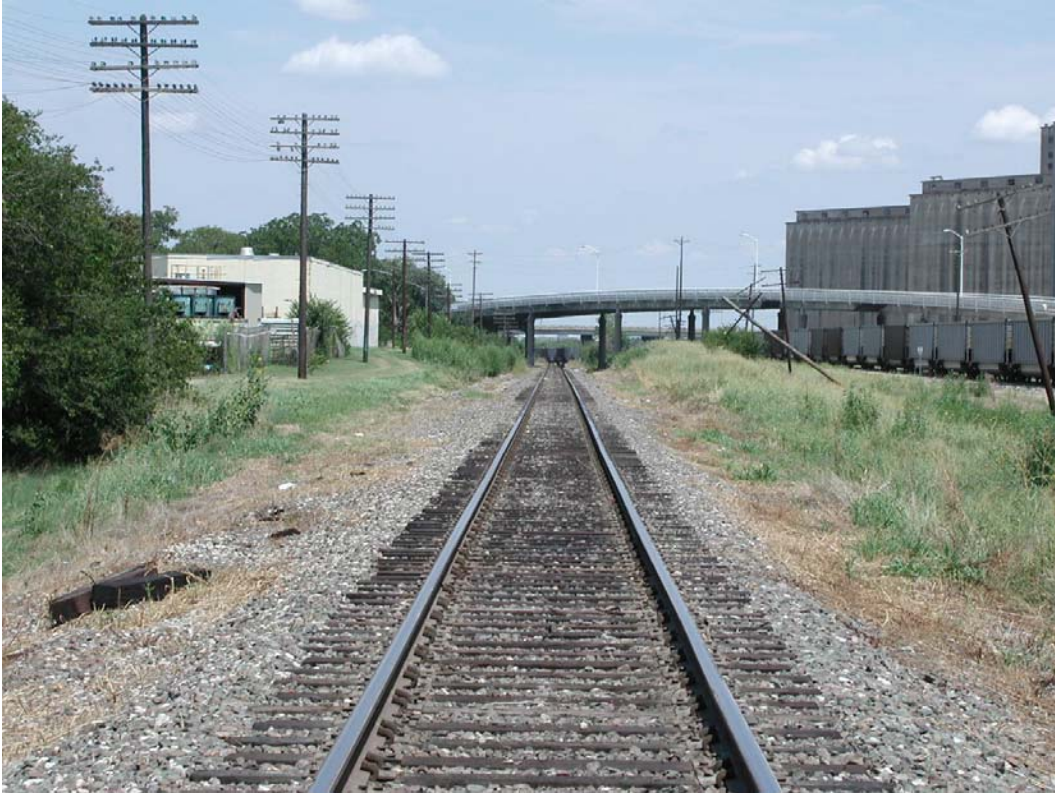
Looking North at bridge MP 344.1 & 344.3
