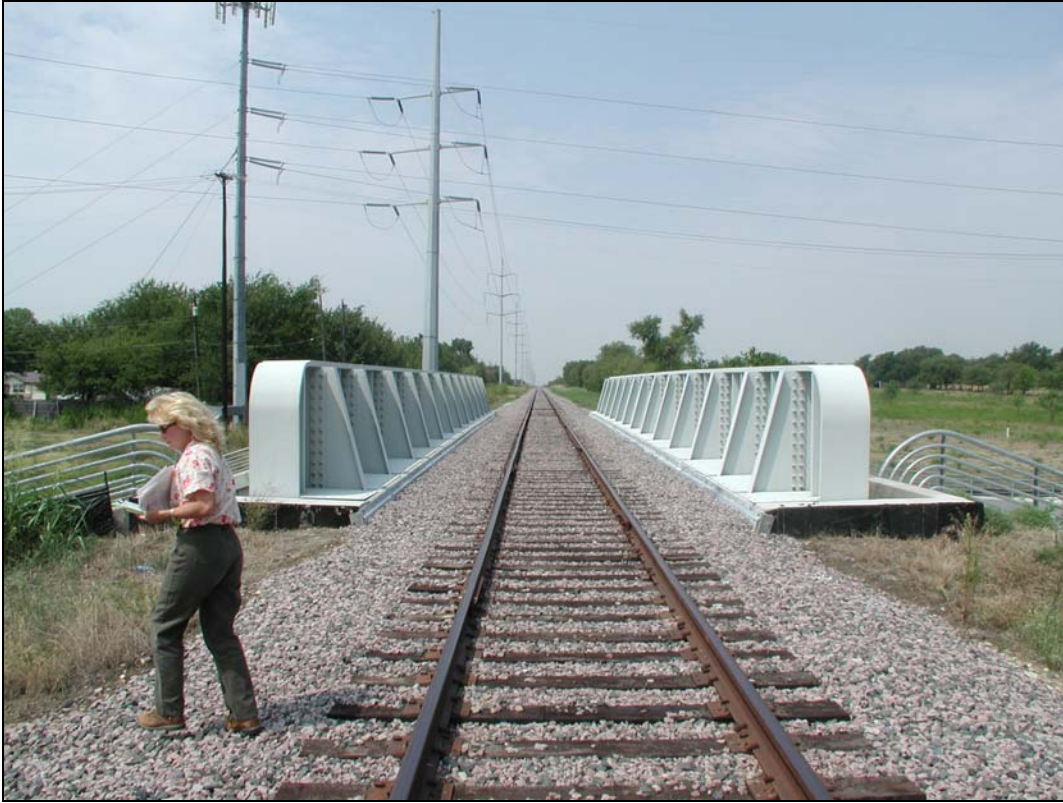
Looking East at Bridge over Business 114 (Loop 382)
