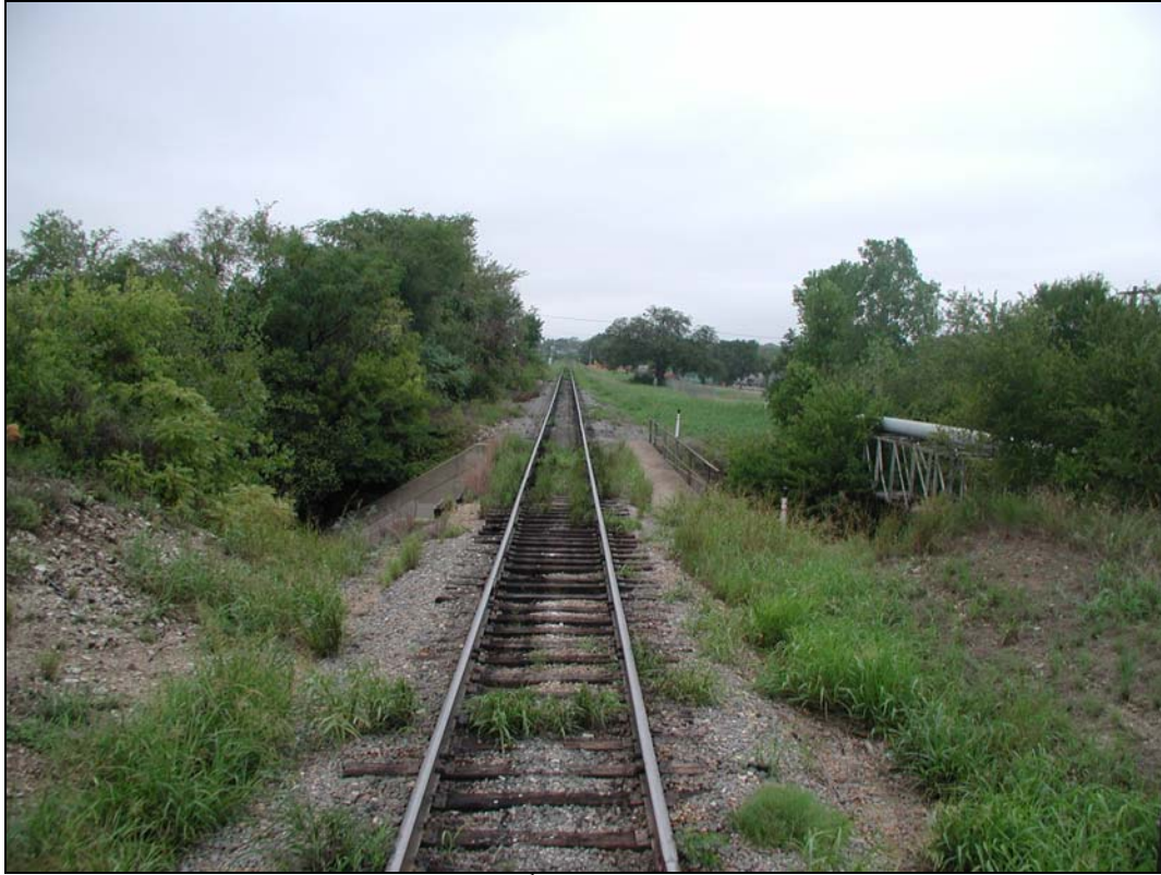
Railroad Bridge Between 28 th St. and BNSF/Cotton Belt Crossing
