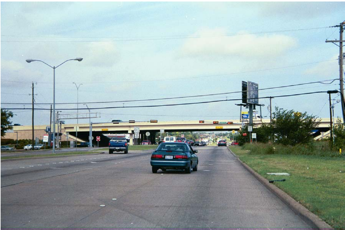
US 75 overpass and Spring Creek Parkway looking West
