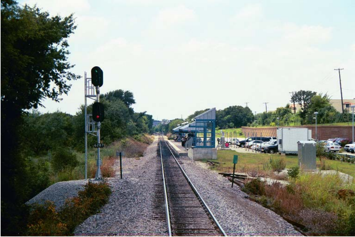
MP 628.5 Centreport Station
