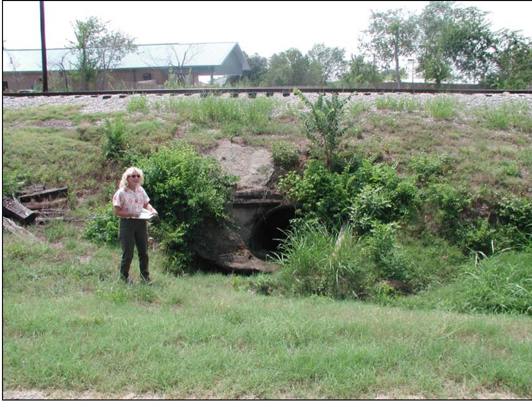
Looking North at 48" CMP 100' west of Dooley St.
