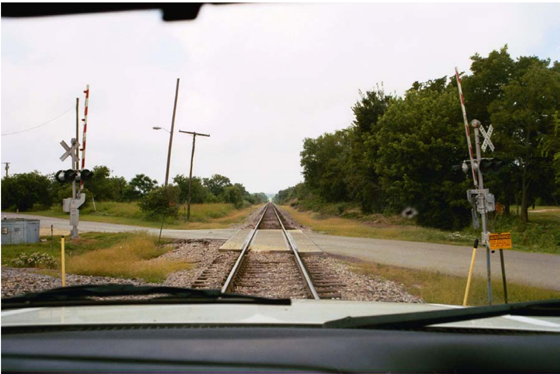
MP 788.1 Water St
