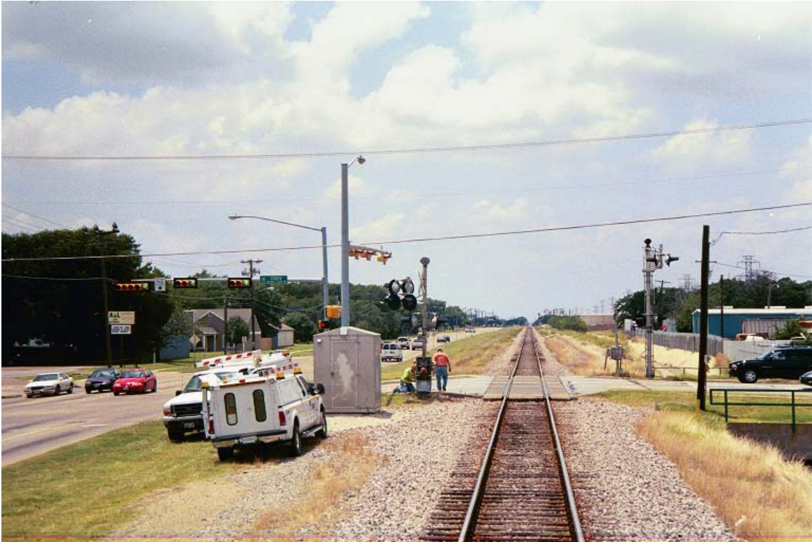
MP 633.0 Story Rd crossing
