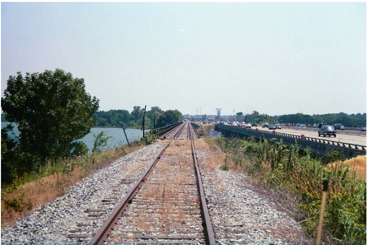
MP 732.1 – Bridge (1020' long) across Lake Louisville with I-35E to right
