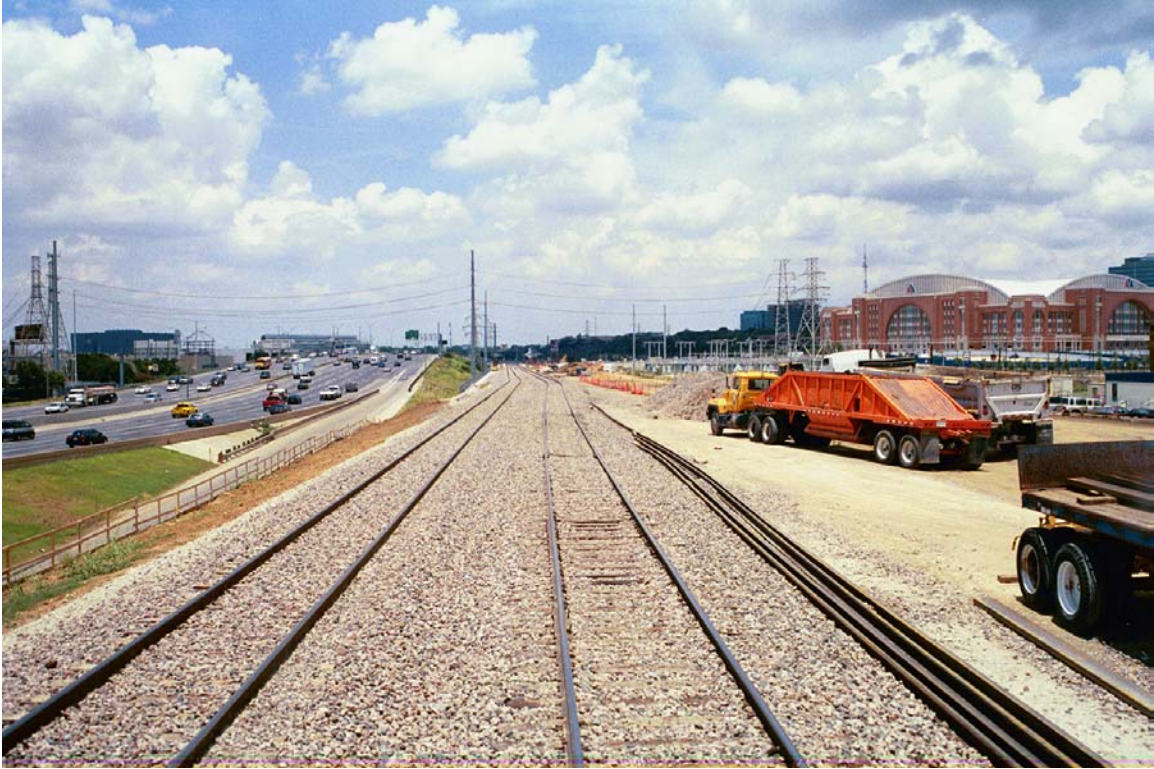
Mp 642.9 New Arena Station under construction in distance
