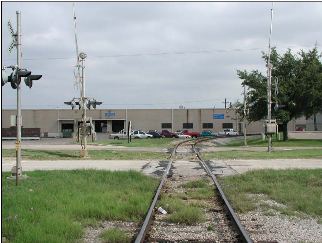
Looking north at Avenue E
