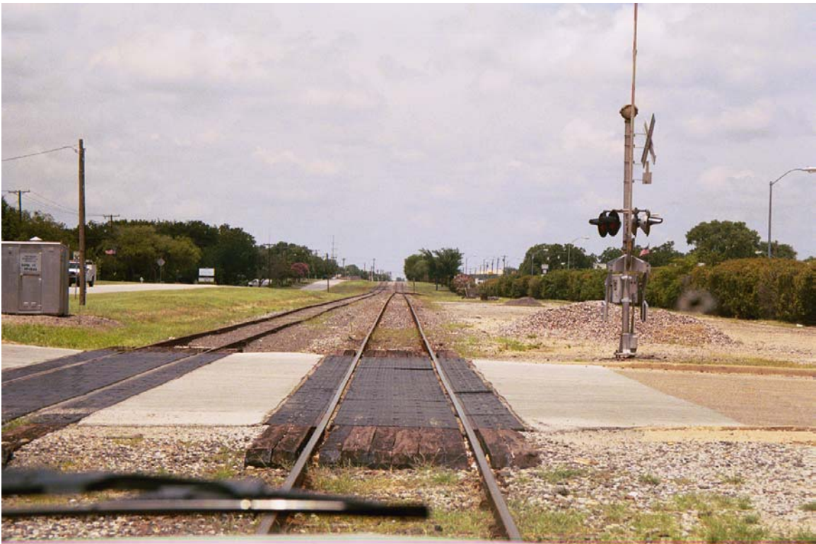
MP 40.1 Davis Street in Duncanville
