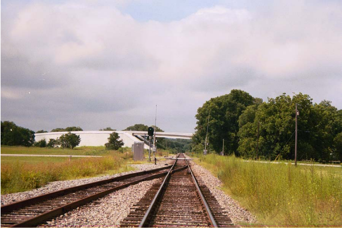
MP 782.1 (East Lancaster) South end of Lancaster siding with Beltline Rd and HWY 342 overpass in distance
