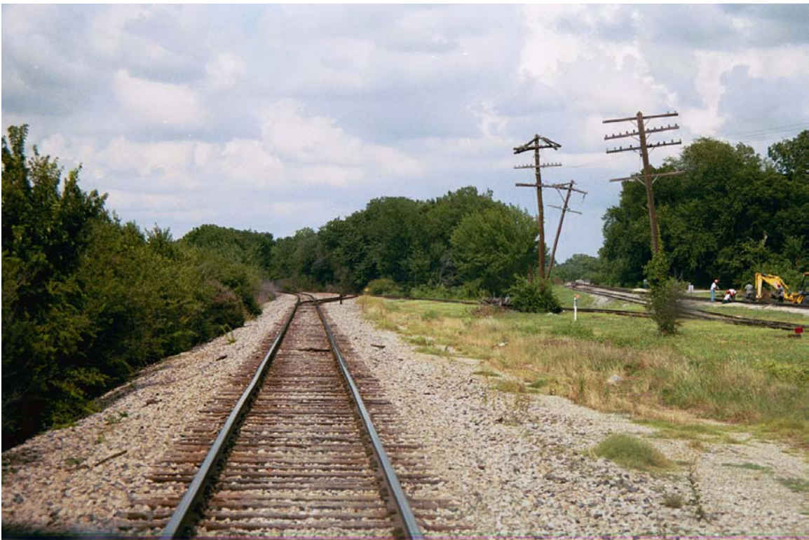
Looking North near MP 700.2
