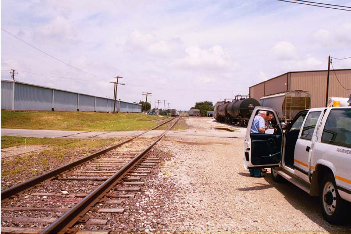
MP 26.9 F Avenue in Midlothian looking north
