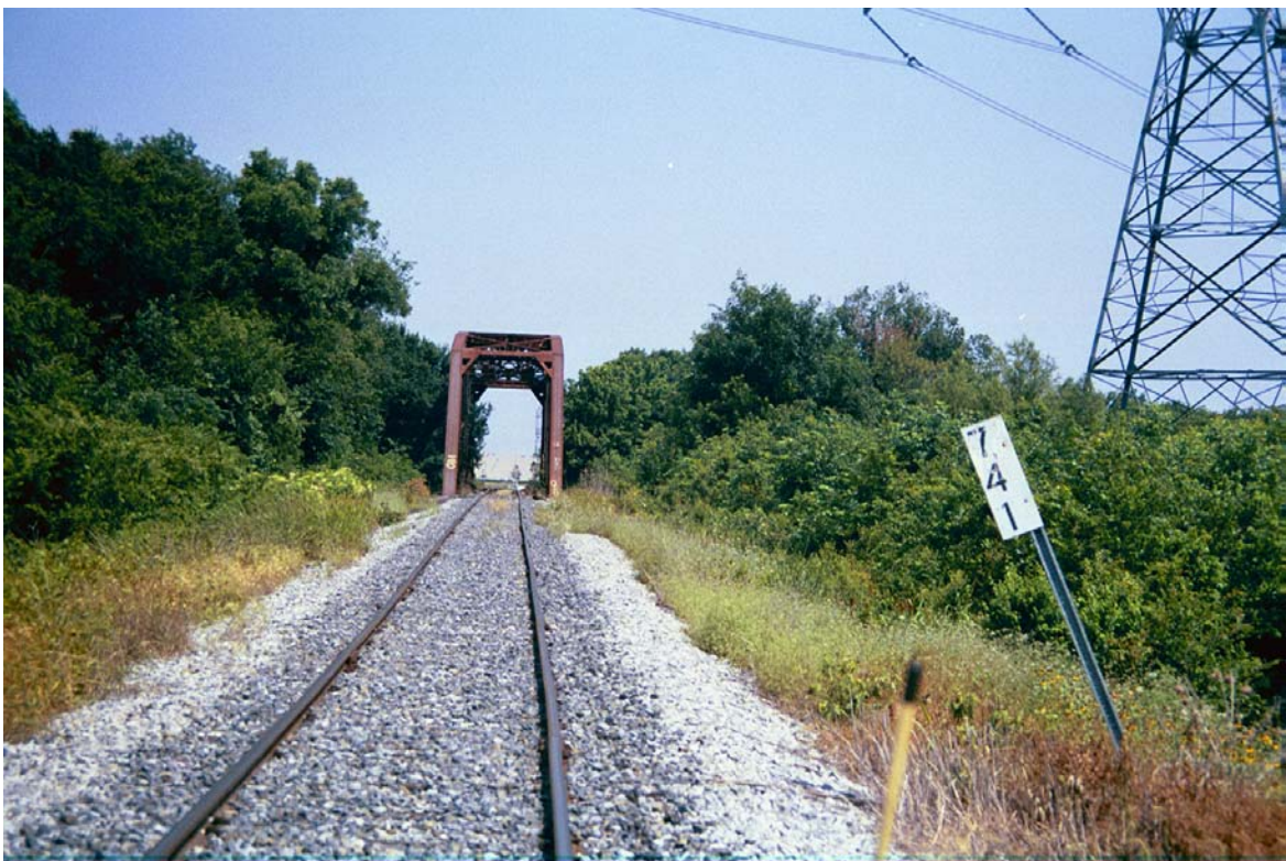
MP 741.1 – Looking south at Trinity River Bridge
