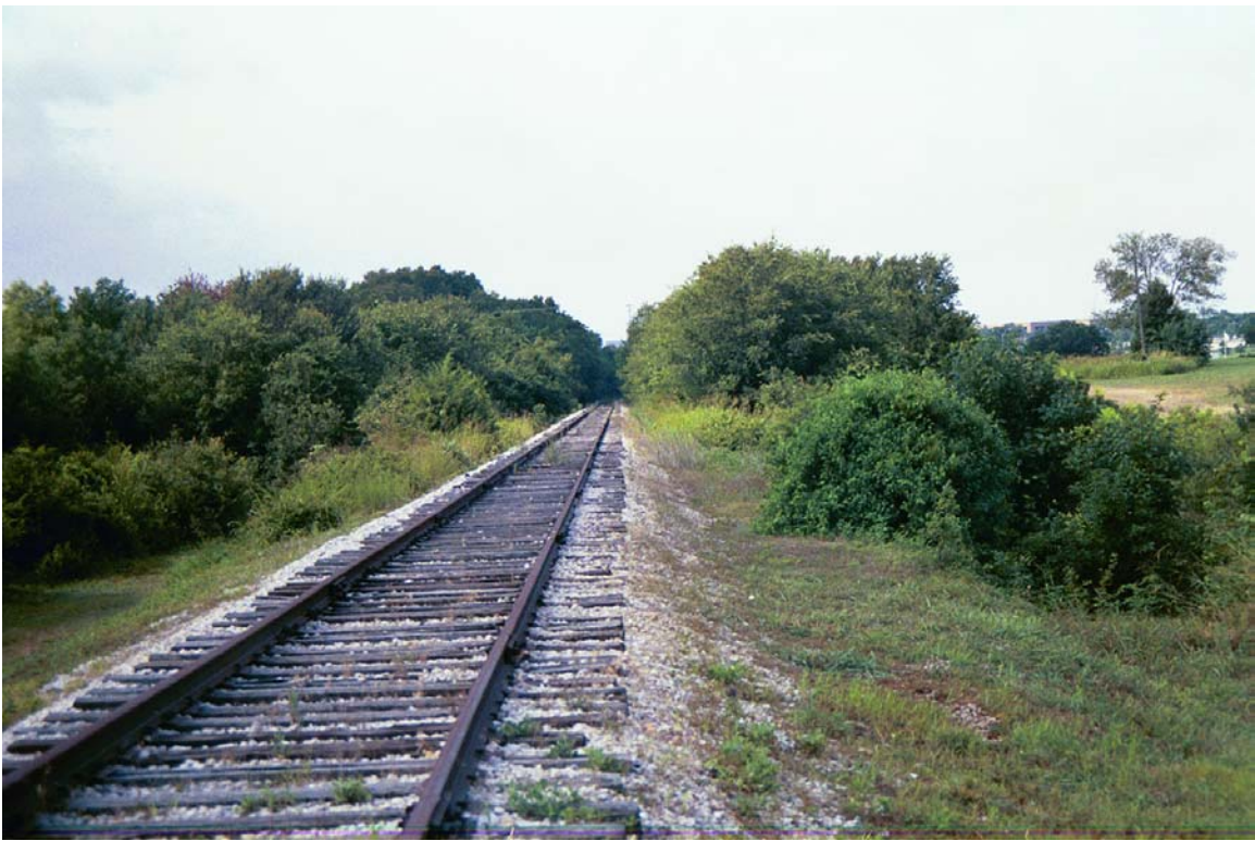
Looking North between Ridgemont and Bethany Dr
