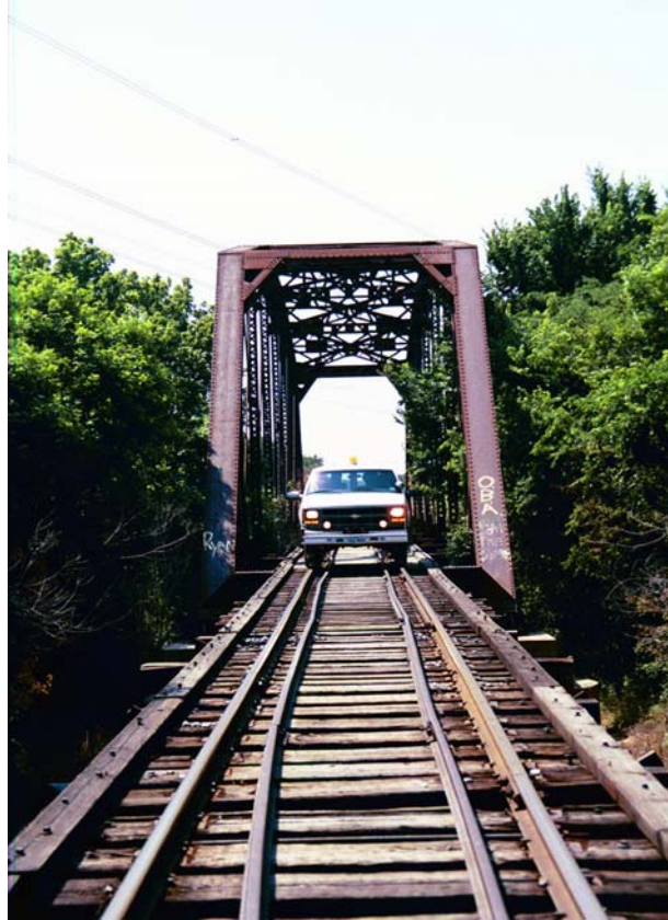
MP 741.1 – Trinity River Bridge, looking north
