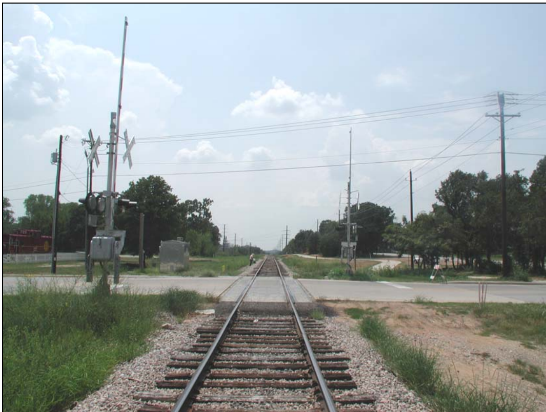
Looking West at Bransford
