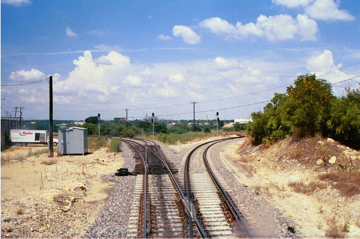
MP 611.9 6 th Street Jct. Looking East
