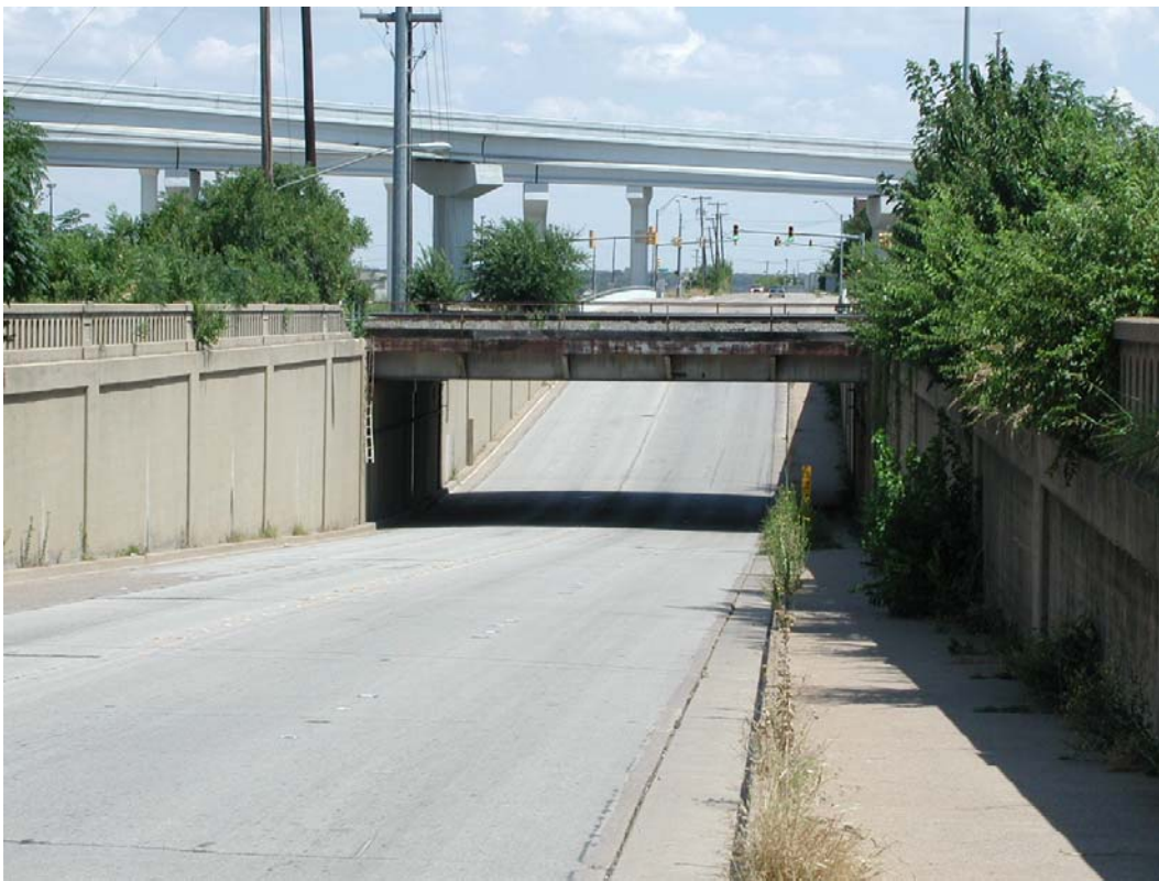
Looking at west railroad bridge elevation on Vickery
