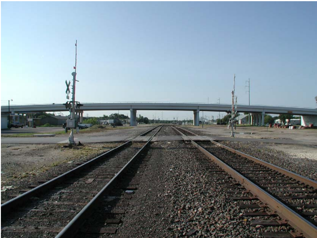
Looking West at Henderson Bridge
