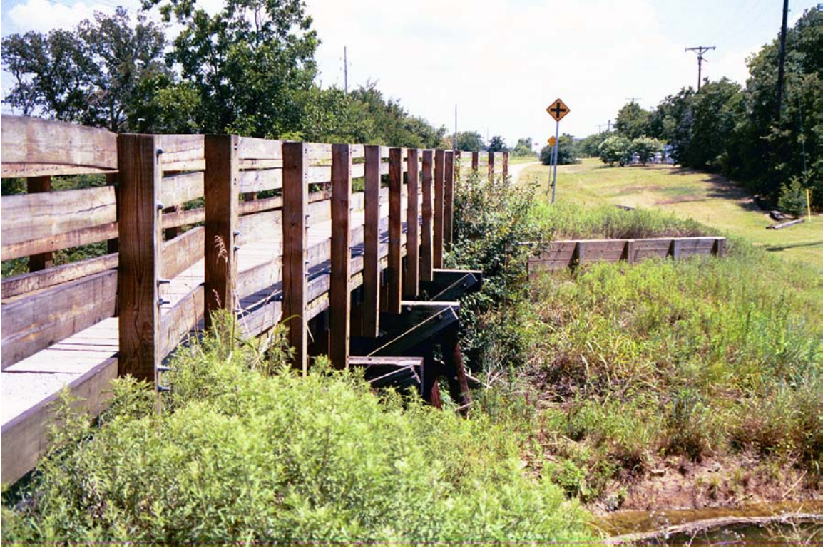
Bridge SE of Burl St Looking NW
