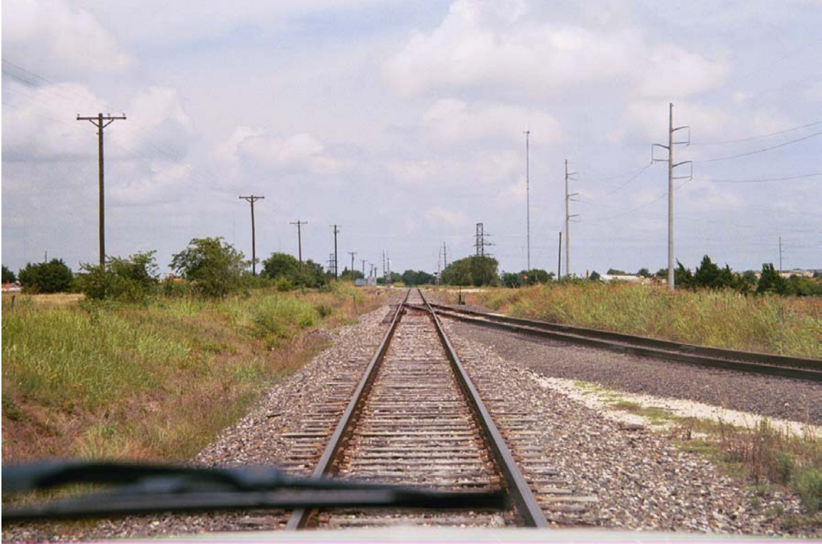
MP 28.8 Spur at north end of auto facility
