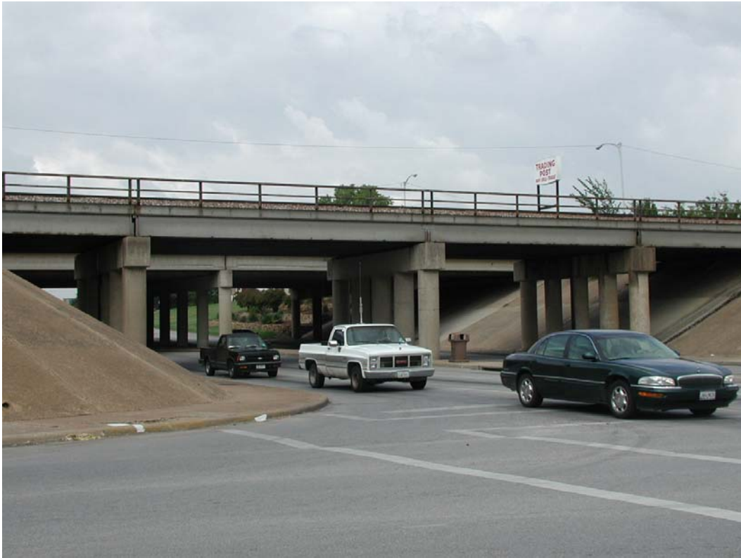
Looking North at south railroad bridge elevation on Carrier St.
