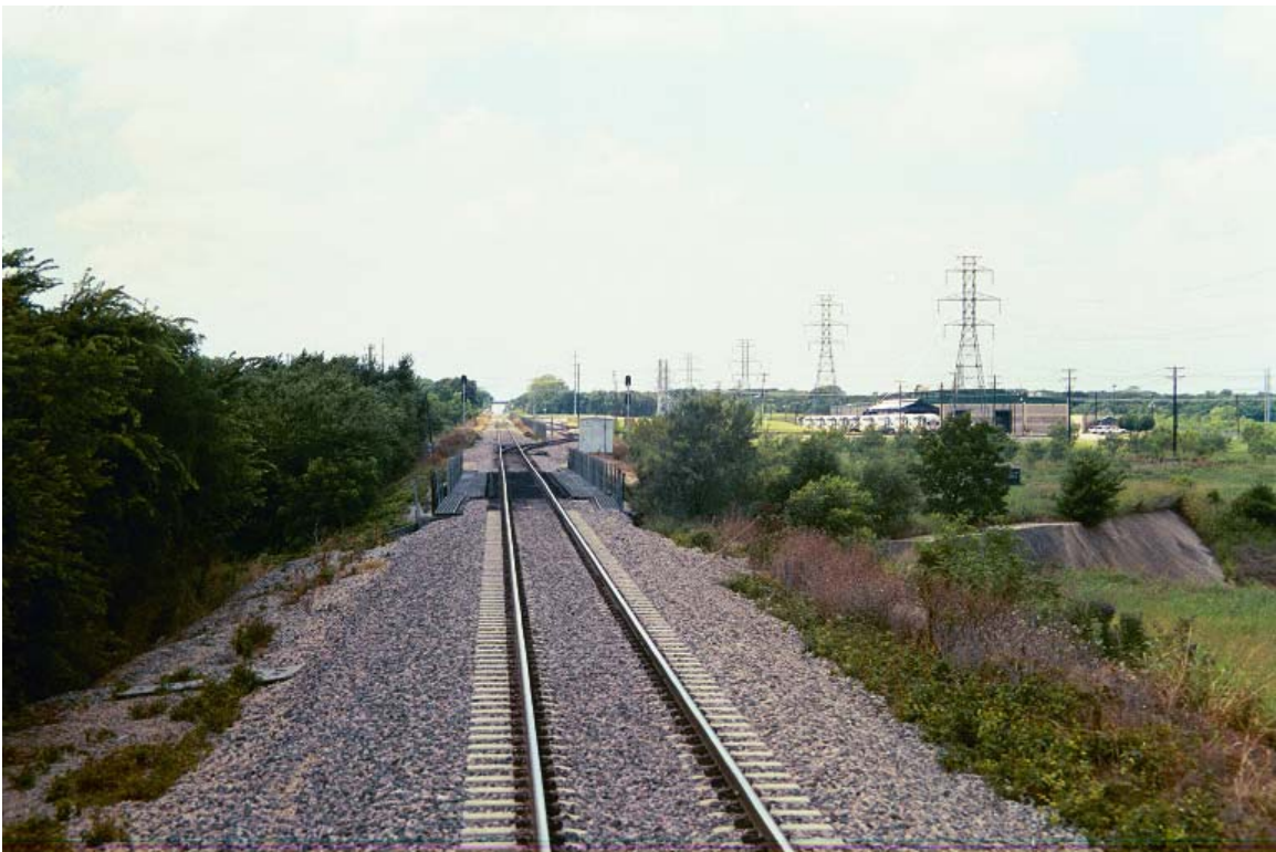
MP 630.8 Bear Creek Bridge and East end of TRE Irving Yard
