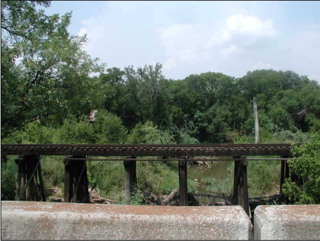
Looking North at Big Bear Creek Bridge
