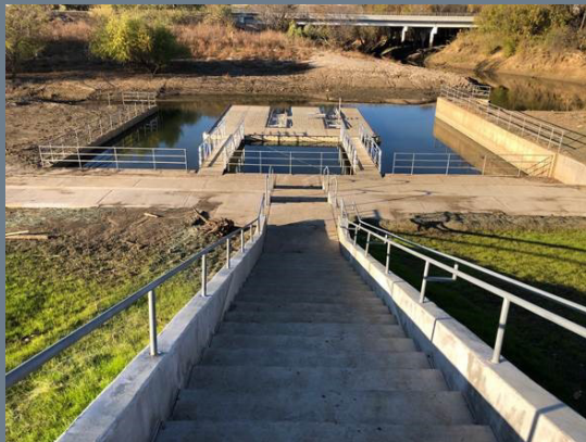
Figure 4.5: The launch site at Trinity Fork Park provides a great example of the use of concrete stairs with dual handrails to help with sliding kayaks up and down.
