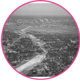
Construction of I-35 1950's
