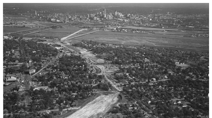
Construction of I-35 - 1950's
