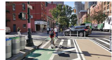
Figure 7-15: Corner Island with Flexible Delineator Posts (Source: Carl Sundstrom, PE, Office of Bicycle and Pedestrian Programs, New York City Department of Transportation)
