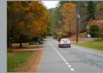
Figure 12-7: Example of Advisory Shoulders in Haveret, WI
