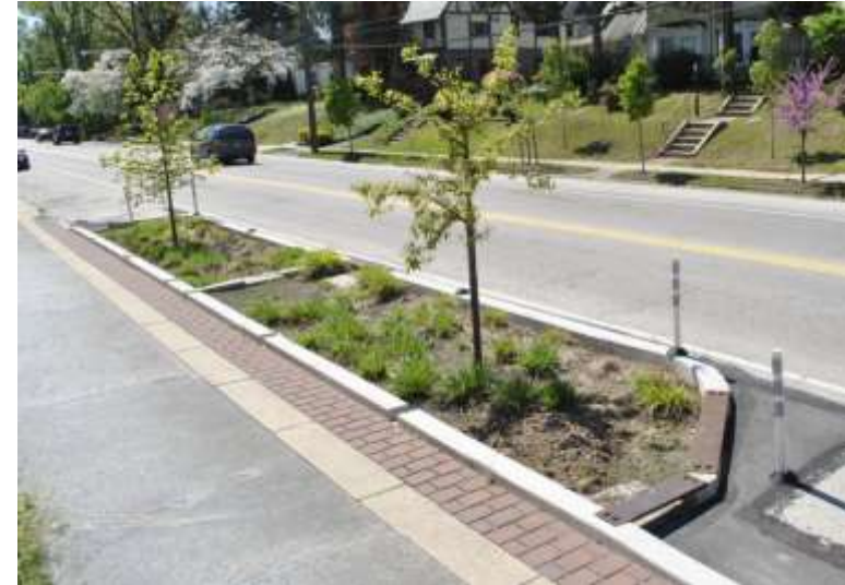
“Stormwater Bumpout” on Queen Lane, Philadelphia
