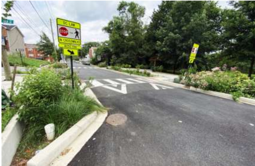
Retrofitted intersection with stormwater retention and traffic calming in DC
