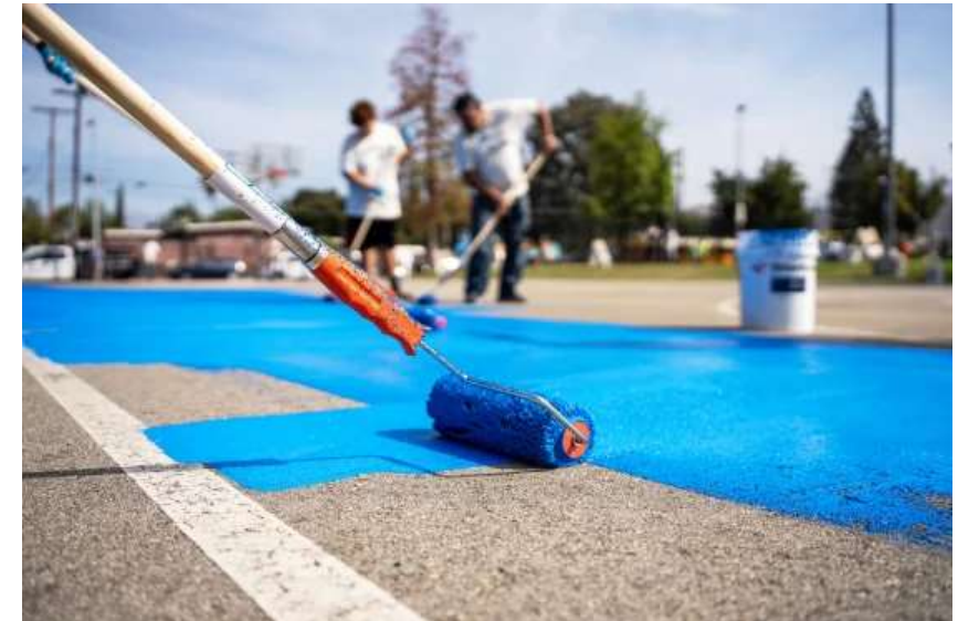
Solar reflective paint coating in Los Angeles
