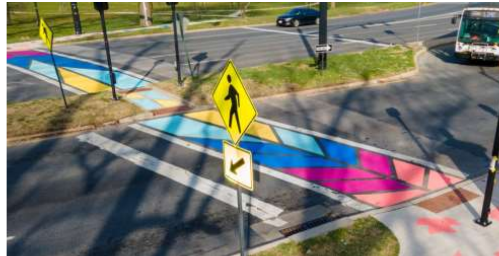
Crosswalk coating for high visibility in Baltimore, MD
