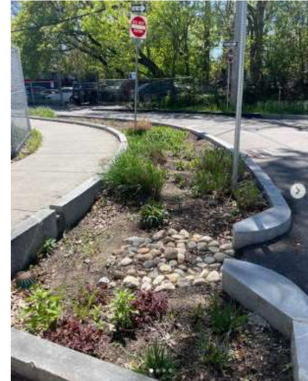
Green infrastructure curb extension in Dorchester neighborhood of Boston, MA
