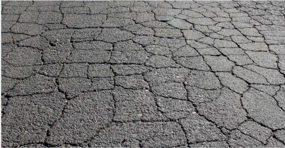
Cracking
