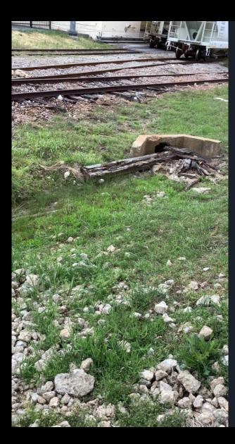
Sometimes neglect gets too much. The blockage of debris at the outfall needs to be removed immediately. The dock area is abandoned, and the crew were trying to pump the rainwater across the grass.
