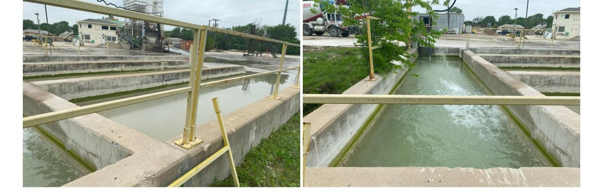
• The large deep end sloped bins allow the concrete plant to drain completely into the bins, allows the sediments to settle to the bottom and be removed by loaders one bin at a time. There are weep holes from bin to bin a few feet off the bottom to allow equalization of water to each bin. The well at the rear has a small orifice opening near 4" and a few feet deep to act as a weir.
