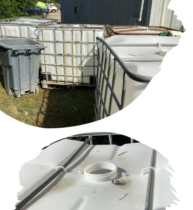
Large empty unmarked admixture tubs waiting for removal by the manufacturer did not have a lid over the openings. I asked the supervisor to place some type of lid or seal over the open containers.
