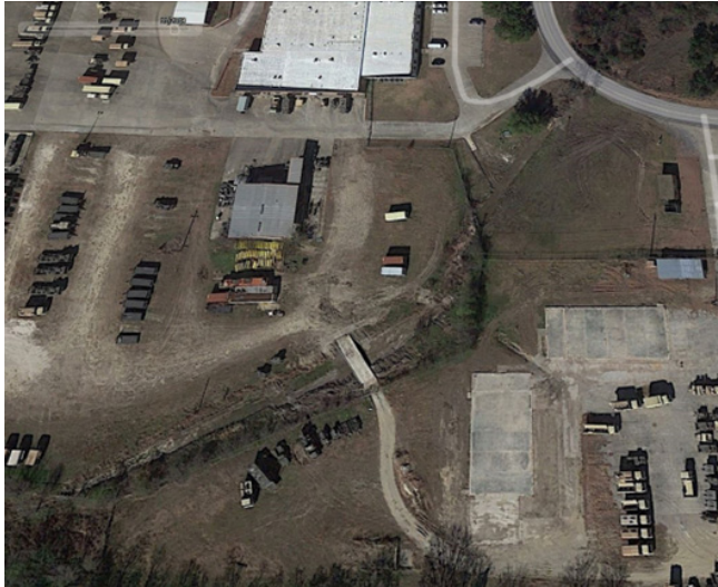
Photo: Drainage ditch with bridge at Shoreview facility
