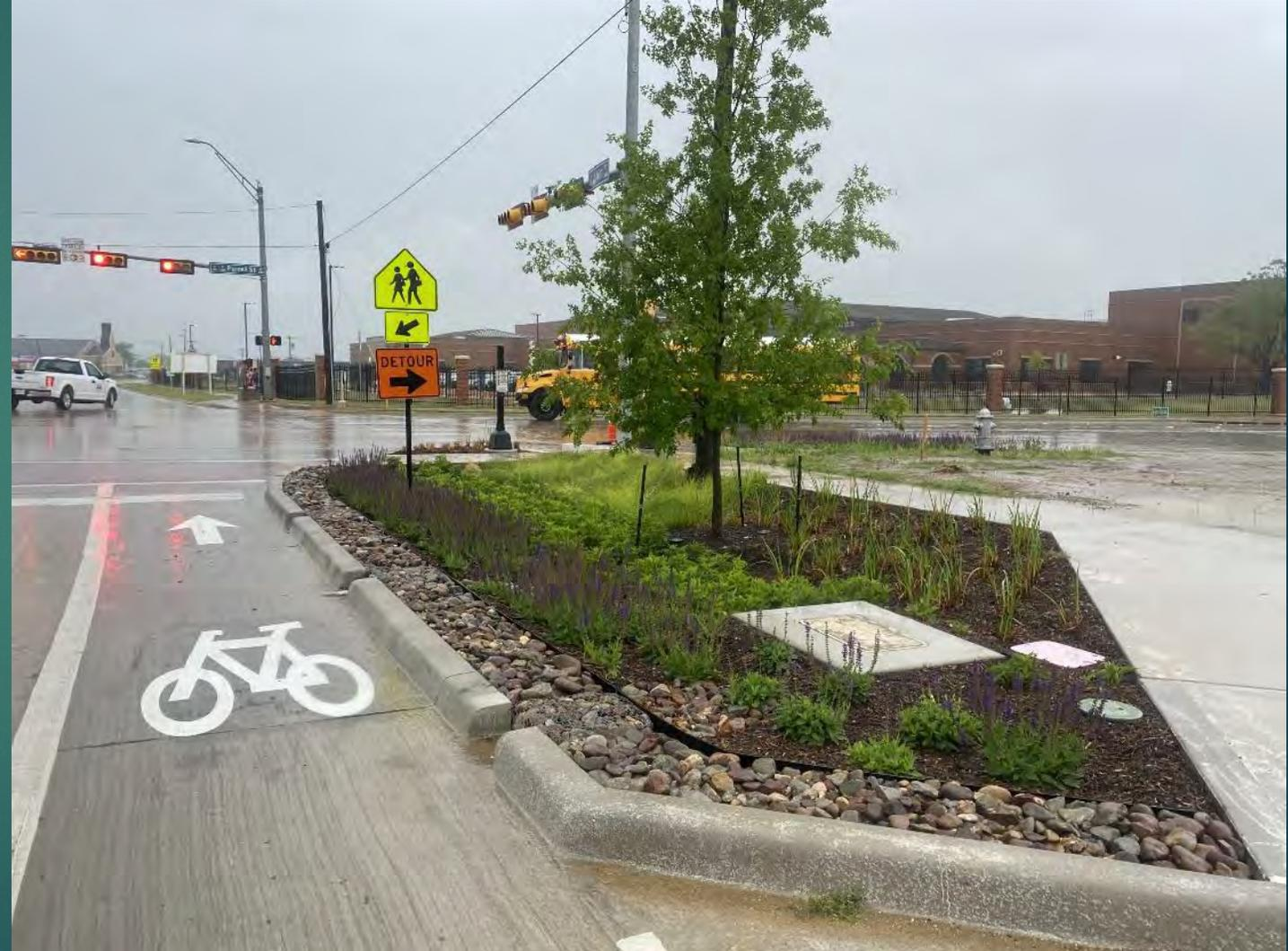
Curb cuts (18" wide) allow storm water from street to enter the swale
