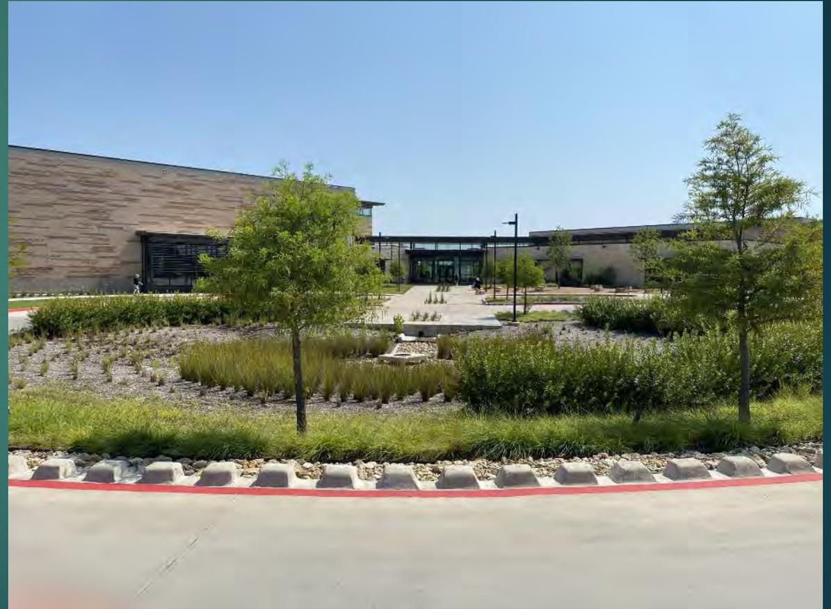
Saw Tooth Curb around the roundabout to provide for stormwater entry
