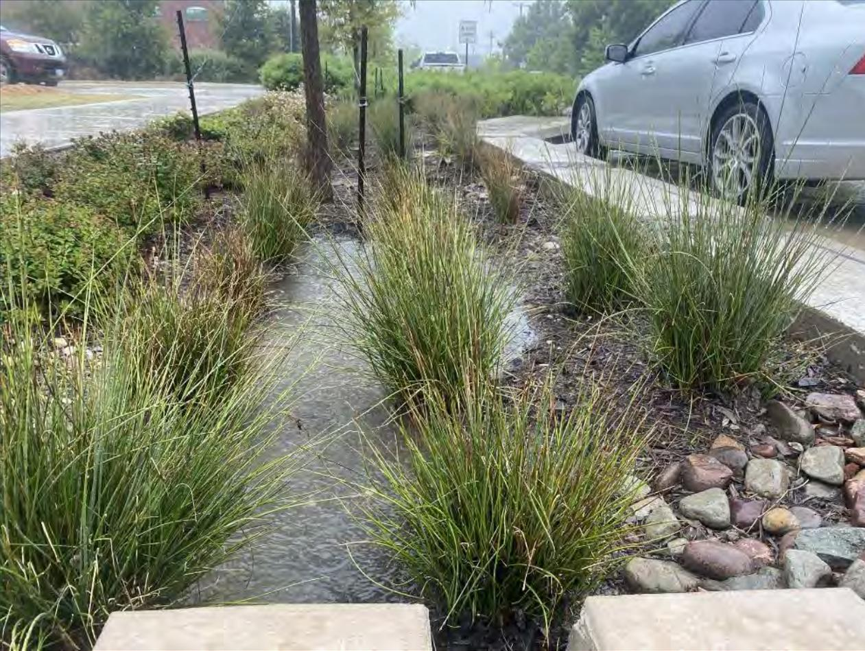
Slight **longitudinal slope** keeps water moving slowly while
