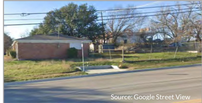
Figure 1. Route 002 Bus Stop Lacking Sidewalk
