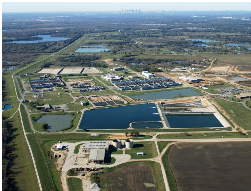
Figure 7-1: Southside Wastewater Treatment Plant
