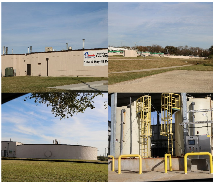
Figure 7-3: City of Denton Pecan Creek WWTP
