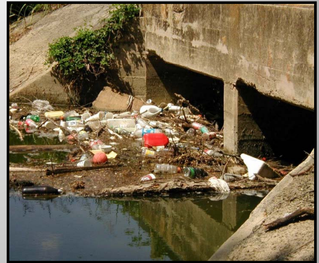
Trash and debris
