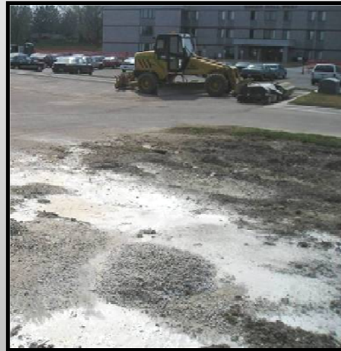
Wash out of solids/liquids
