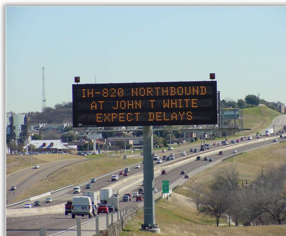
Dynamic Message Signs provide travel-time estimates and other information to improve commutes.
