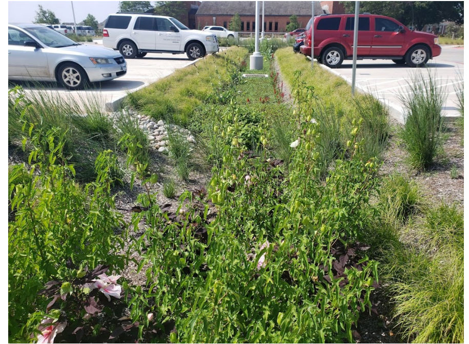
Above: Bioretention in a parking lot; Below: Bioretention Cell (Credit: Texas A&M AgriLife)
