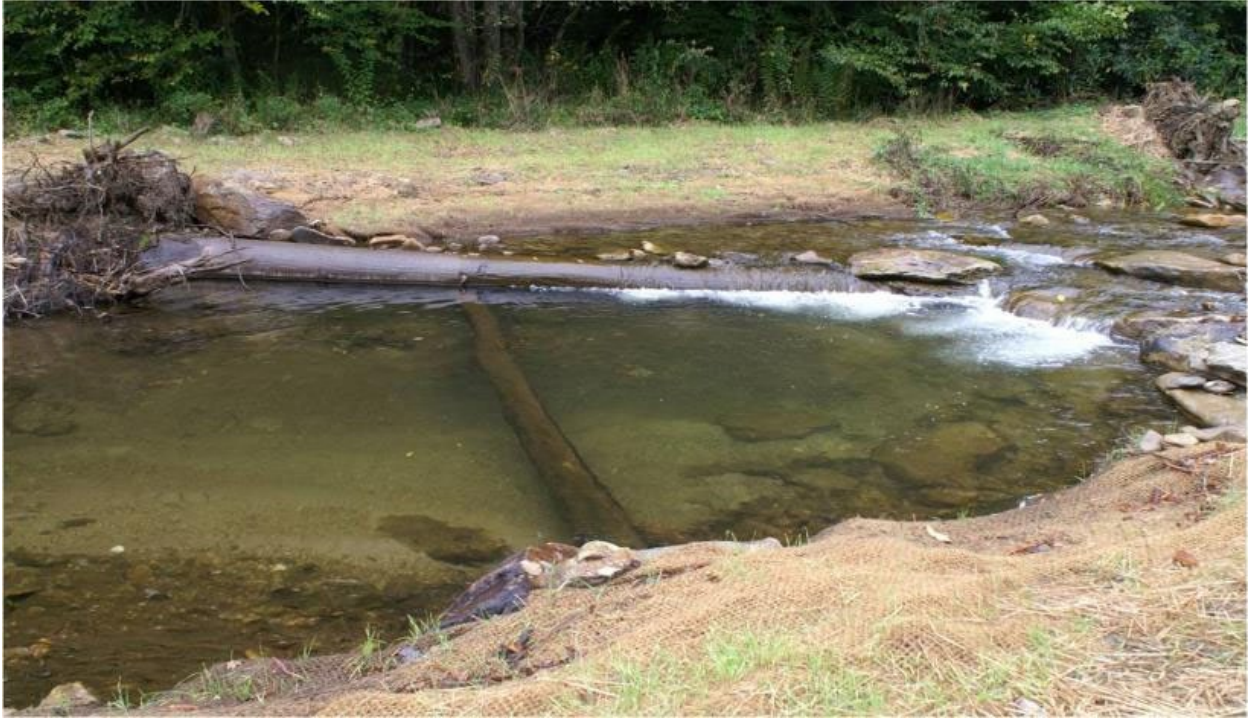
Large Woody Debris Cover Log in a Pool
