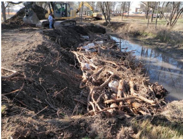
Toe Wood (Under Construction)
