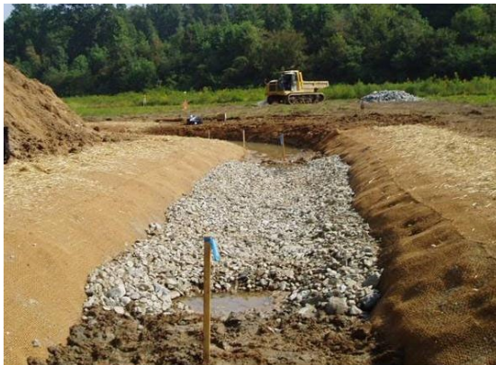
Constructed Riffle during Construction
