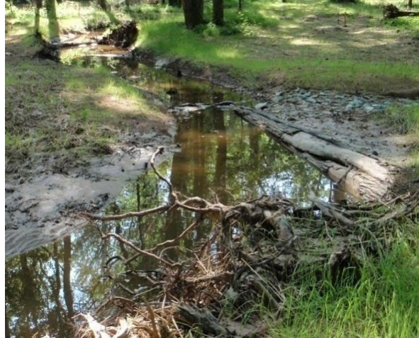
Log Vane and Root Wad Structure
