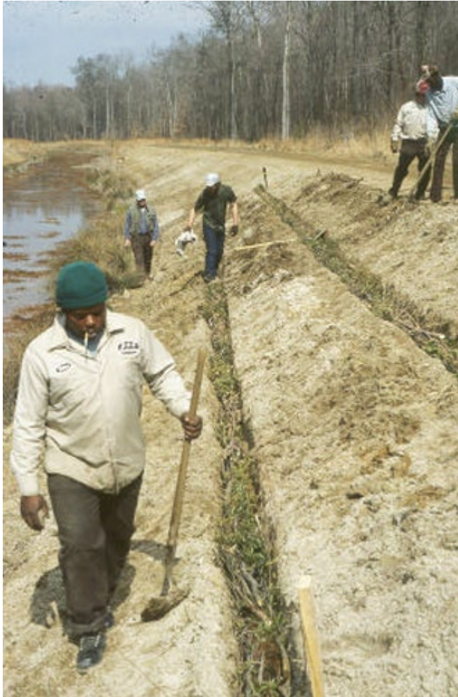
Installing Live Fascines
