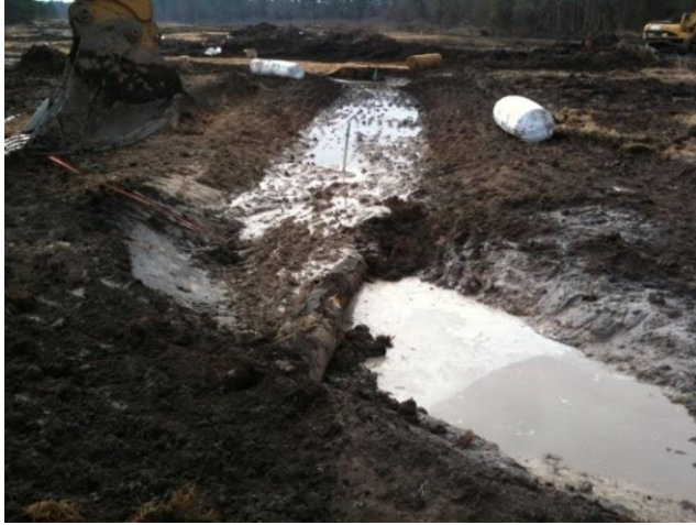
Log Vane (Under Construction)
