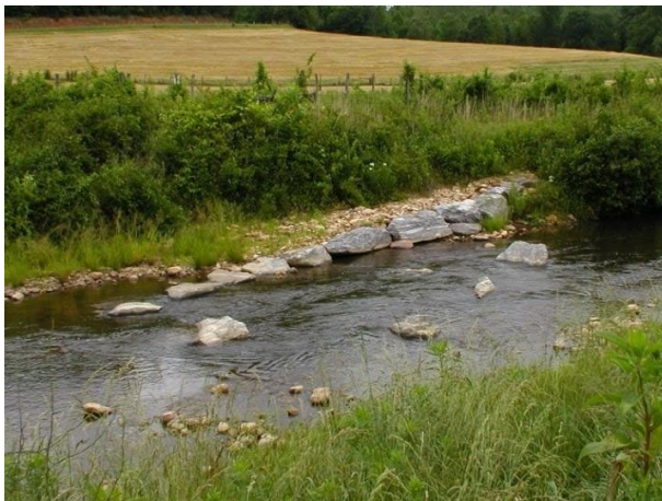
J-Hook and Rock Vane Examples
