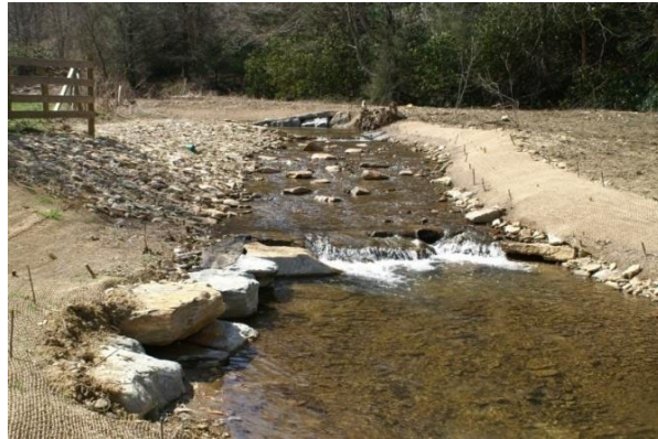
J-Hook Example (Rock) (Under Construction)
