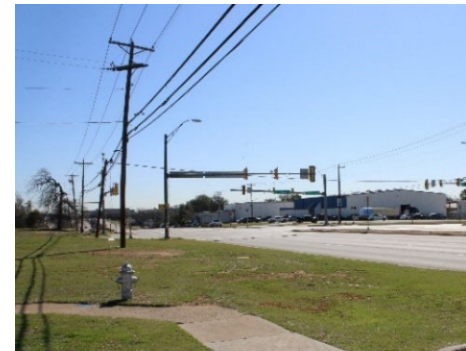
Power lines in the Hurst Boulevard right-of-way.
