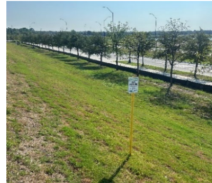
Example of the steep elevation change along the TRE Corridor ROW near the Trinity Lakes Station.
