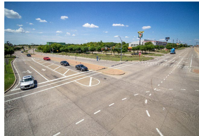
Example of turn-lane striping to better indicate turning movements within an intersection.
