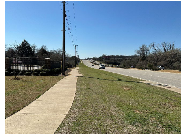
The segment of Hurst Boulevard between Precinct Line Road and Hurstview Drive is nearly 0.7 miles long with no places for pedestrians to cross in between the signalized intersections.
