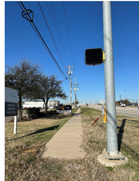
Sidewalk gaps are prevalent in many portions of the study area, including near intersections where sidewalks abruptly end.
