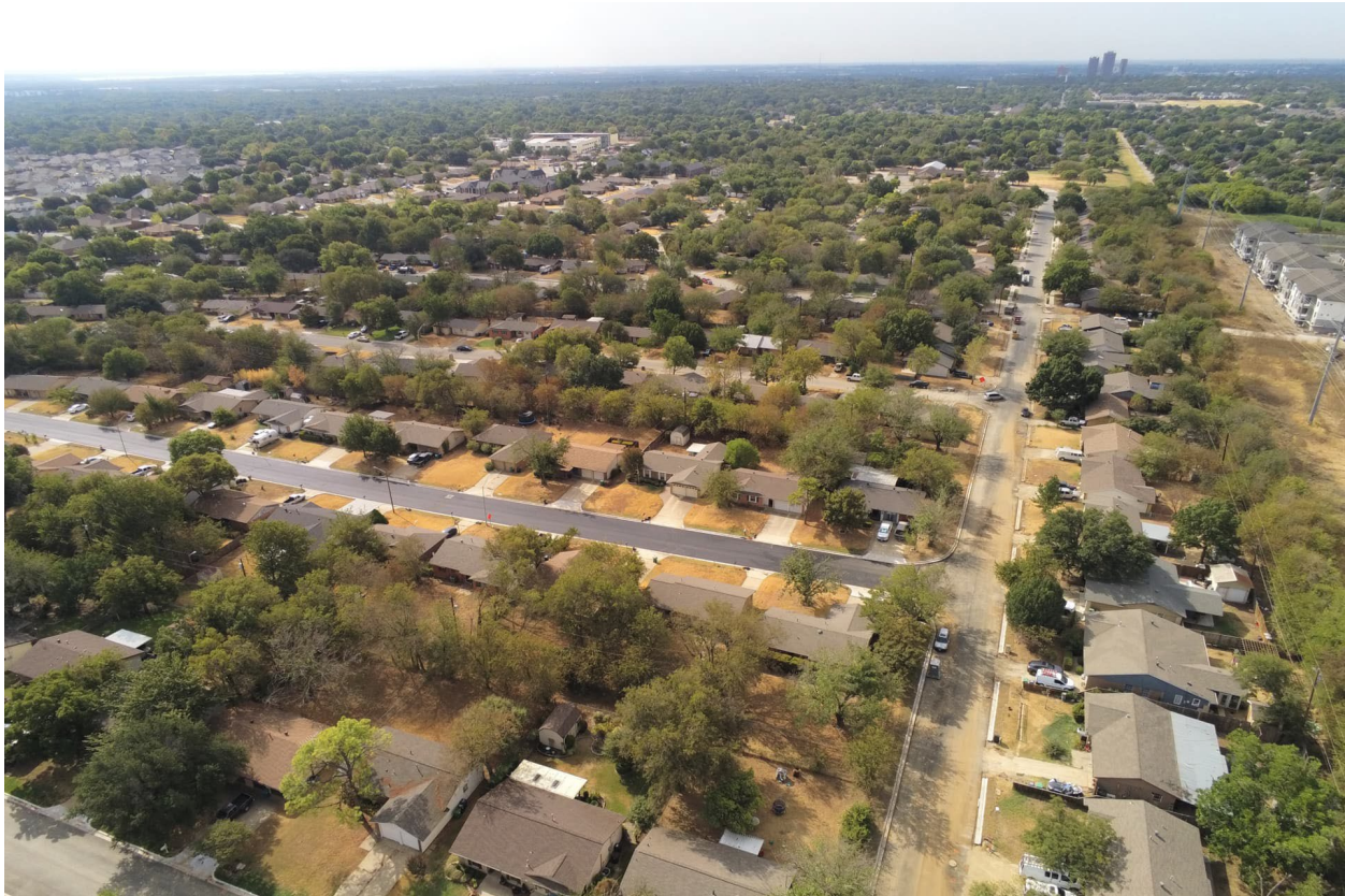
Crews are wrapping up work on Redstone Road in Denton. (City of Denton)
