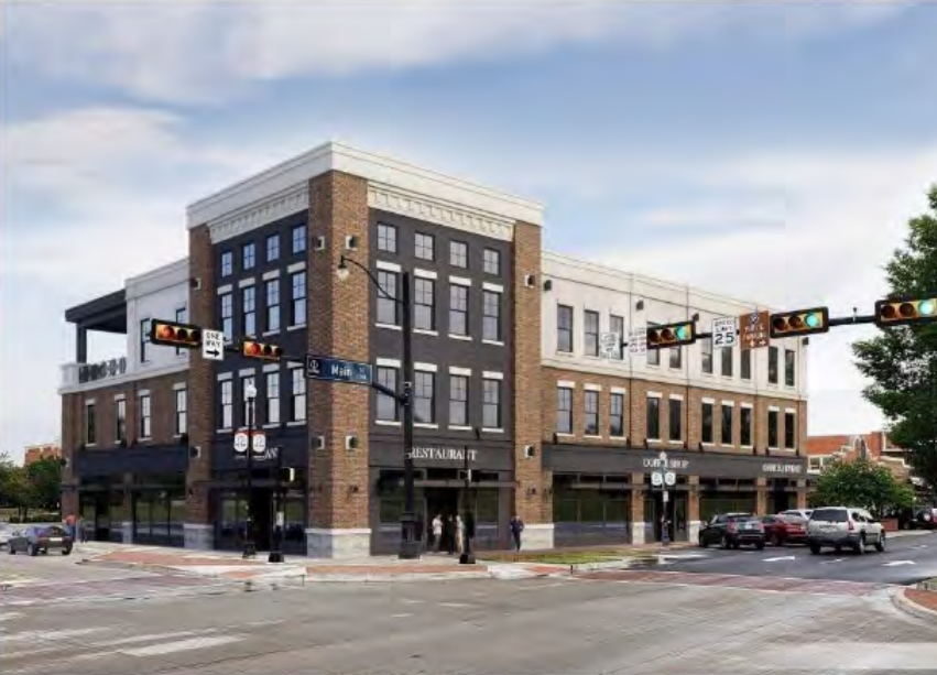
Deck on Main – credit: City of Lewisville
