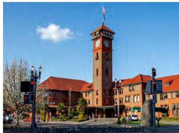
Portland Union Station Credit: Amtrak
