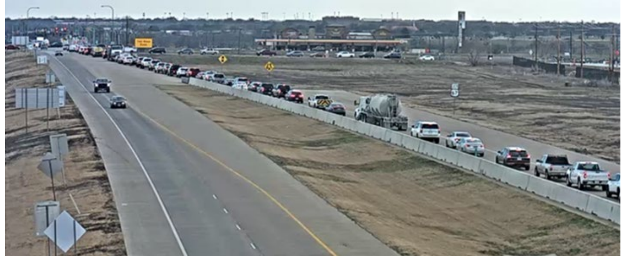
Southbound Chisholm Trail Parkway congestion on approach to US 67 interchange (NTTA)
