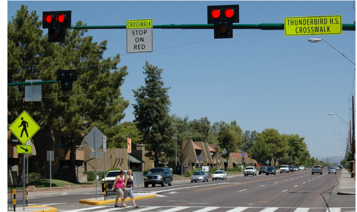
The HAWK beacon is a pedestrian crossing that uses a red light indication to stop vehicular traffic on an as-needed basis, allowing pedestrians more time to cross busy roadways away from a signalized intersection.
