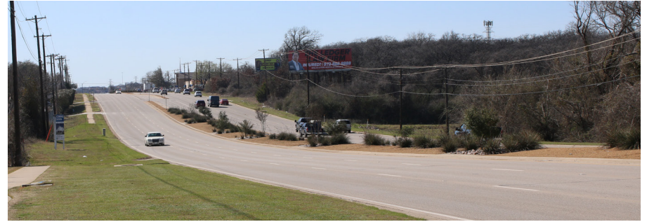
View of Hurst Boulevard facing west from the Central Catalytic Site.
