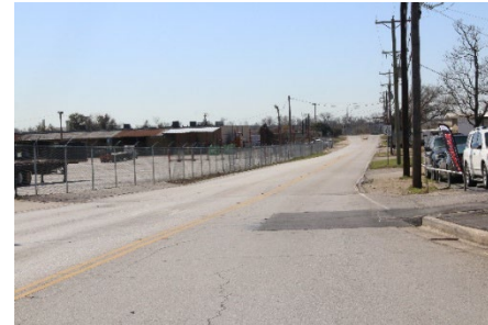
Limited right-of-way along Norwood Drive facing south.
