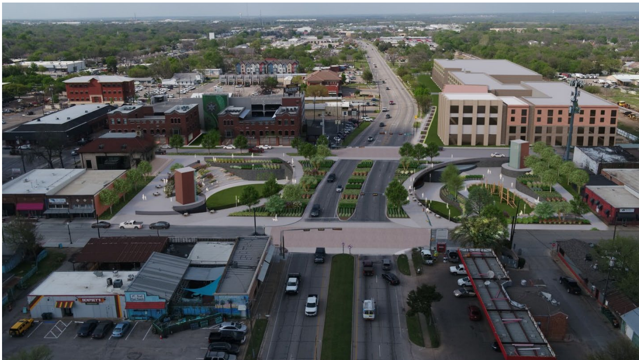
Highway 5 downtown pedestrian Connection Deck Park inverted deck park design.(City of McKinney)
