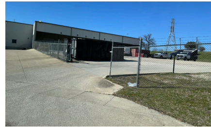
Many study area properties flanking the corridor are characterized by industrial buildings with large parking lots.
