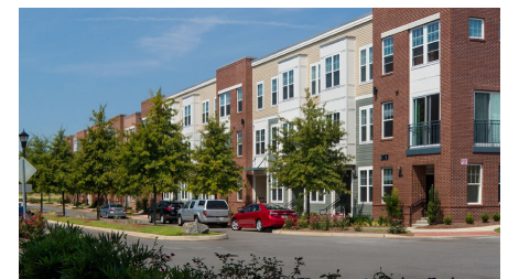
Multi-family apartments with ornamental trees and landscaping
