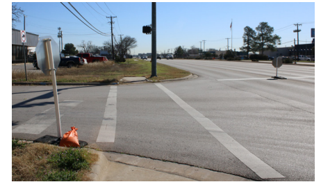
Intersection at Hurstview Drive highlighting lack of sidewalk connections.
