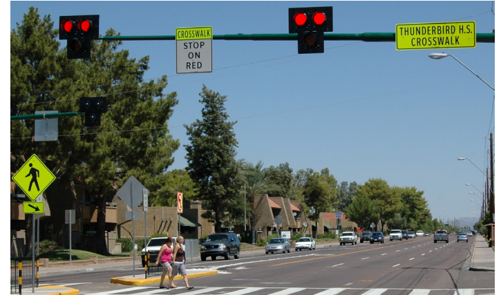
The HAWK beacon is a pedestrian crossing that uses a red light indication to stop vehicular traffic on an as-needed basis, allowing pedestrians more time to cross busy roadways away from a signalized intersection.
