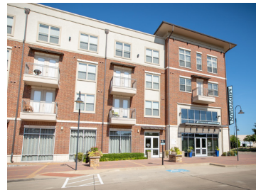
Vertical mixed-use multi-family apartments
