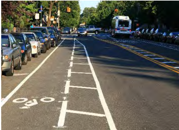
Shy zone on left - Brooklyn, NY Source: New York Department of Transportation
