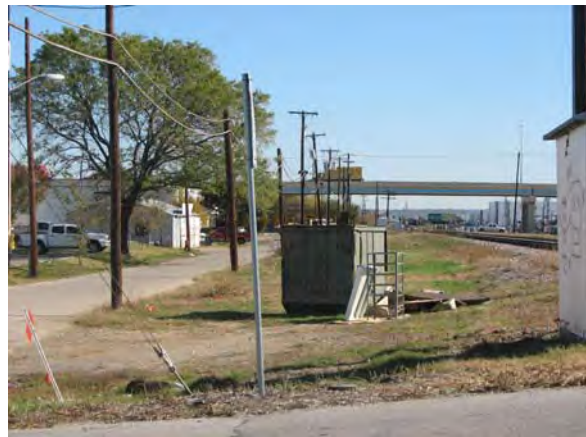
East 5 th Street at UP Mainline facing east Source: NCTCOG
