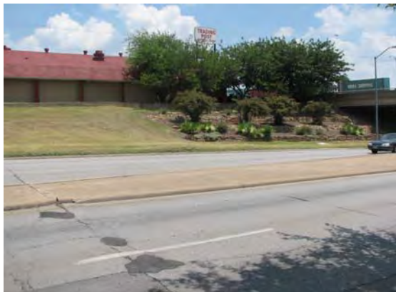
Carrier Parkway at Main Street overpass facing east Source: NCTCOG
