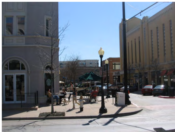
Bulb-out - McKinney, TX Source: NCTCOG
