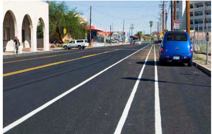
Shy zone on right - Tucson, AZ Source: Arizona Department of Transportation
