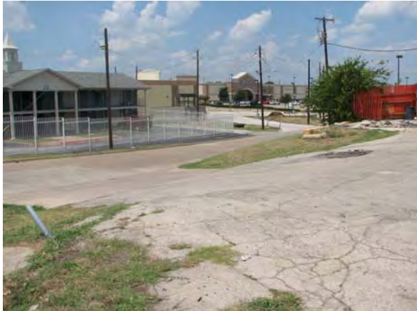
10 th Street at Main Street facing northwest Source: NCTCOG
