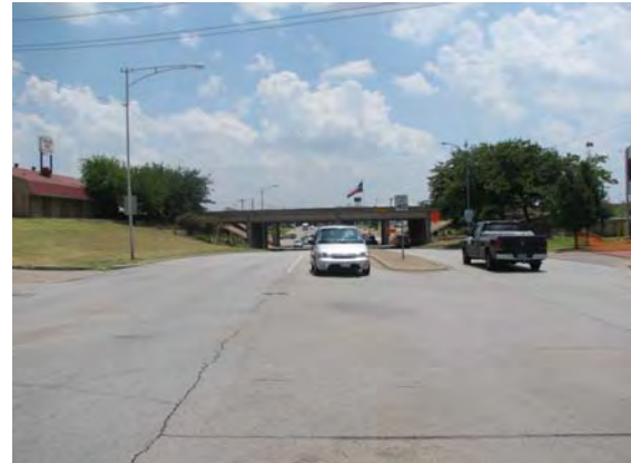
Carrier Parkway at Fort Worth Street facing south Source: NCTCOG
