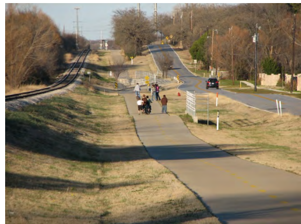
Shared Use Path - North Richland Hills, TX Source: NCTCOG
