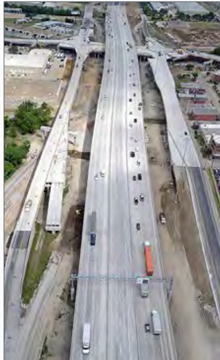
Above image: Belt Line Road interchange in Carrollton.
