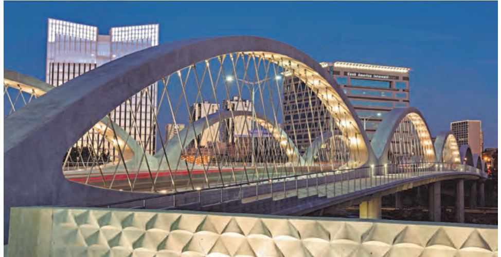
The world's first precast network arch bridge, the West 7th Street bridge was opened in 2013.
