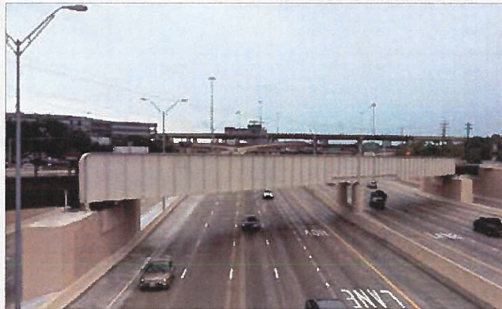
PHOTO 1: New railroad bridge at the US 75/PGBT interchange.
