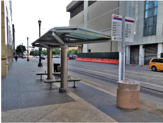
Bus Stop Shelter (Source: Houston, Texas)
