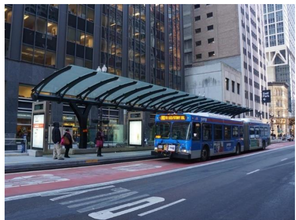
Designated Bus Lanes/High Quality Shelter (Source: CTA Loop Link Station)
