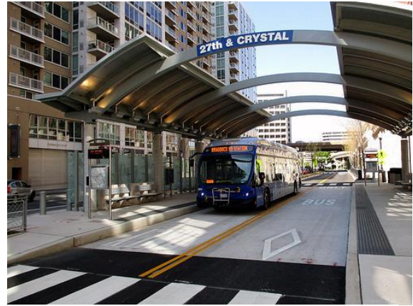
Metroway Station (Source: Arlington, Virginia)
