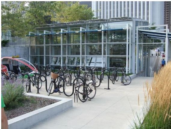
Millennium Park bicycle parking (Source: Chicago, IL)
