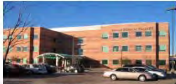
Medical Office Buildings
