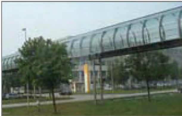
Over-Rail Pedestrian Access
