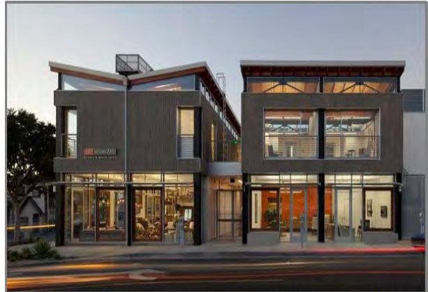
Loft Office R&D
