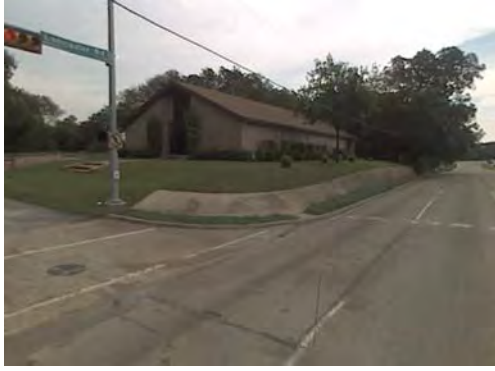
Sweet Fellowship Church located at 2106 Shellhorse Dr. The building and landscaping are in good condition. No sidewalks provided for entrance to the church.
