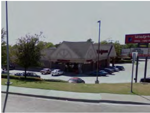
Walgreens located at 5101 S. Lancaster Rd. The building and landscape are in good condition. However, the entrance of the building is surrounded by parking making it difficult to walk to from the sidewalk.
