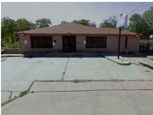
Wholesale Beauty Supply located at 3411 S. Lancaster Rd. The property contains a free-standing building with parking in the front.
