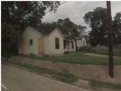
Single-family located at 2103 Arden Rd. This residence is in need of repairs as indicated by the wooden boards over several sections of the house.
