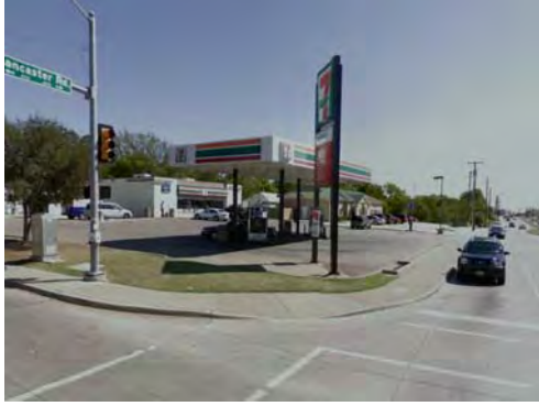
7 Eleven located at 3602 S. Lancaster Rd. The property contains a gasoline station with a convenience store.
