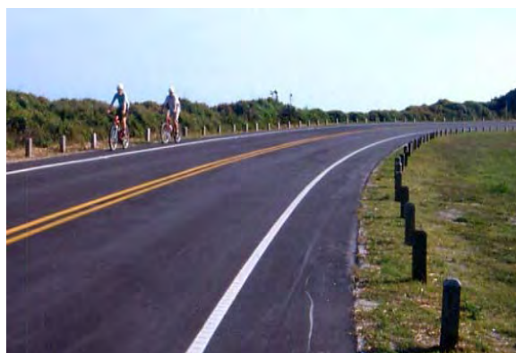
Exhibit B-14: Paved Shoulder Source: Federal Highway Administration
