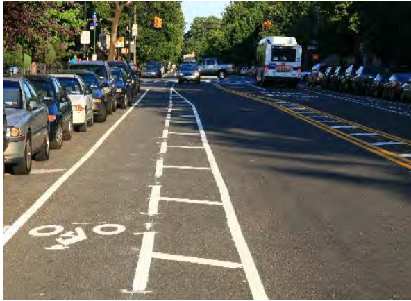
Exhibit B-8: Shy zone on left Source: New York DOT
