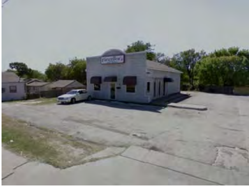
Flewellen's Hair Salon located at 3611 S. Lancaster Rd. The property contains a free-standing building surrounded with parking.
