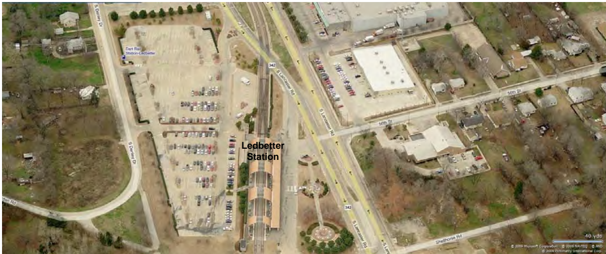
This image shows the overview of the Ledbetter Station and some existing development.
