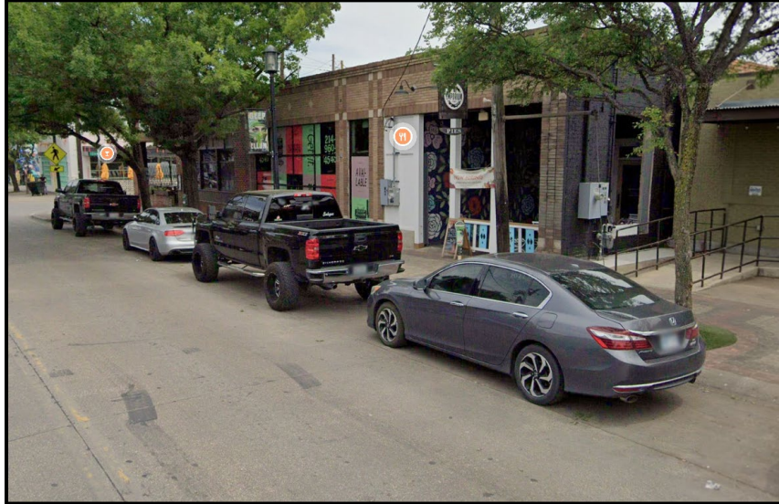
Figure 8: Main Street Missing On-Street Parking Space Delineation
