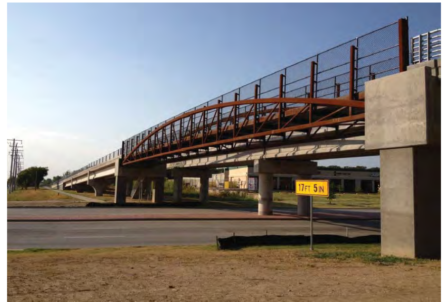
Photo Courtesy City of Denton: MLK Trail Bridge at Loop 288 constructed adjacent to the DCTA Rail Bridge
