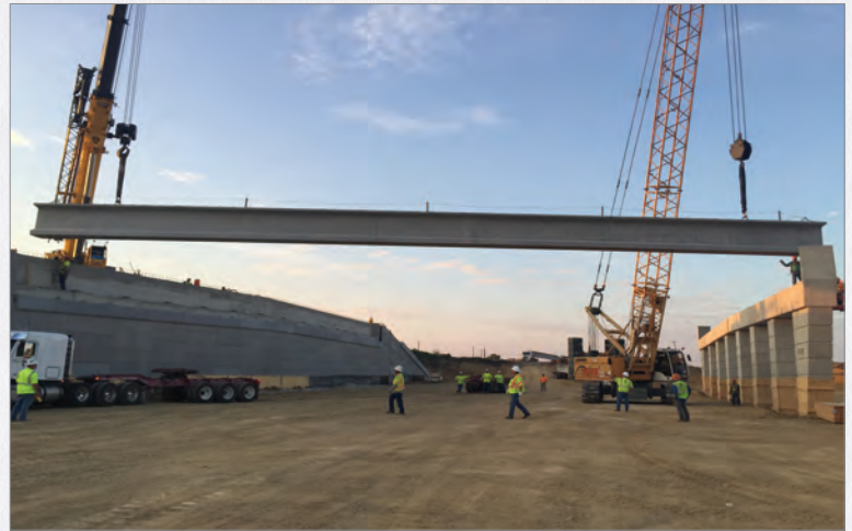
September 2016 - Construction on Webb Lynn Road bridge at SH 360
