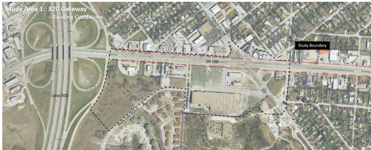
Figure 23. IH 820 Gateway: Existing Conditions
