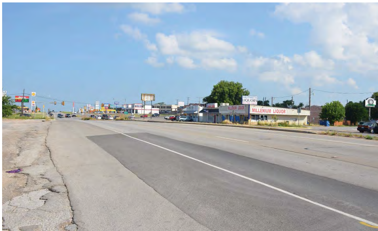
Figure 1. Continuous Driveways Along SH 199 East of Roberts Cut Off Road
