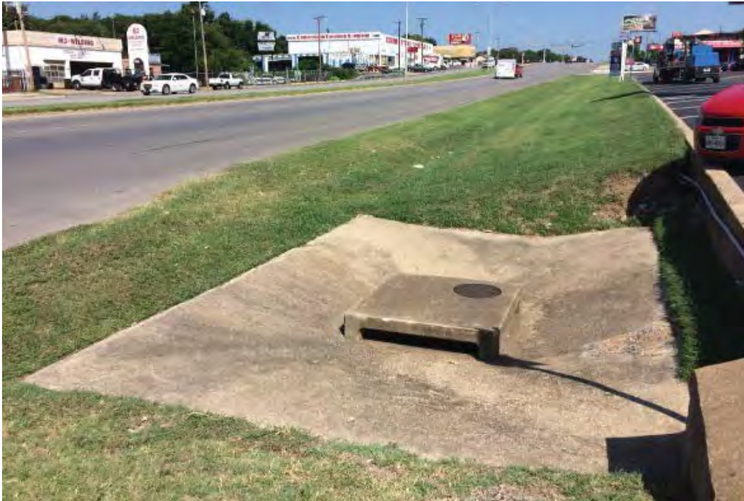
Figure 1. Area with Road Side Ditches and Inlet at Low Point (SH 199, Fort Worth) Source: Freese and Nichols, Inc., 2016
