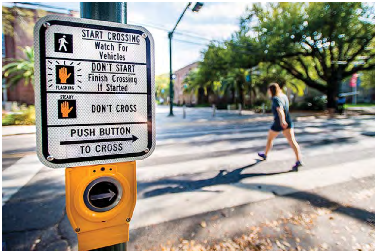
Figure 15. Accessible Pedestrian Signal Pushbutton Assembly
