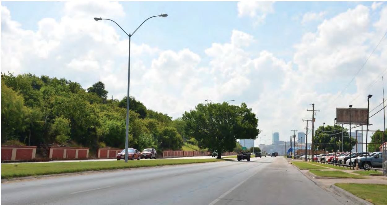
Figure 2. Median Tree and Lighting East of SH 199 and 18th Street Intersection
