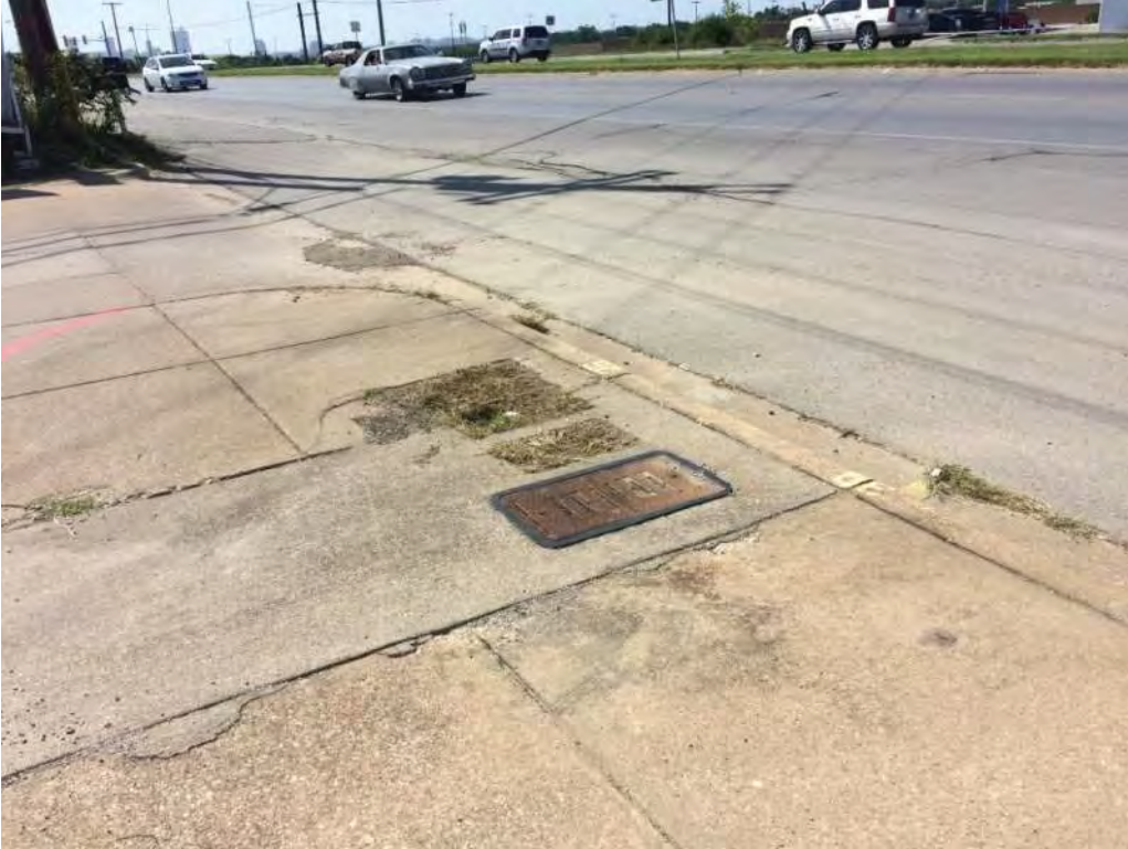
Jacksboro Highway with Curb and Gutter in Fort Worth near Ephriham Avenue
