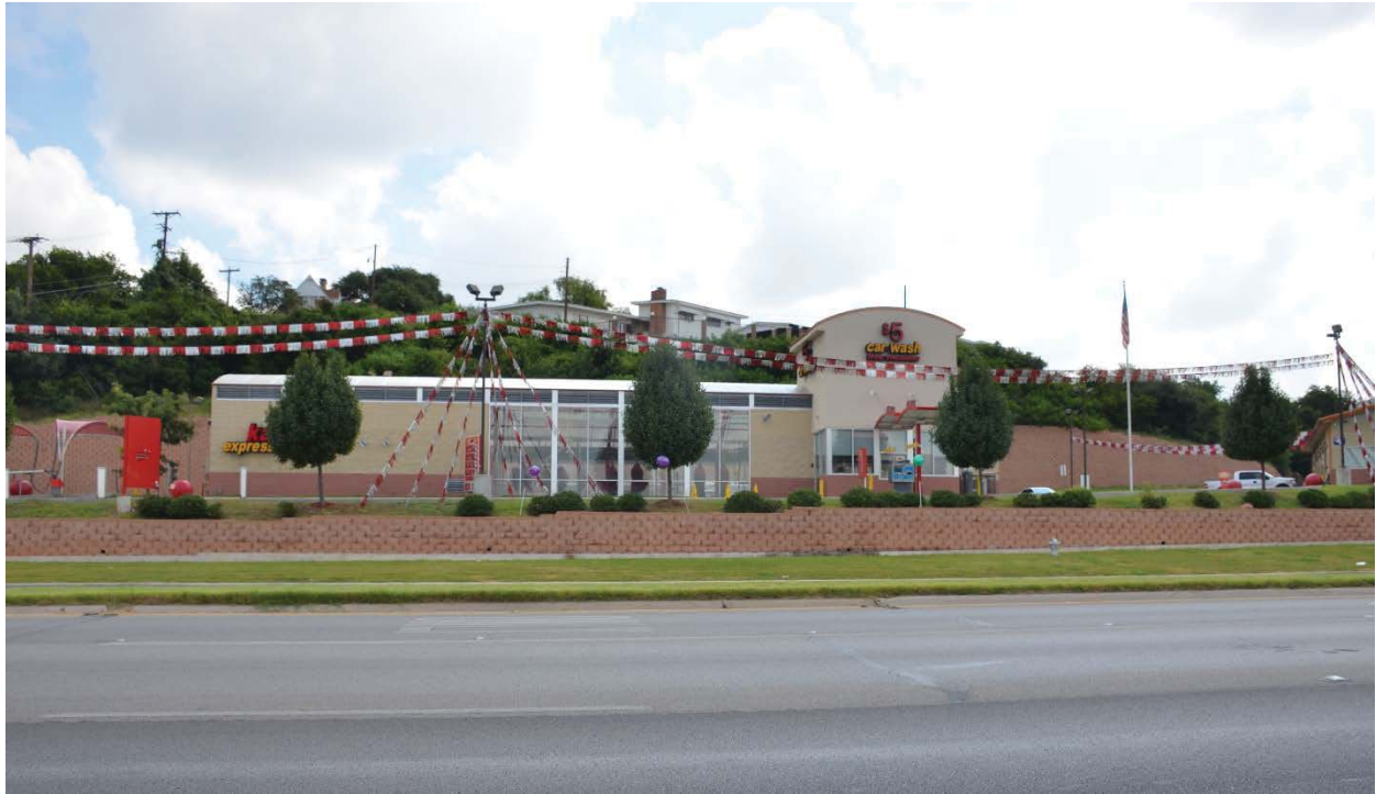
Figure 8. Recently Constructed Commercial Development Near SH 199 and 21st Street Intersection
