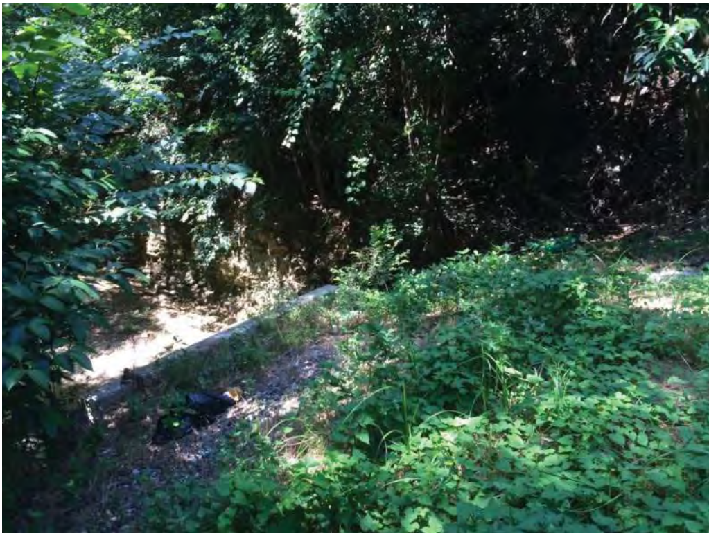
Culvert Outfall at Circle Ridge Drive
