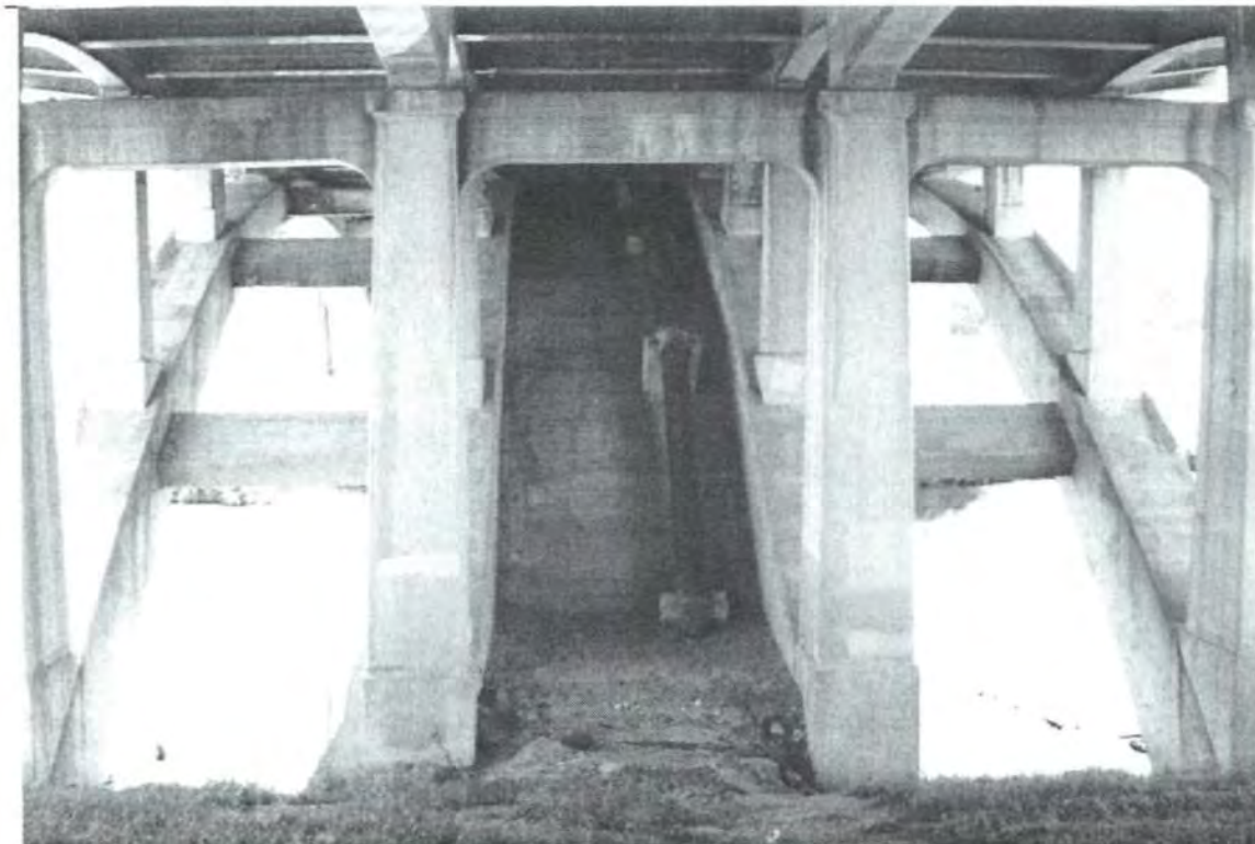
Figure 8: Conduit slab between the ribs of the arch, looking south
