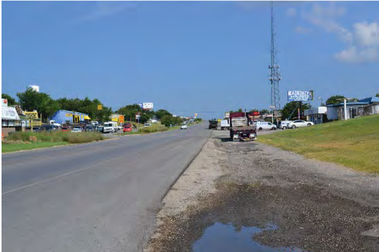
Figure 5. Typical Character Zone 2 Commercial Frontage
