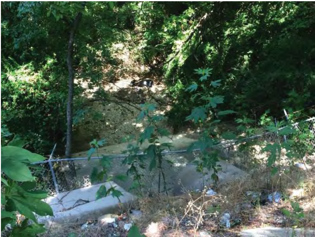
Culvert Outfall at Belle Avenue
