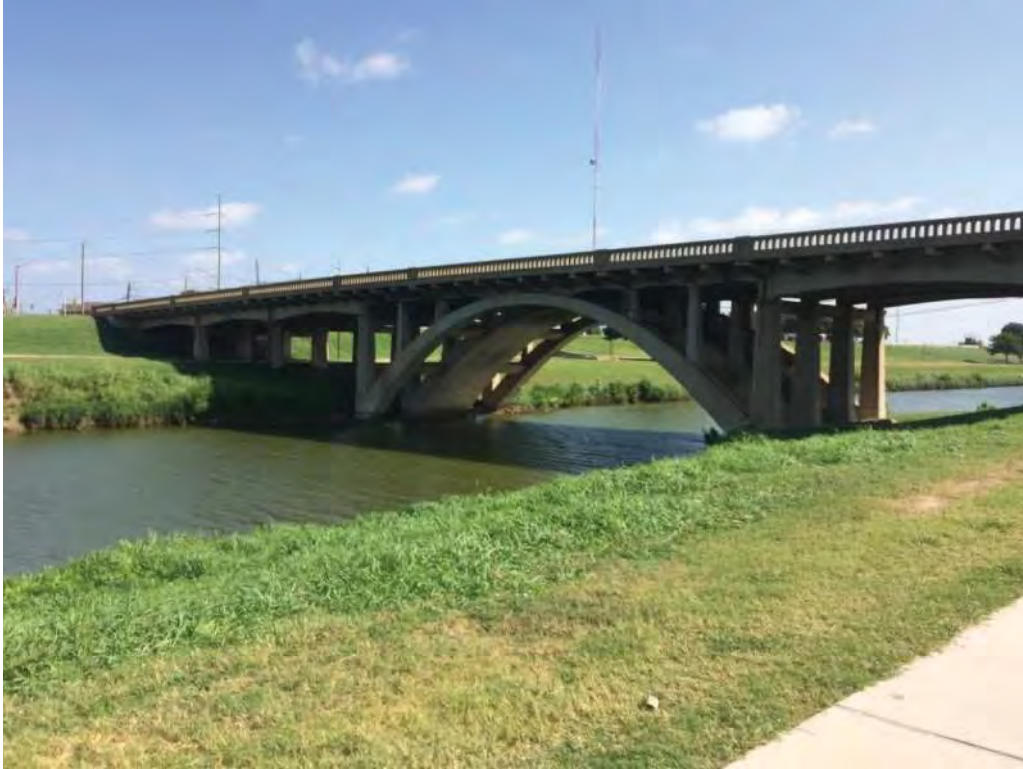
Henderson Street Bridge over the Clear Fork Trinity River
