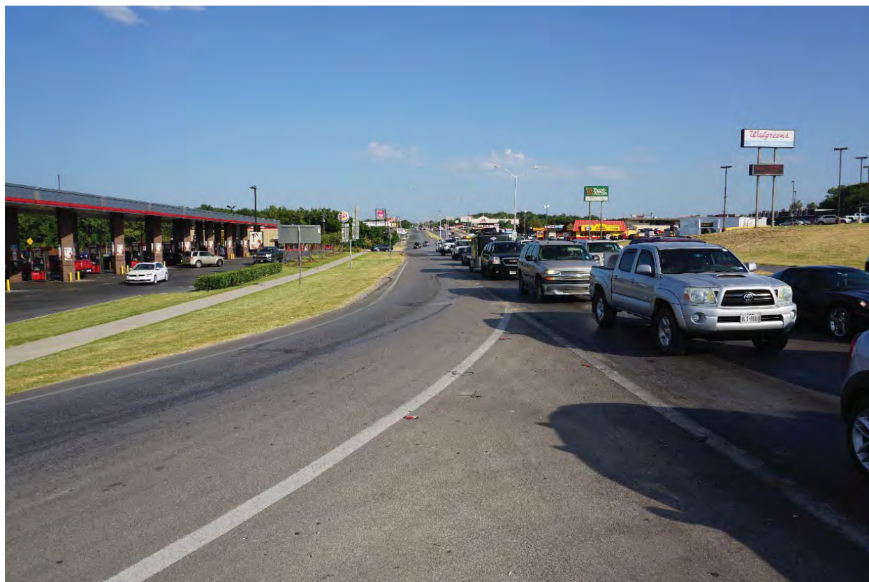
Figure 6. Typical Character Zone 3 Commercial Frontage West of SH 199 and SH 183 Intersection
