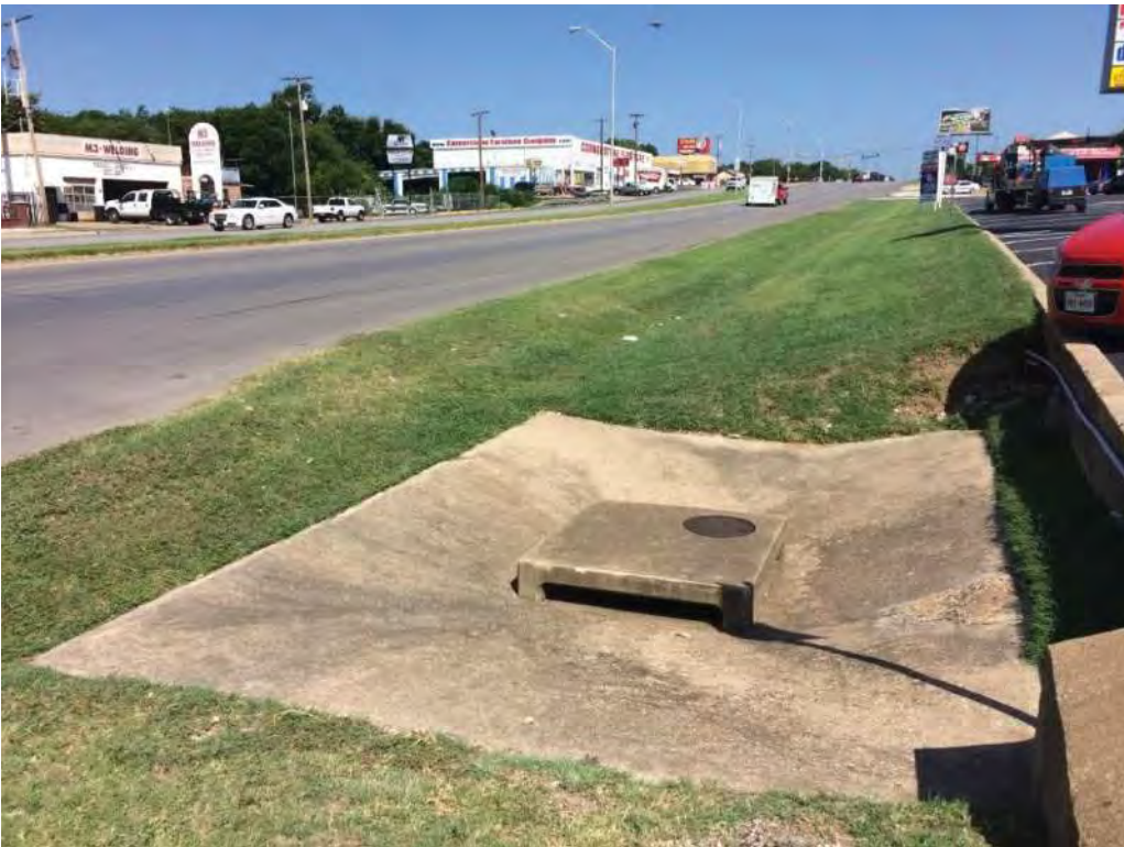
Inlet and Ditch at Jacksboro Highway in Fort Worth; No Curb and Gutter
