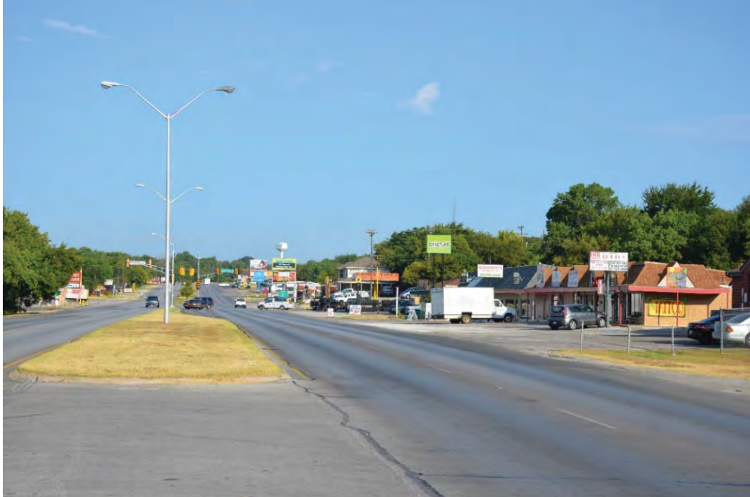
Figure 4. Median Opening and Left Turn Lane West of SH 199 and Beverly Hills Drive Intersection
