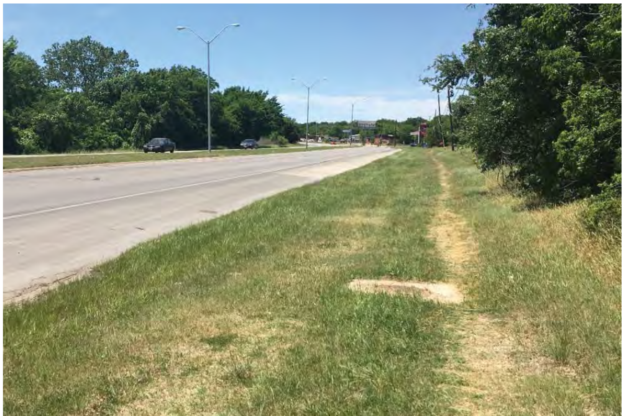
Figure 3. Pedestrian-Created Path along SH 199 West of Capri Drive Intersection Source: Freese and Nichols, Inc., 2016
