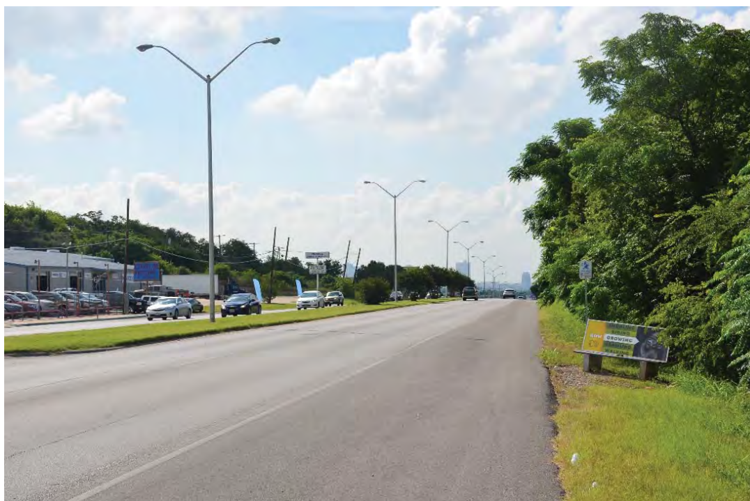
Figure 8. FWTA Bus Transit Stop East of SH 199 and Capri Drive Intersection
