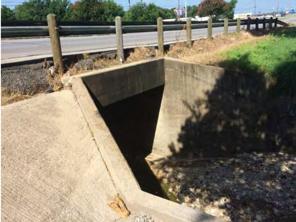
Culvert at Jacksboro Highway near Belle Avenue; No Curb and Gutter
