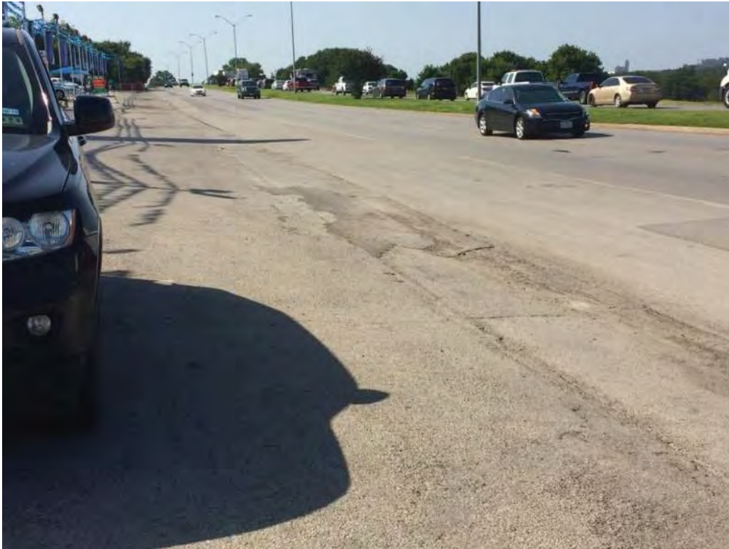
Jacksboro Highway Without Curb and Gutter near 21 st Street
