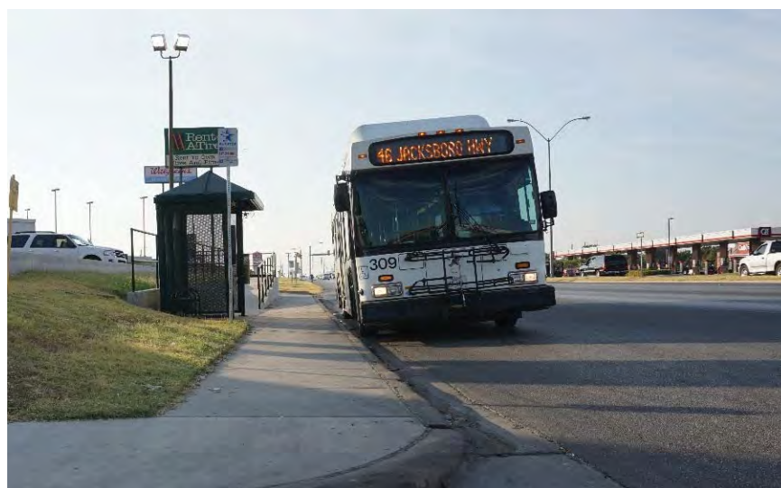
Figure 3. Existing Bus Shelter and Pull Out West of SH 199 and SH 183 Intersection at Town and Country Center
