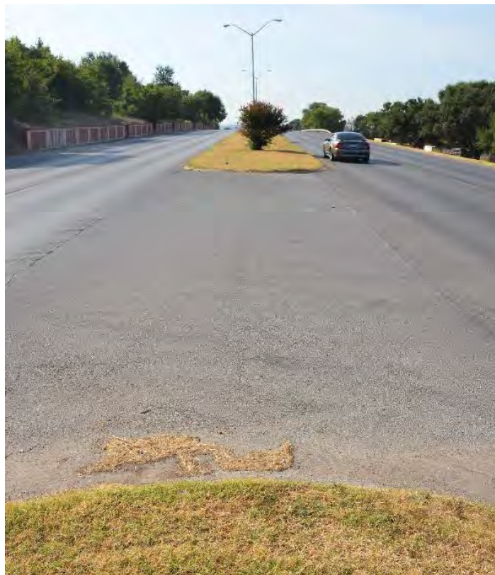
Figure 5. Center Median Opening East of SH 199 and 21 st Street Intersection
