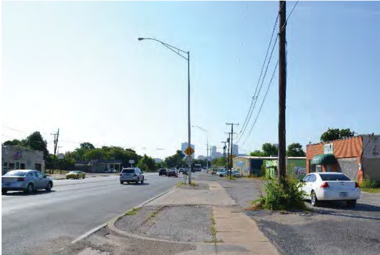
Figure 10. Typical Zone 4 Commercial Frontage Near SH 199 and University Drive Intersection
