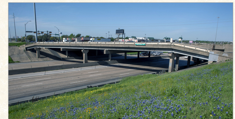
Looking west at the Skillman Street bridge over I-635.
