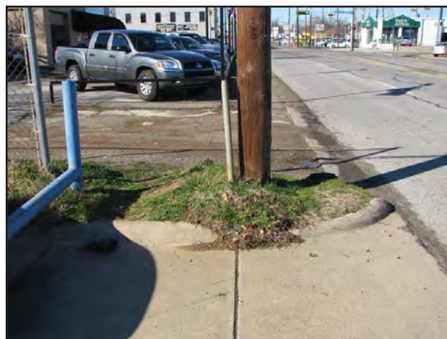
The Corridor's right-of-ways have disconnected sidewalks, aging curbs and drives, and numerous utility poles which cause pedestrian conflicts with the poles and traffic.
