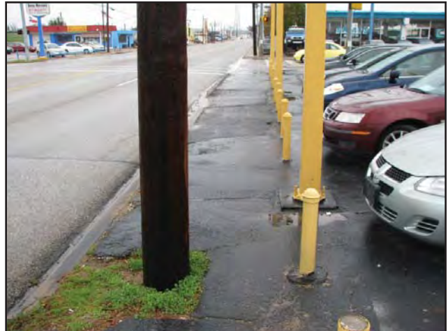
Utility poles affect pedestrian safety and narrow right-of-ways limit preferred solutions.
